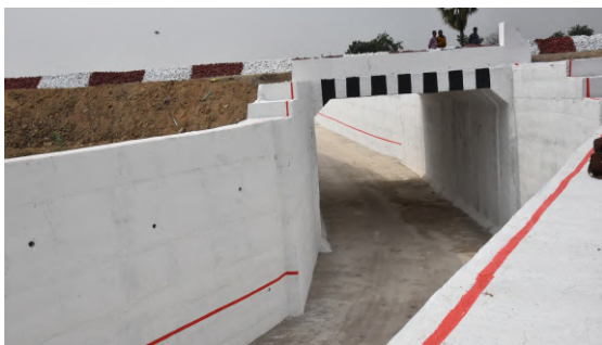
UMLC converted to Limited Height Subway
