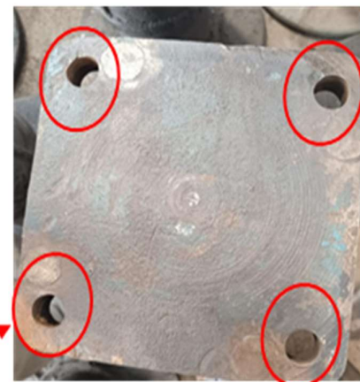
Riveting of Buffer base plate with casing.
