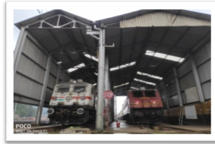
Pic: Freight Loco Trip shed (FTS)
