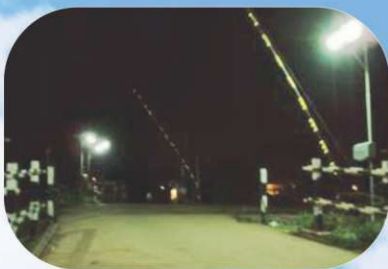
Solar Power Light 161 Nos. (Total 12.8 KW)
