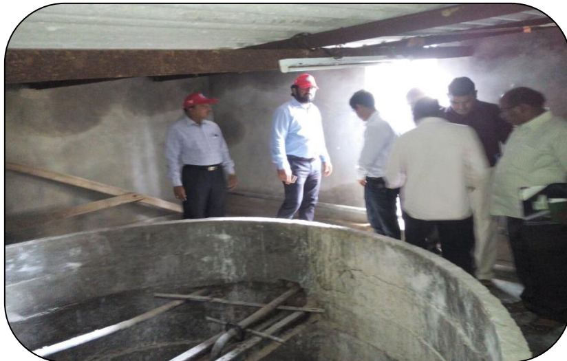
Inspection by DY. CE/Br. Lines /SC, and Sr DEn /C/BZA at CHIRALA
