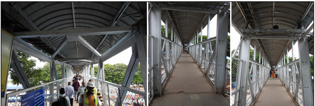
Fig 6: Roof truss and roof elements of three spans
