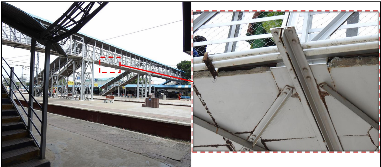
Fig 2: Pipeline – Utilities are observed along the span
