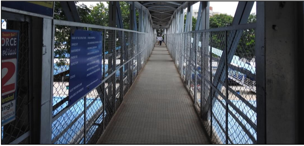
Fig 4 Flooring and protective screen
