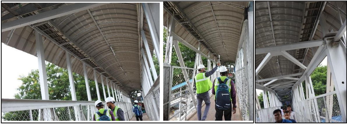
Fig 1: Cables and Roof truss
