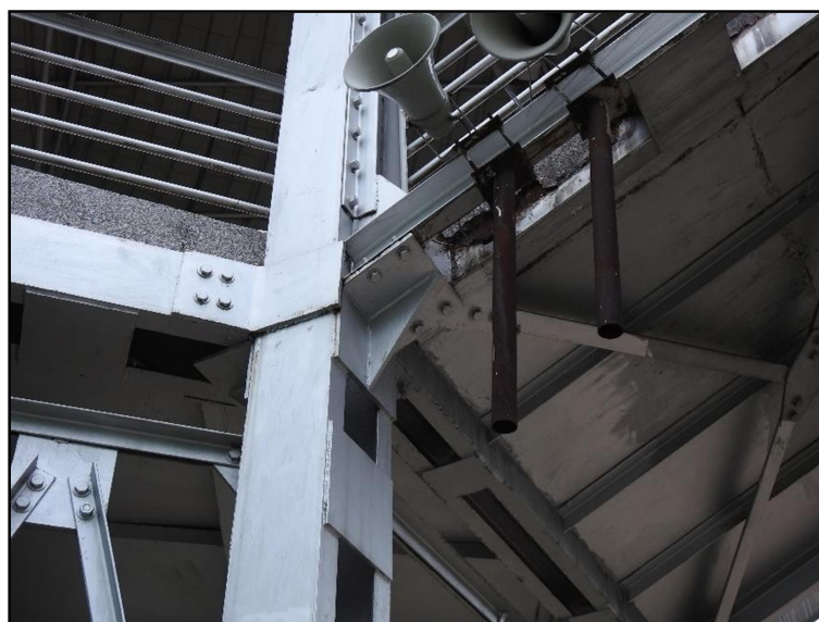
Fig 6: Cleat angle
