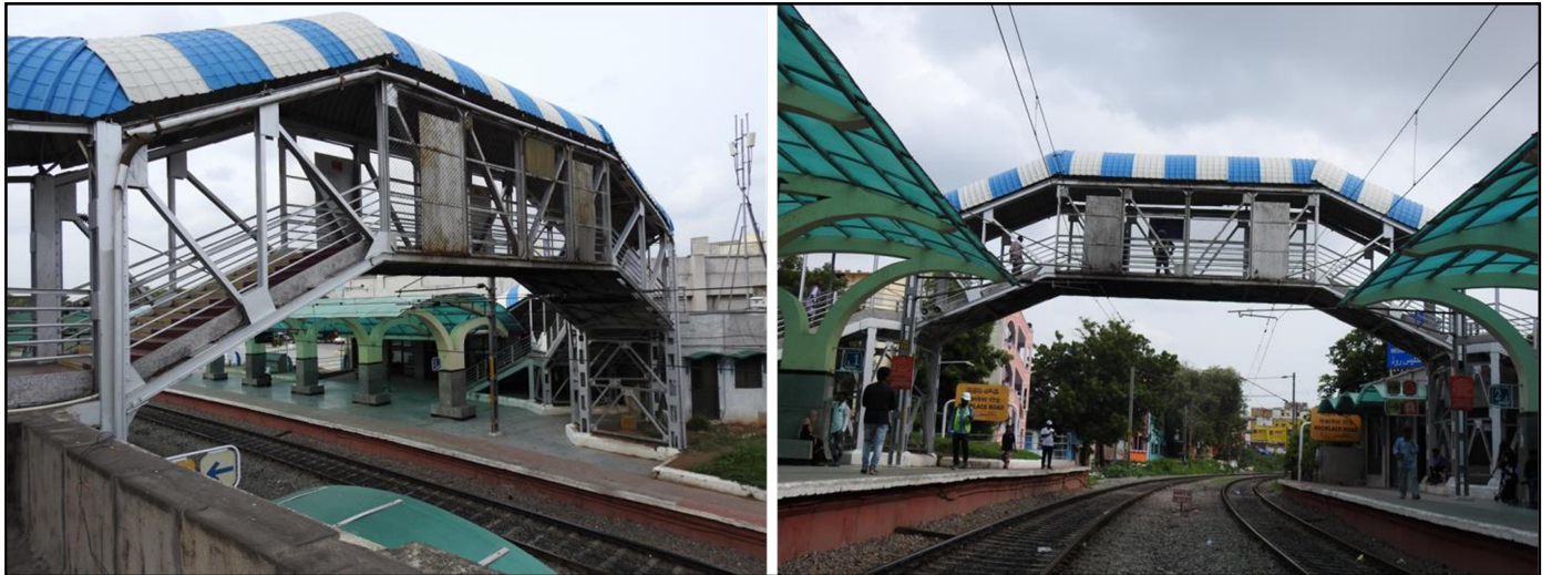
Fig 5: FOB Truss view
