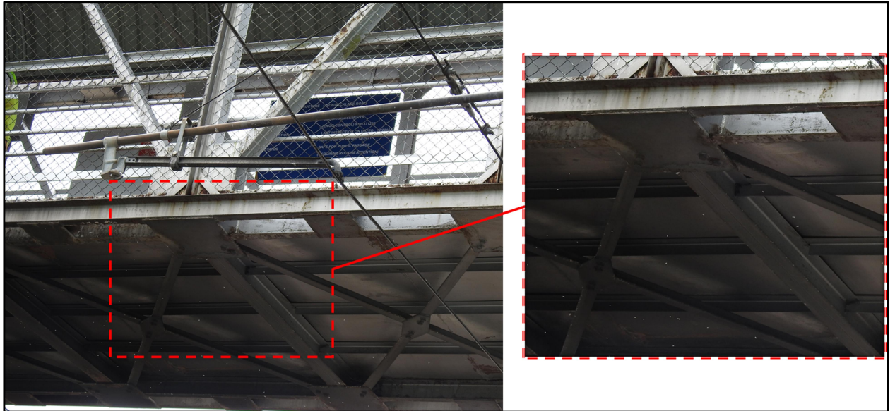
Fig 4: Tie members and secondary girders with bracings
