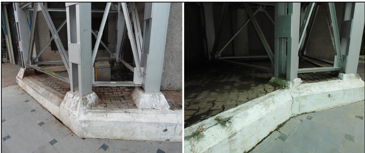
Fig 3: Trestles and their protection with concrete encasement
