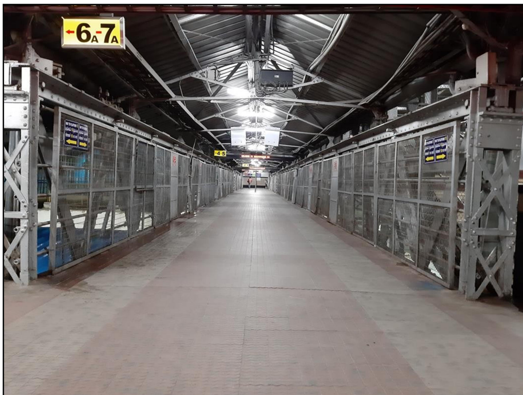
Fig 3: Protective screen provided on both sides and details of Flooring
