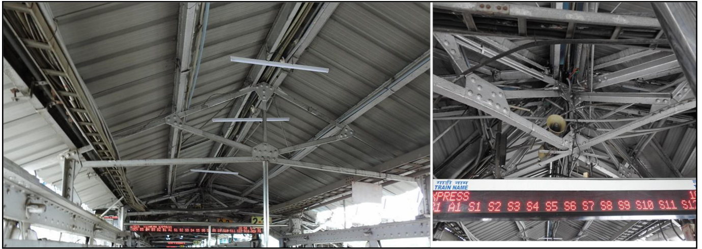
Fig 1: Electrical Cables, Roof truss and Roof sheet
