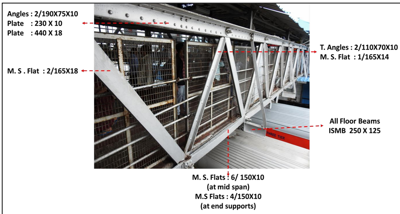
Fig 4: Section properties of Truss
