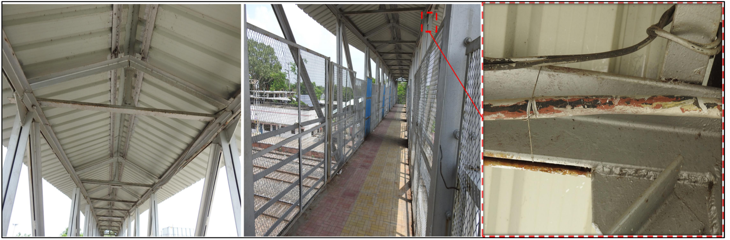
Fig 1: Cables, Roof truss, Flooring and Protective screen
