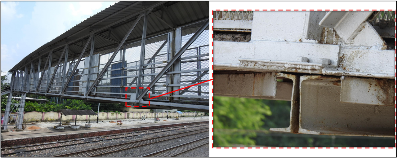
Fig 3: Top and bottom chord members, bracings and Floor beams
