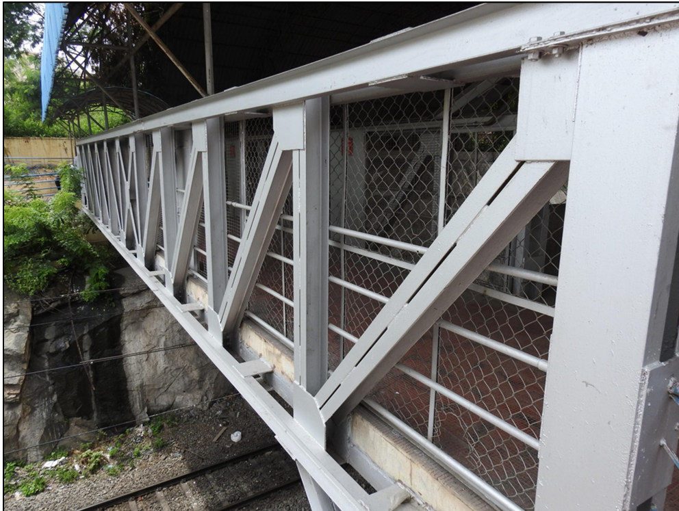
Fig 4: Top and bottom main chord members with vertical and diagonal bracings
