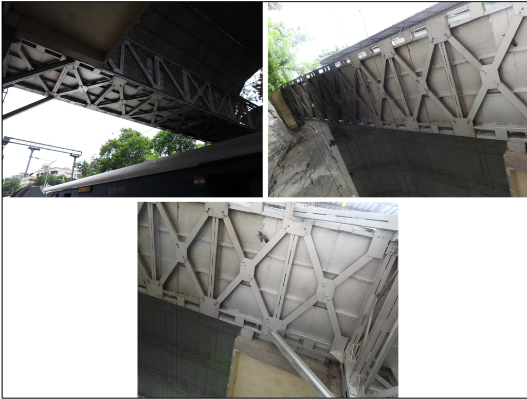
Fig 5: Slab is supported with sacrificial plate
