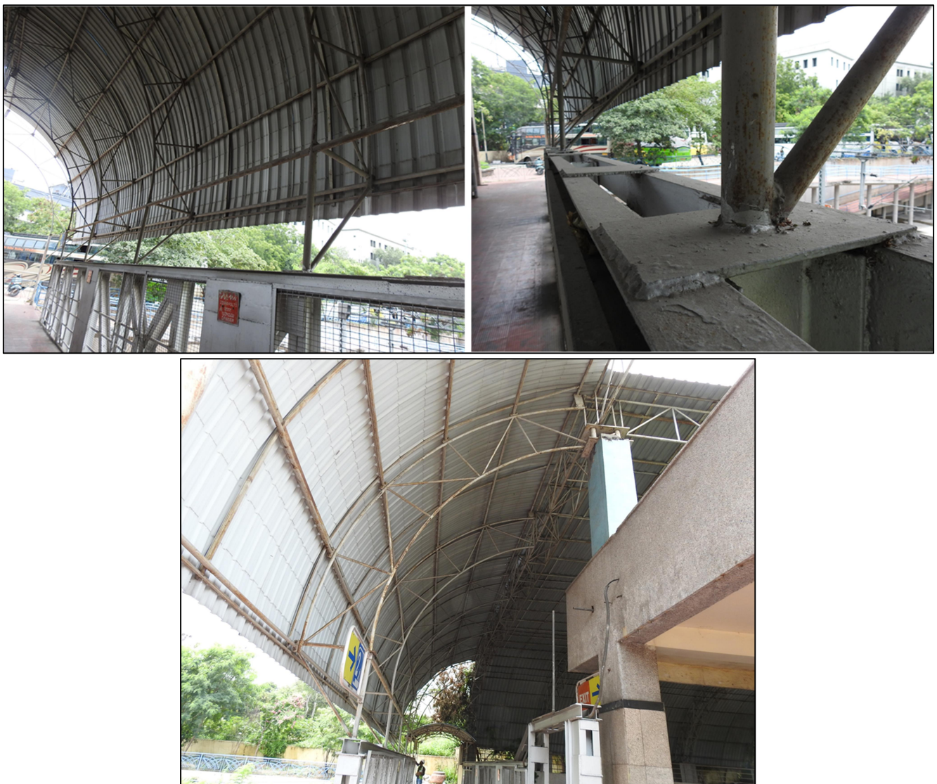
Fig 2: Roof Sheet and Roof truss
