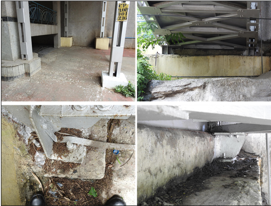
Fig 3: Trestles and their protection with concrete encasement
