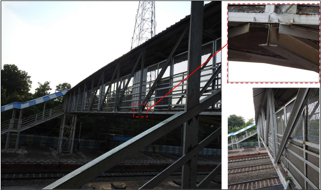
Fig 3: Top and bottom chord members, bracings and Floor beams
