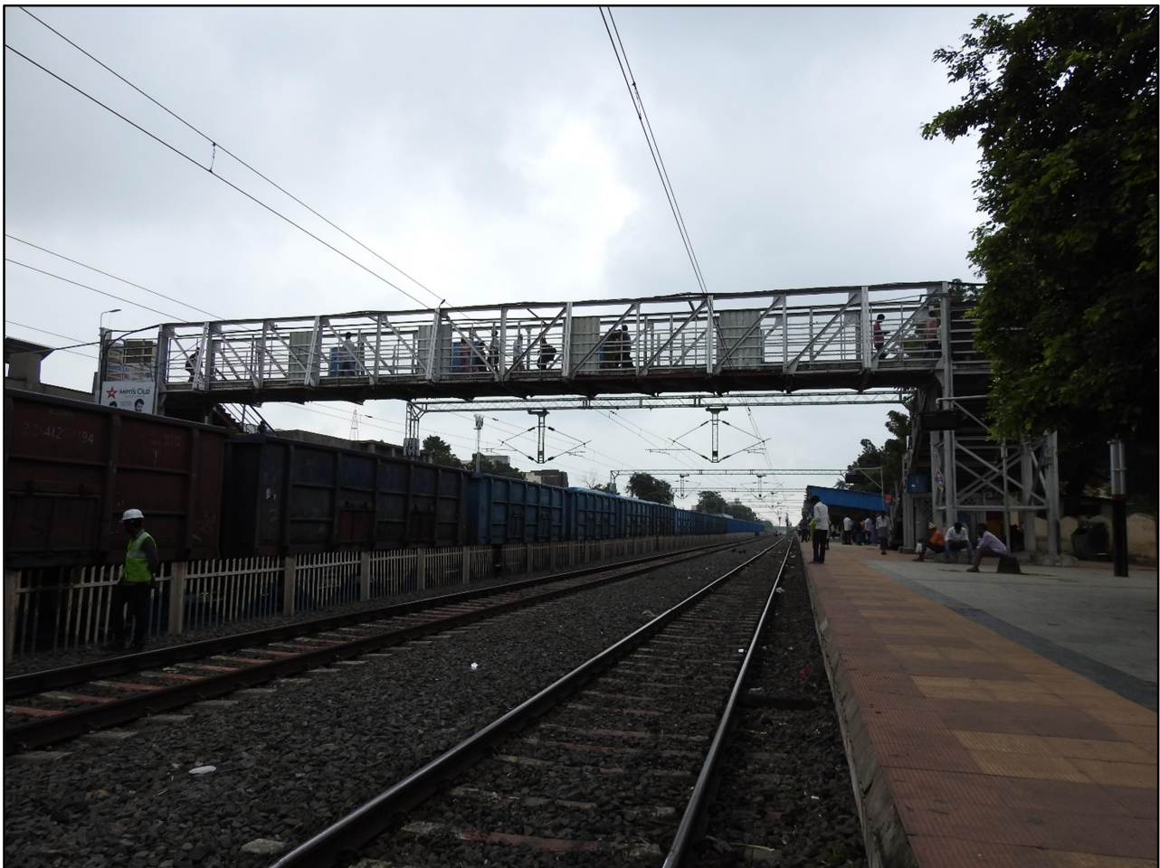
Fig 1: Front view of FOB towards Khammam
