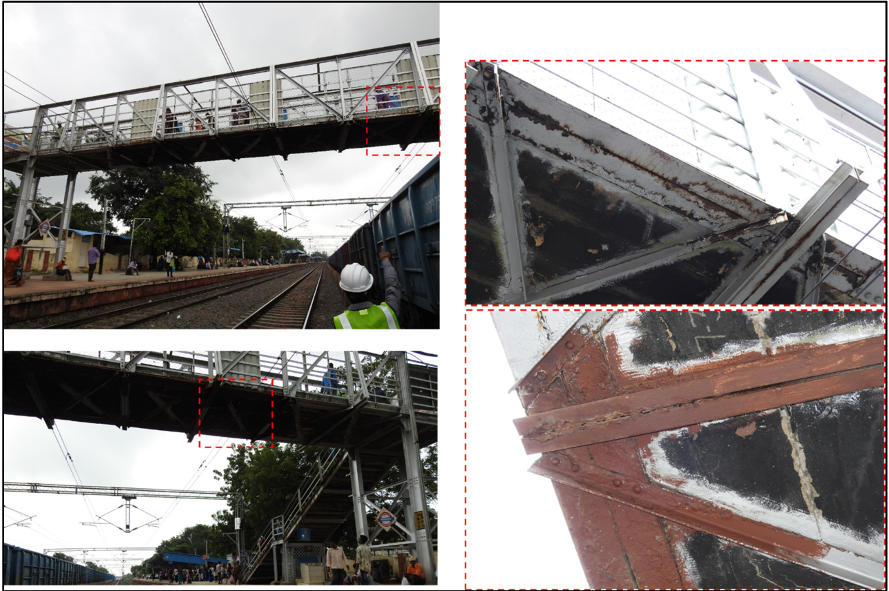
Fig 6: Redoxide paint applied at corroded joints and member
