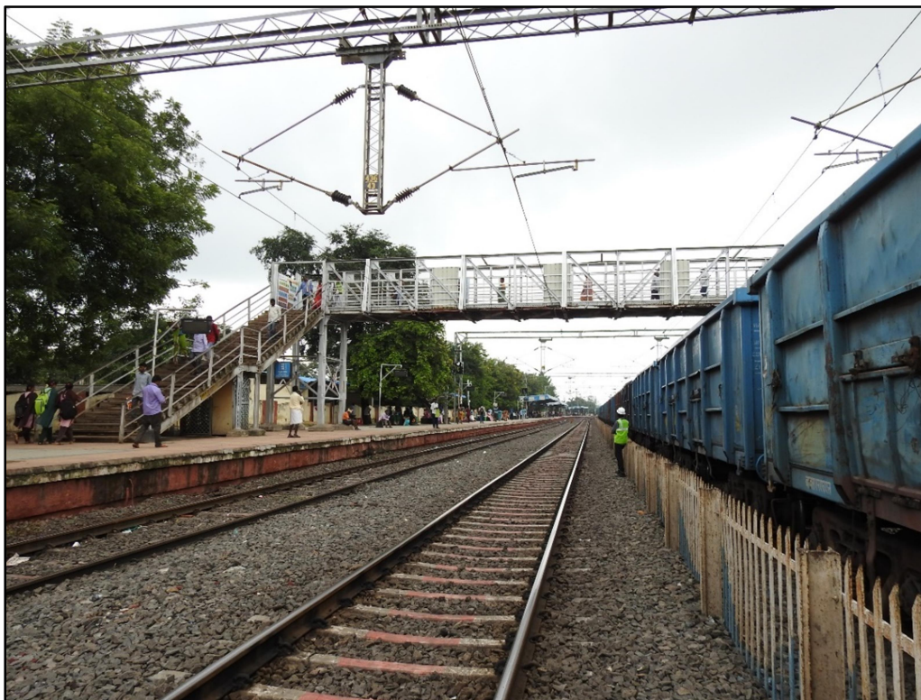
Fig 5: FOB view from platform 2 with staircase
