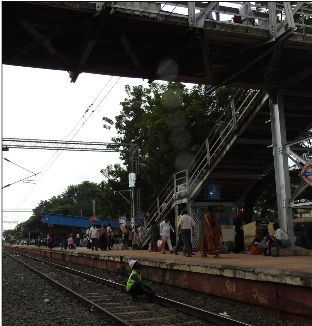
Fig 4: Measuring Vertical Clearance using laser meter (from rail top to girder bottom)
