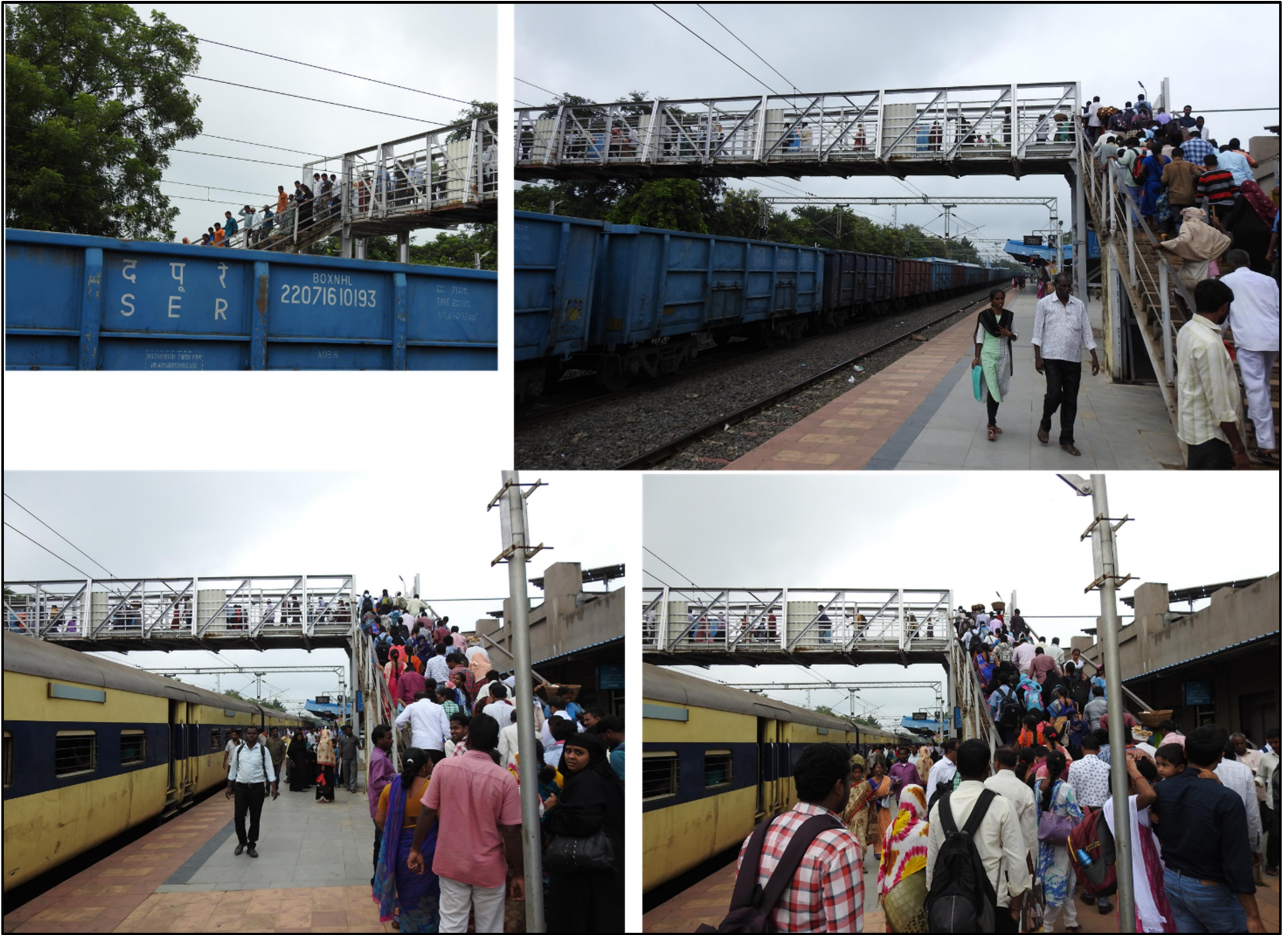
Fig 2: FOB under live load
