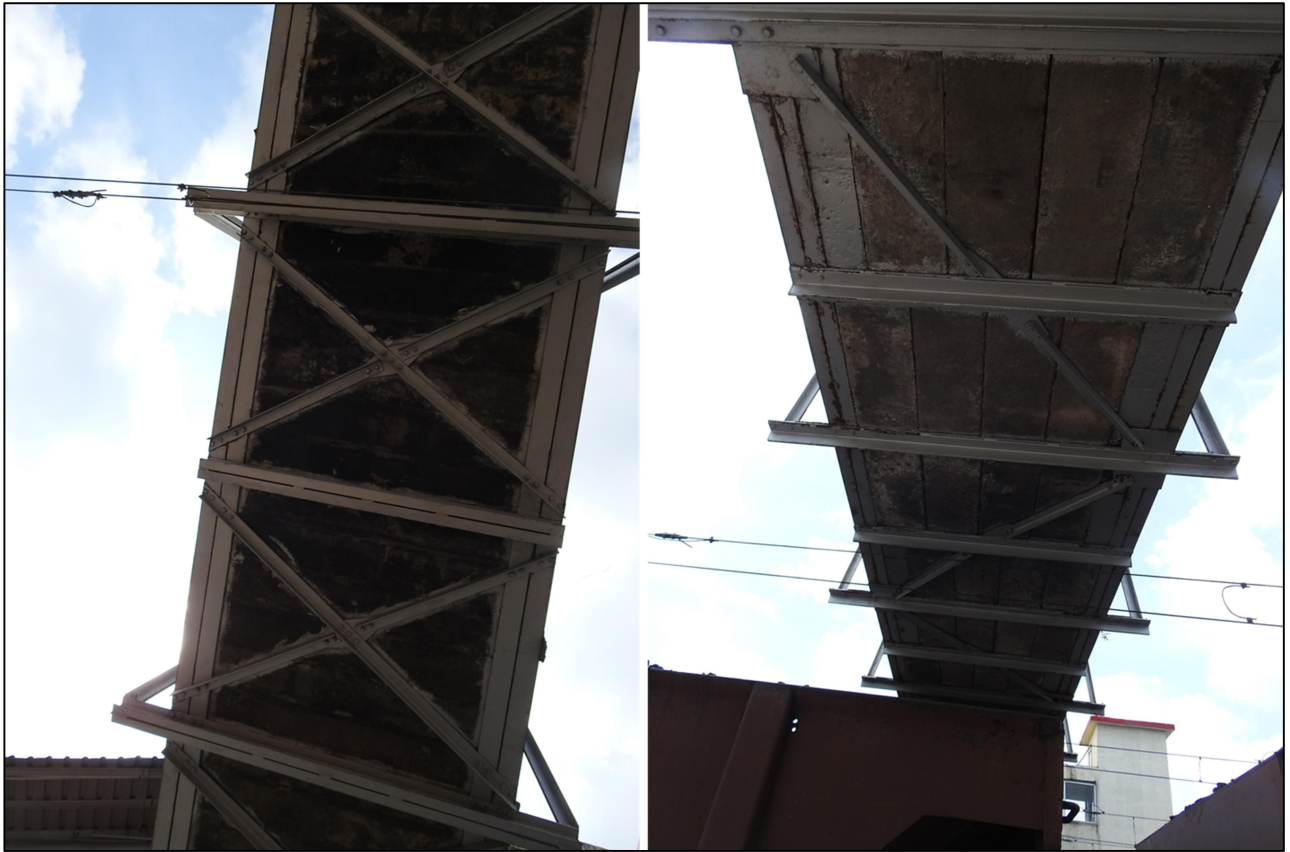
Fig 5: Bottom view of 1 st and 2 nd span of FOB
