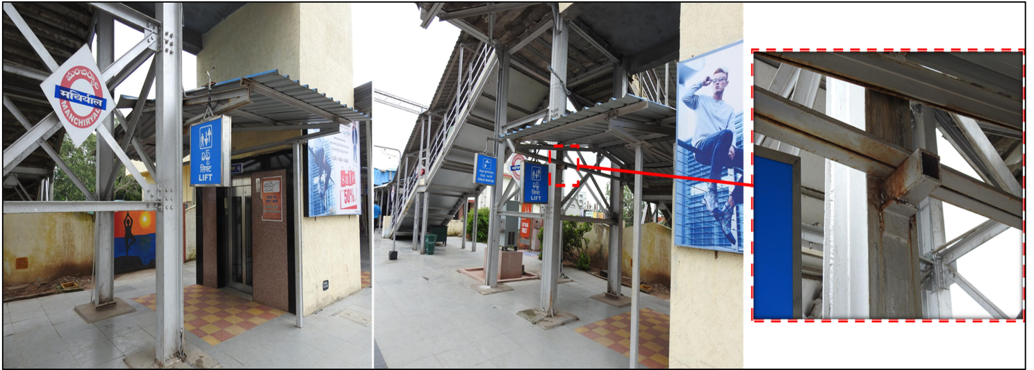
Fig 3: Elevator Roof truss supported on trestles on PF-1 and PF-2 & RCC slab resting on trestles
