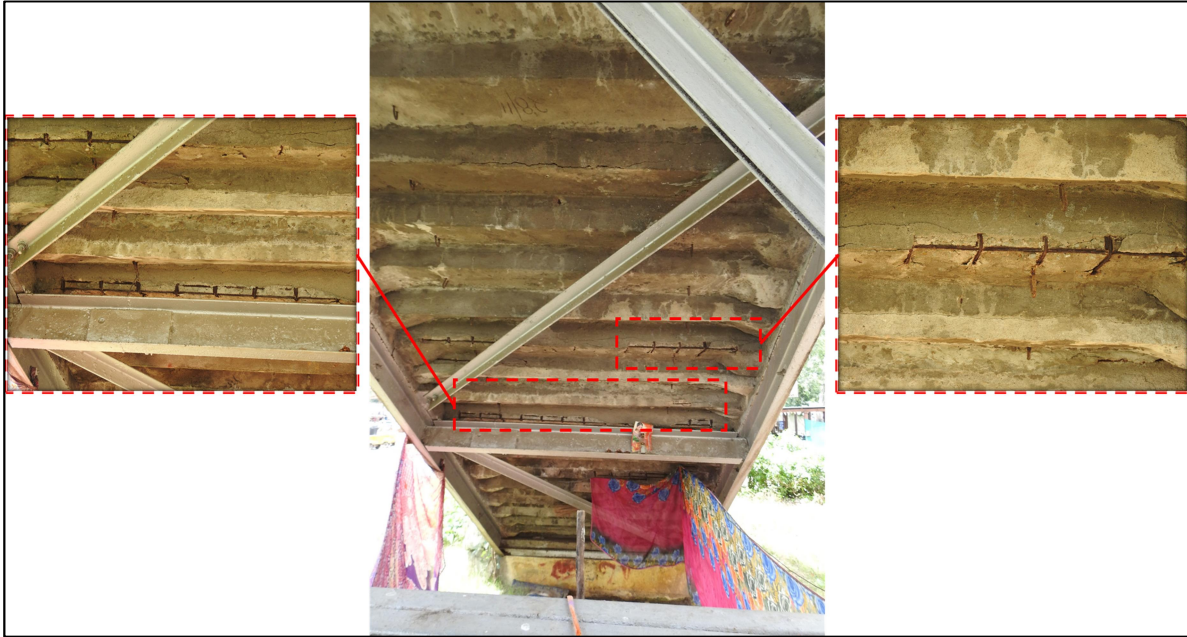
Reinforcement exposed slab panels
