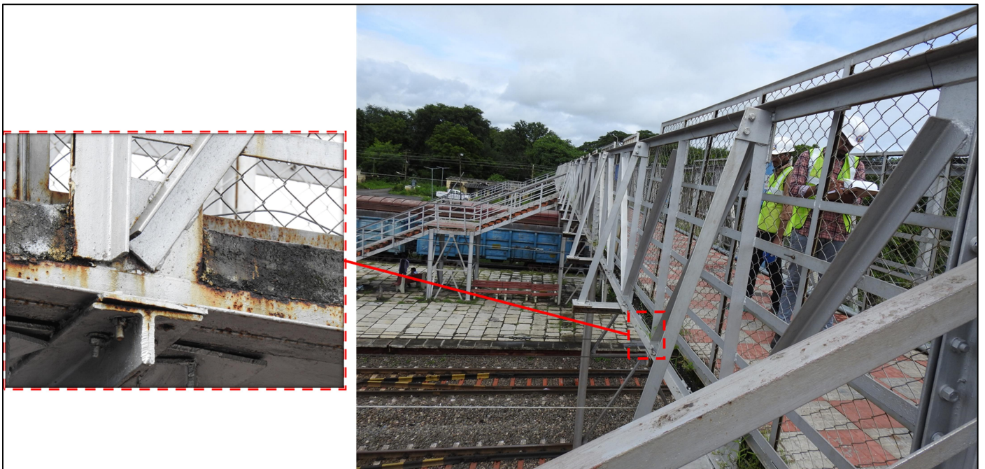
Fig 3: Chord members, Floor beams, vertical and diagonal bracings
