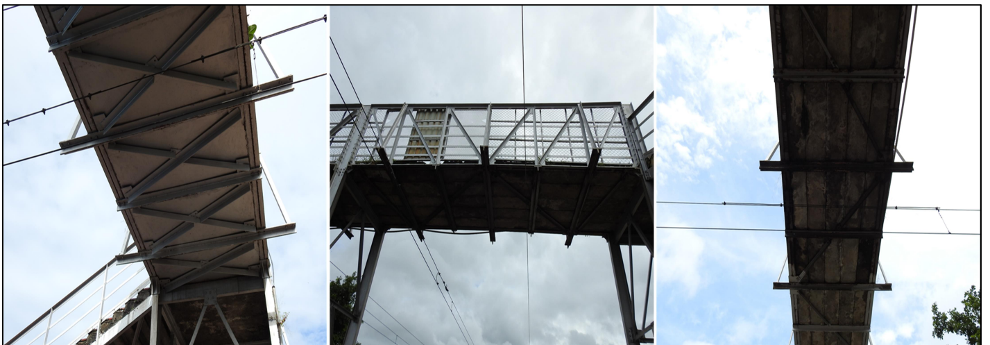
Fig 3: Chord members, Floor beams, vertical and diagonal bracings
