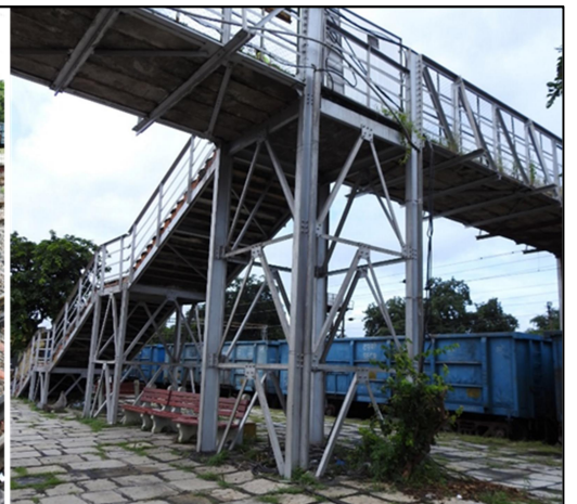
(f) Platform-4 staircase landing
