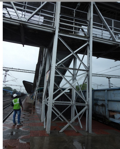
(b) Platform-2 staircase landing
