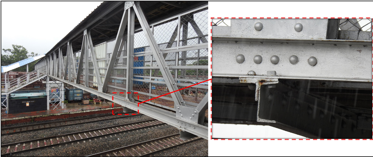
Fig 3: Chord members, verticals, diagonal bracings and Floor beams
