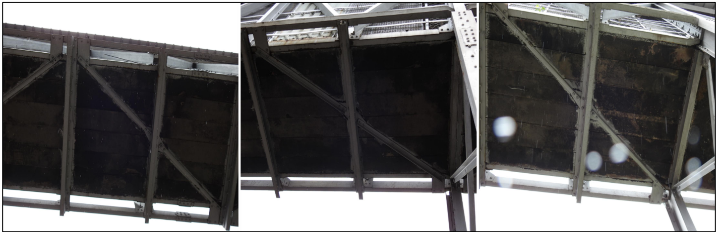
Fig 4: Bottom view Slab panels
