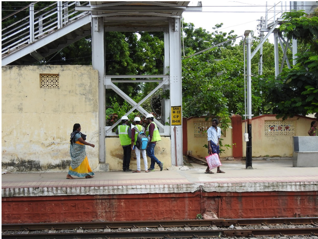
Fig 5: FOB is supported on four column Trestles on either side
