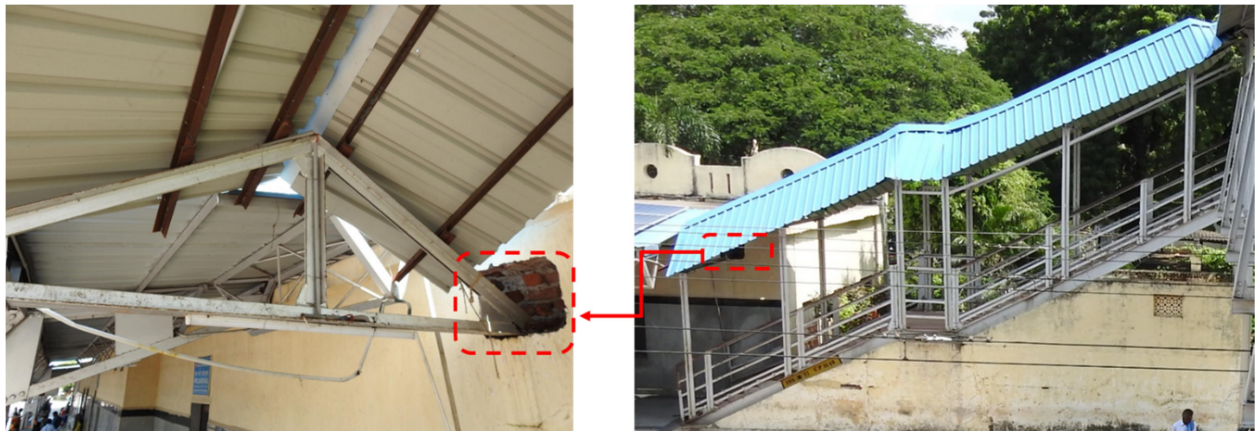
Fig 2: Staircase Roof truss on platform 1
