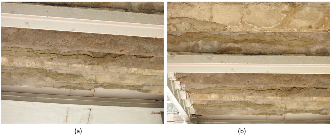
Fig 8: Cracks are observed in staircase steps
