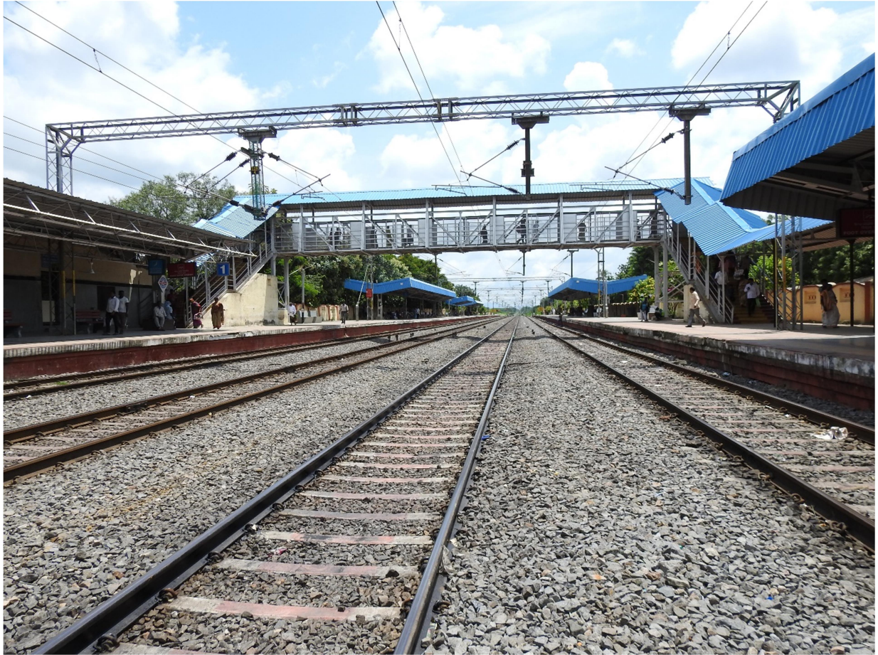
Fig 1: Front view of FOB towards Vijayawada Junction
