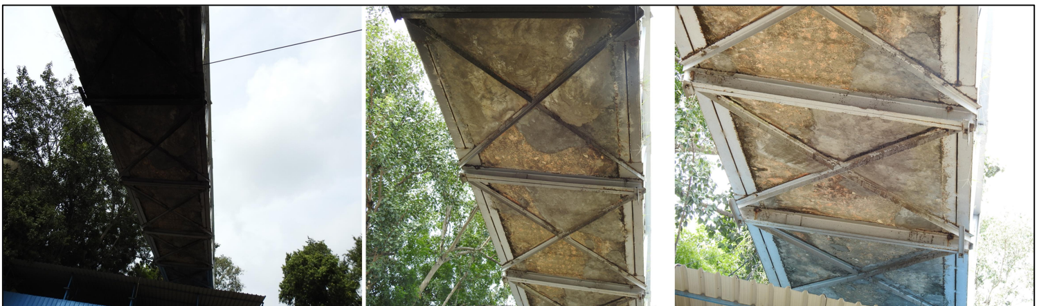
Fig 4: Bottom view Slab and Repair work
