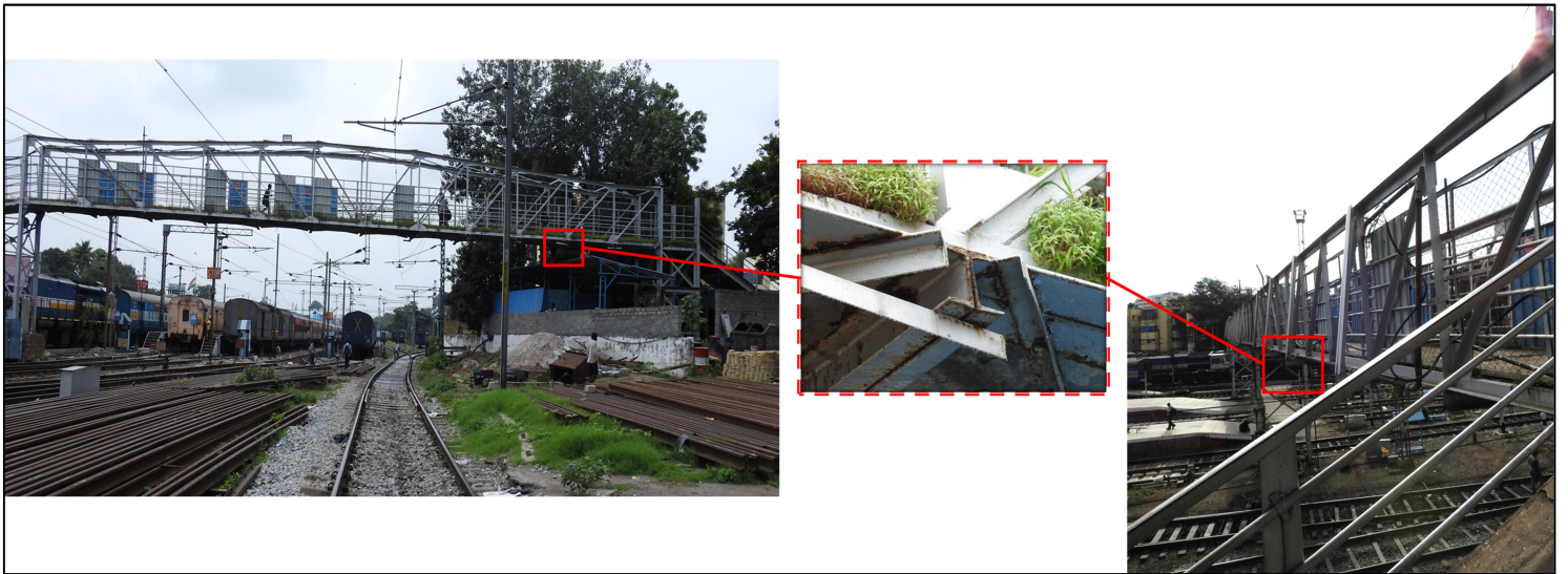
Fig 3: Chord members, Floor beams, vertical and diagonal bracings
