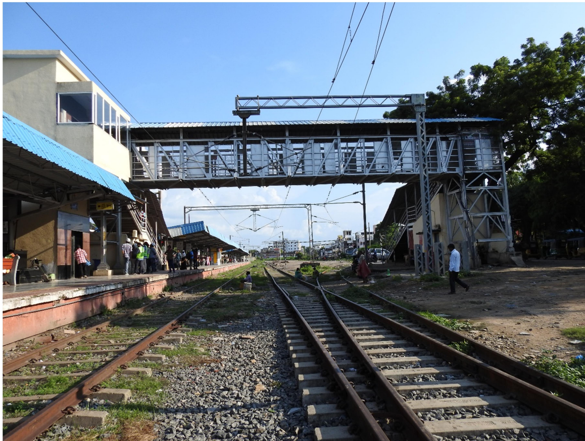
Fig 1(b): Front view of FOB span 2 towards Madira
