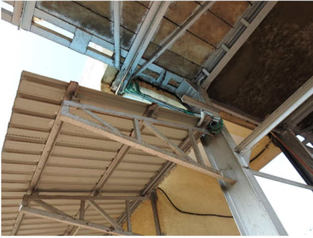
Fig 6: shed for lift is supported on Trestles
