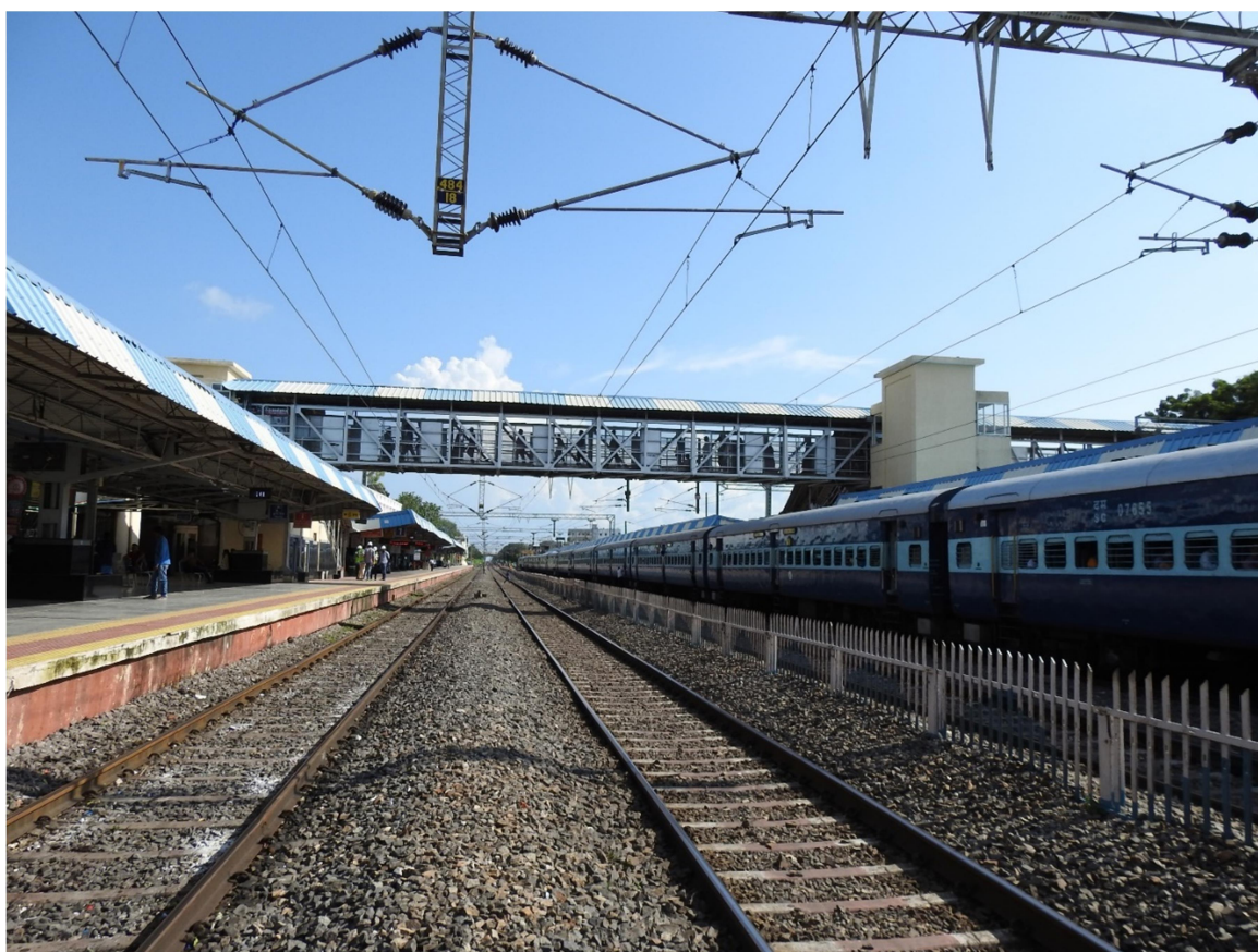
Fig 1(a): Front view of FOB span 1 towards Madira
