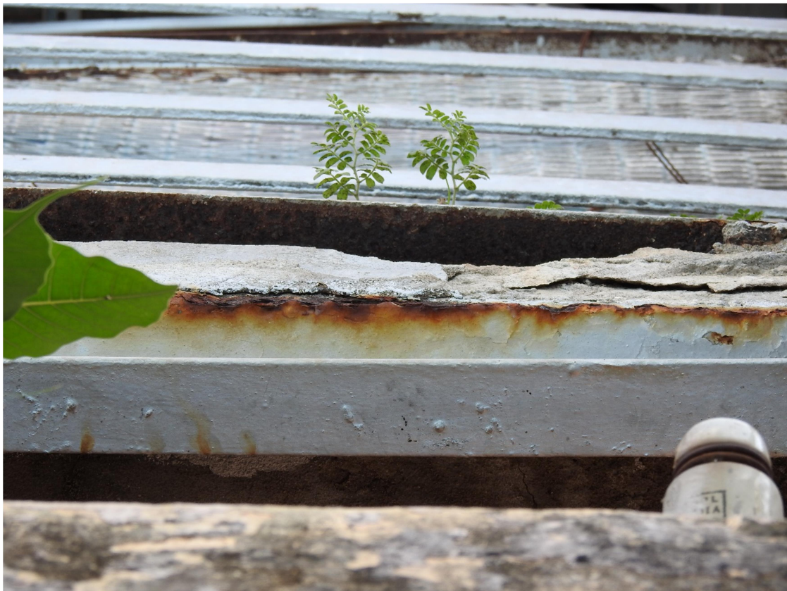
Fig 5: Vegetation is observed along the length of FOB
