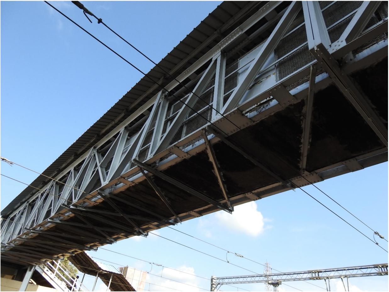
Fig 9: span 1 bottom view
