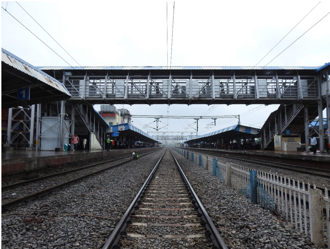
Fig 1(a): Span 1 Front view of FOB towards Khammam
