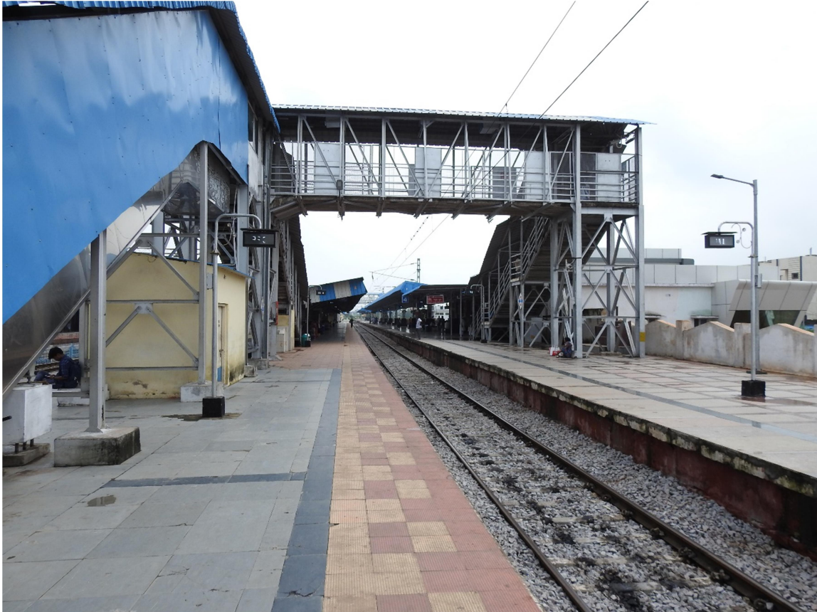
Fig 1(b): Span 2 Front view of FOB towards Khammam
