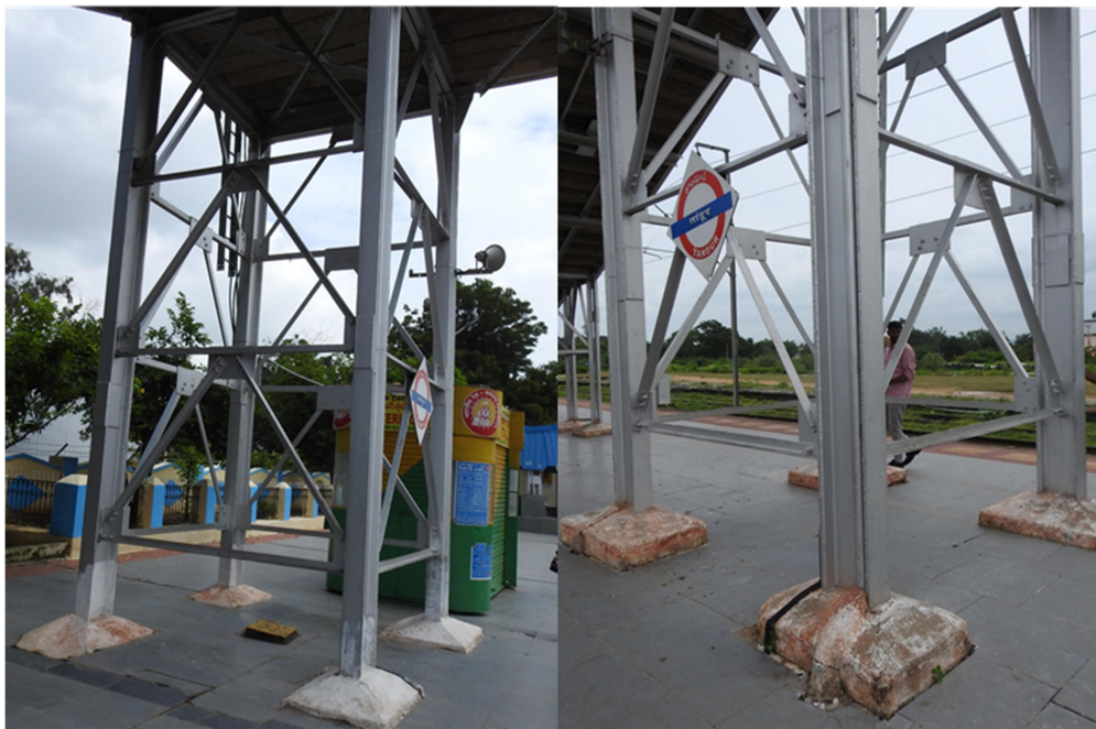
Fig 5: Concrete encasement is provide for ISMB columns
