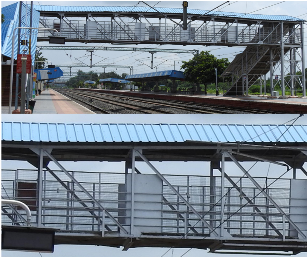
Fig 8: View of Steel Truss
