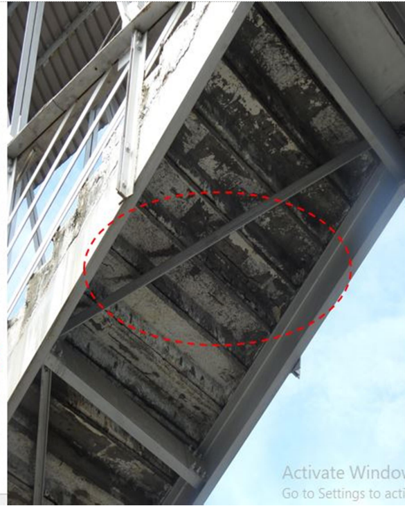
b) Spalling and cracks on staircase steps
