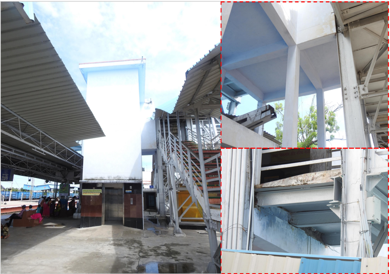
Fig 7: Lift connected to Trestle at Plat form 2
