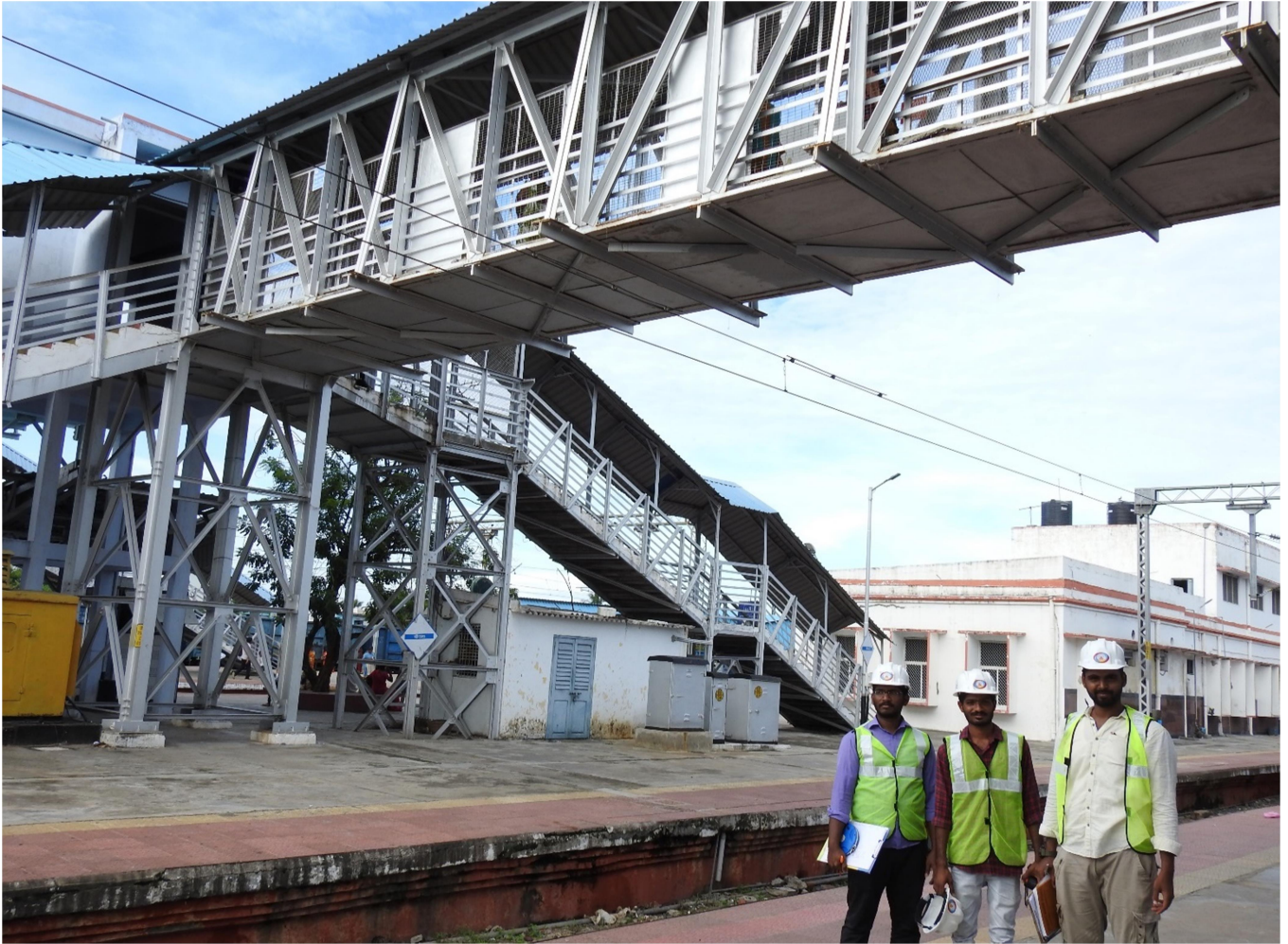
Fig 9: Inspection Team at Chirala FOB
