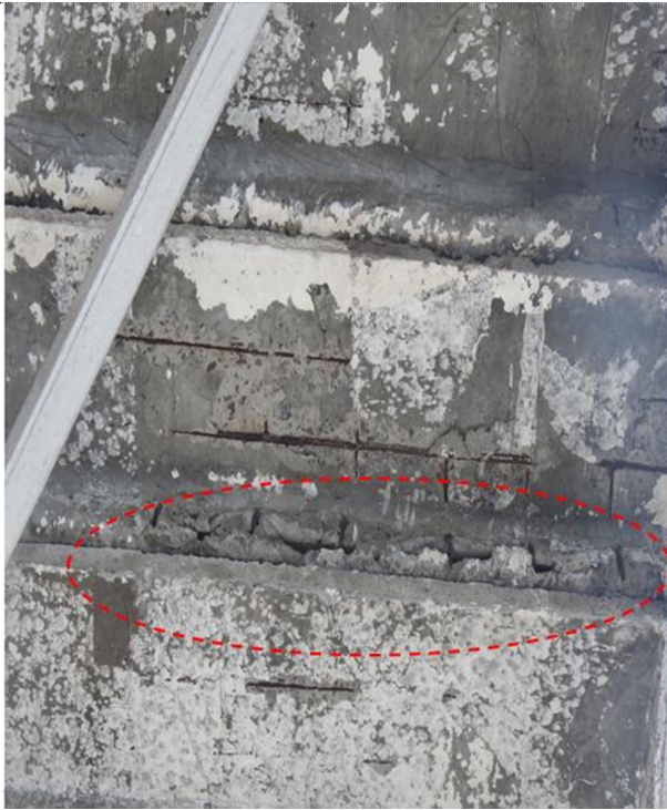
b) Spalling and cracks on staircase steps
