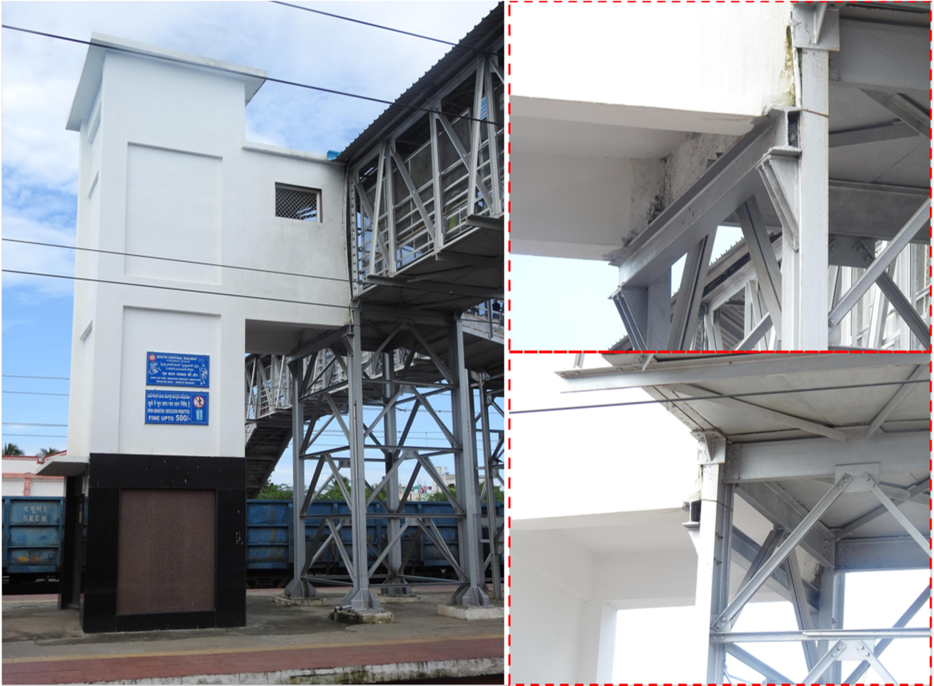
Fig 8: Lift connected to Trestle at Plat form 4
