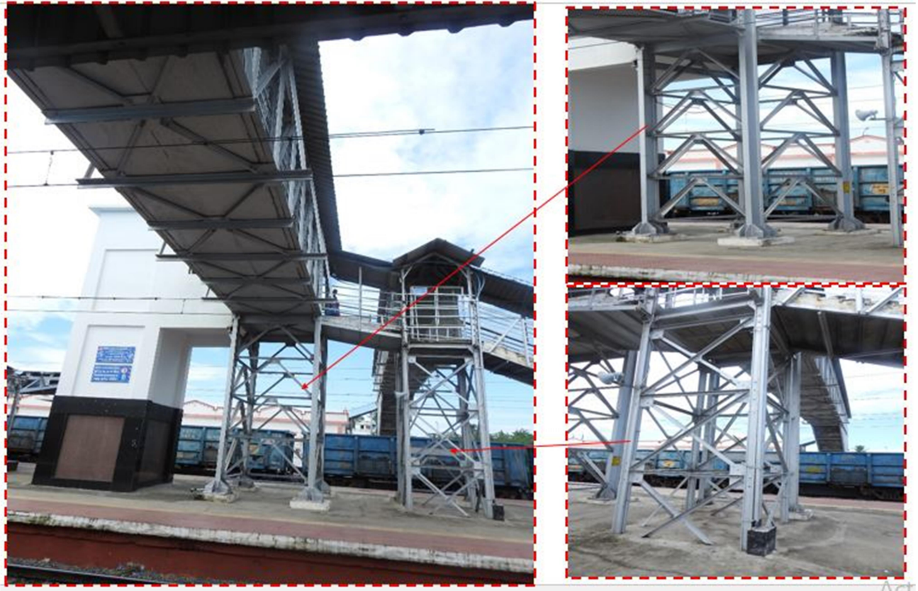
Fig 4: Stanchion column sections details
