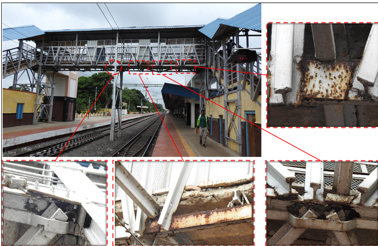
(a) Corrosion observed at floor beams
