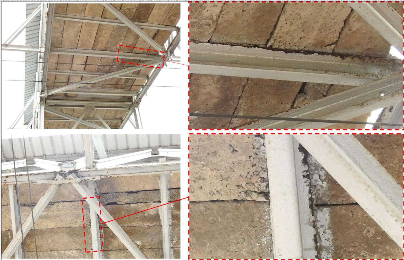
(a) Corrosion observed at floor beams
