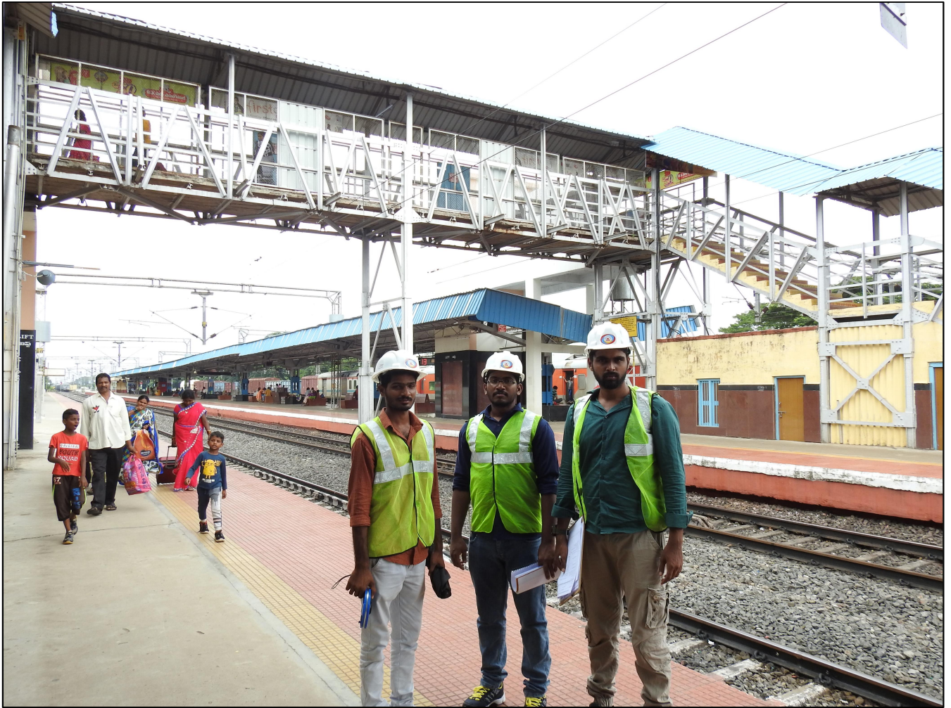
Fig 10: Inspection Team at Eluru FOB
