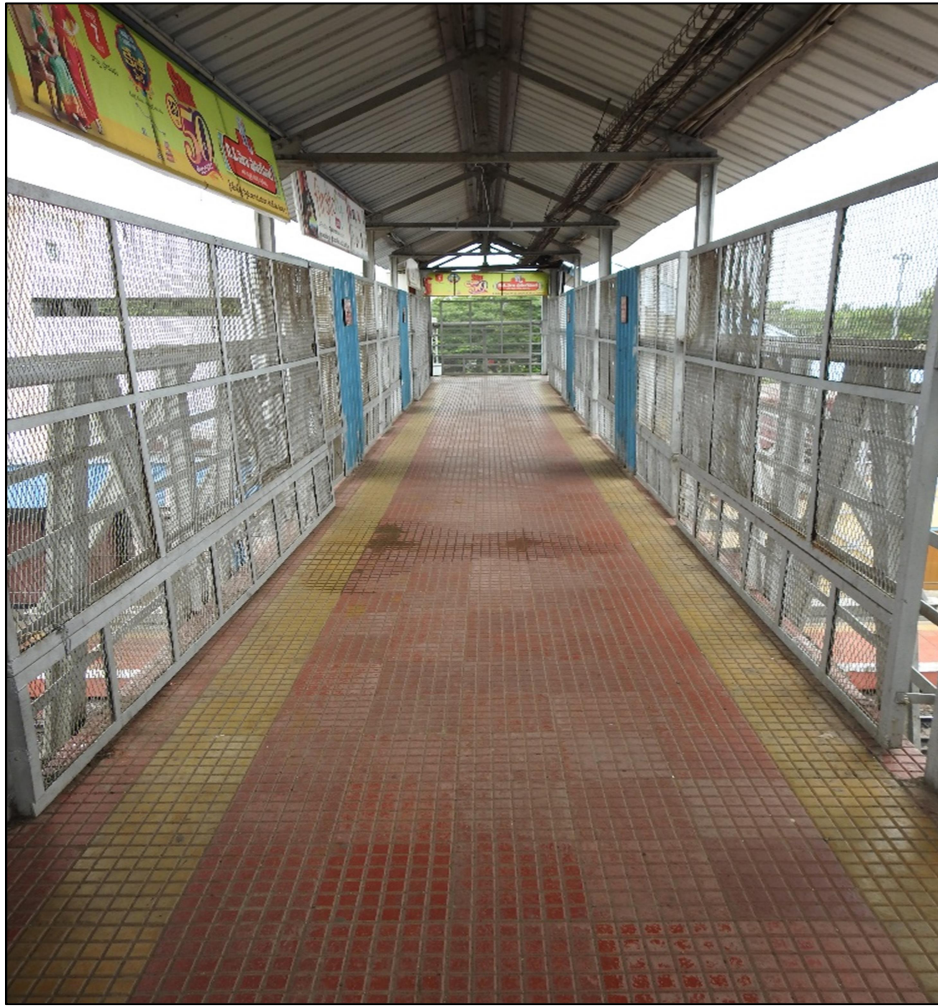
Fig 2: FOB span 1 & 2 pathway, Roof Truss, Chequered tiles, protective screen and Hoardings
