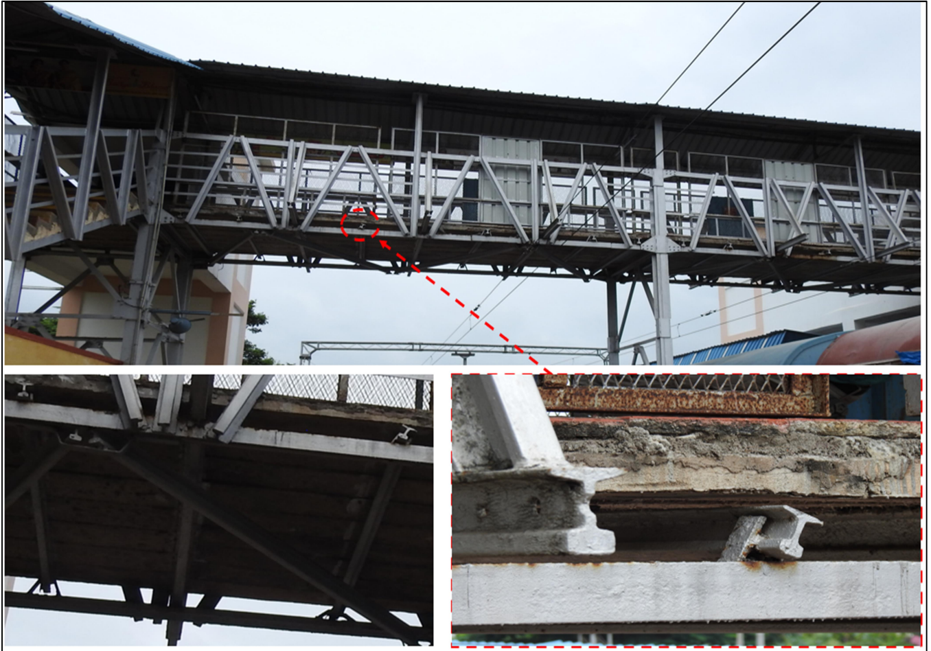
(a) Deformations in floor beam of span 1
