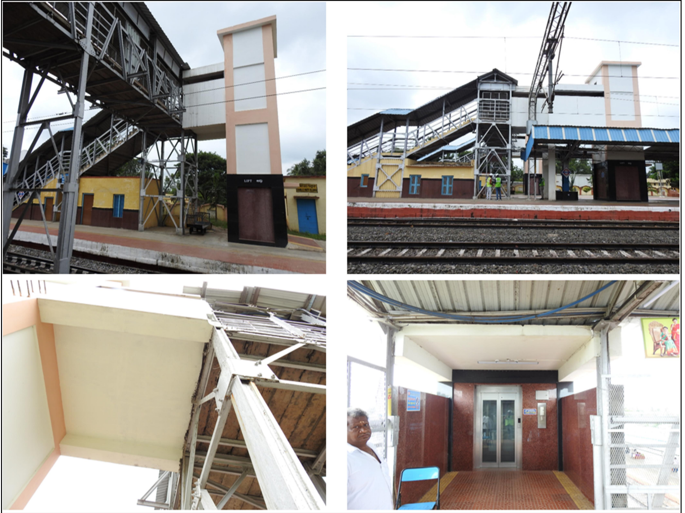
Fig 5: Lift is connected to staircase landing in both platforms
