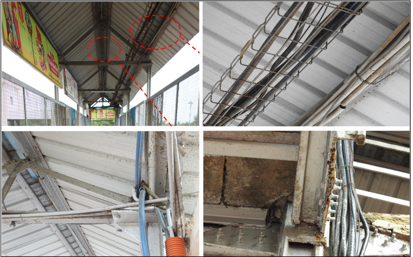
Fig 3: Additional loads of HDPE, PVC pipes
