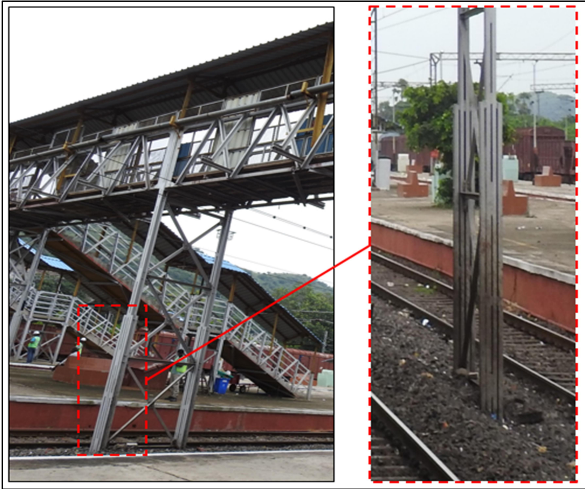
Fig 4: Stanchion column Rail sections details
