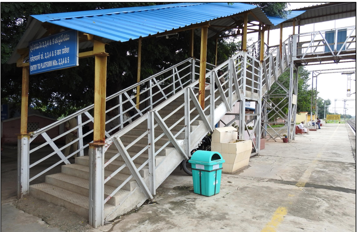
Fig 7: Staircase side view of FOB
