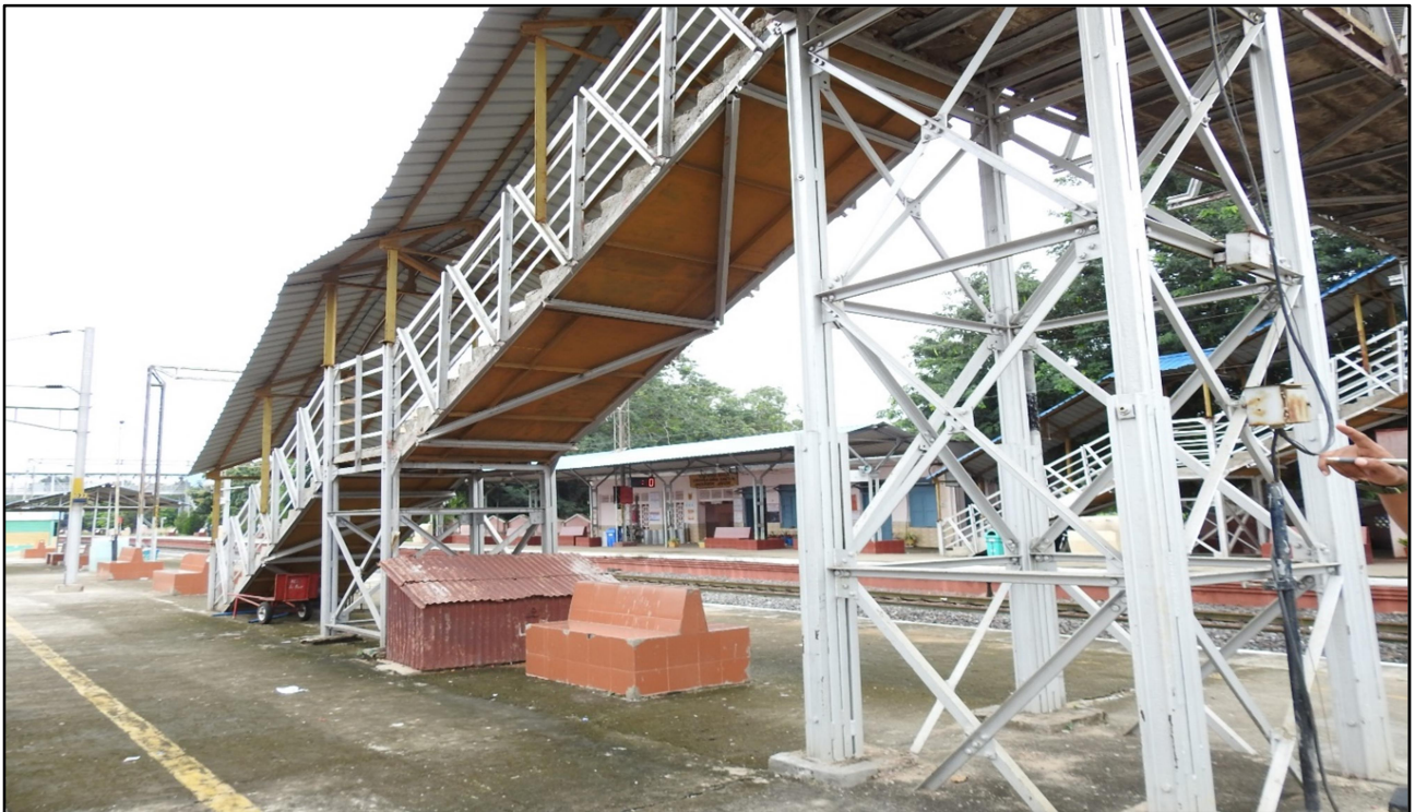
Fig 5: Staircase bottom view
