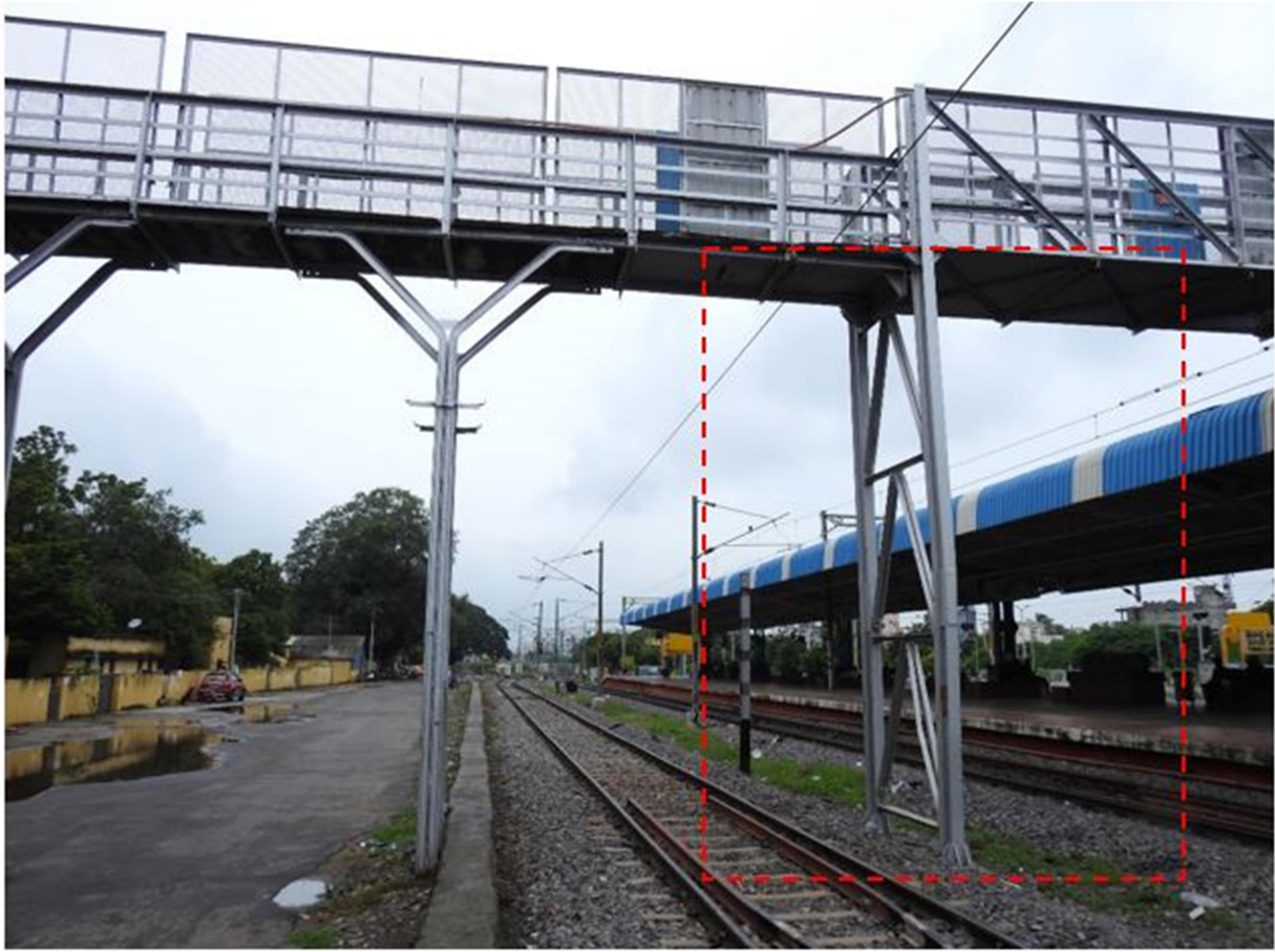
(a) Deformation observed in Stanchion-7 column and bracing
