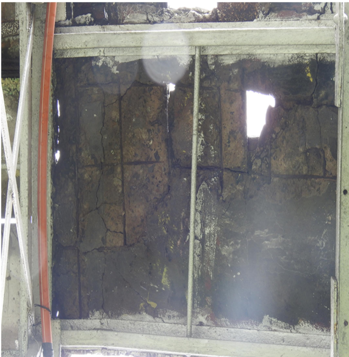
Fig 6: Patch work is observed at slab panels of stair case landing
