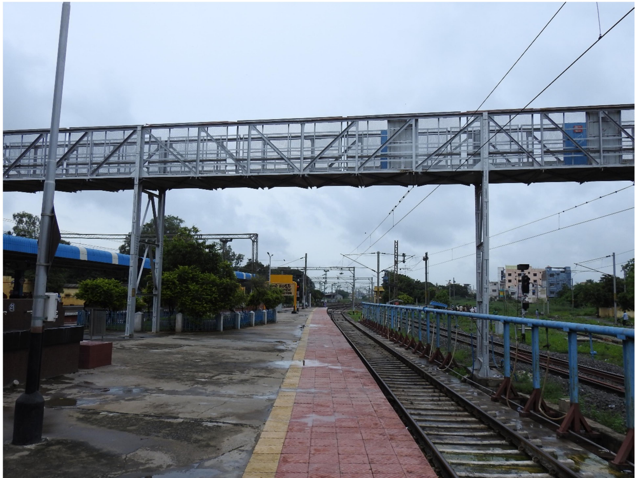
Fig 1: Front view of FOB span 4, 5 & 6
