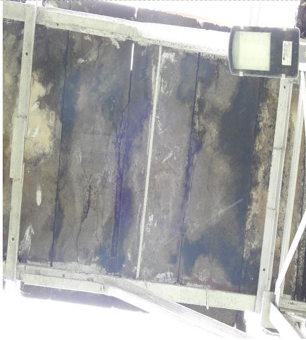
a) Leaching effect and Cracks are observed on Pre-cast slab panels
