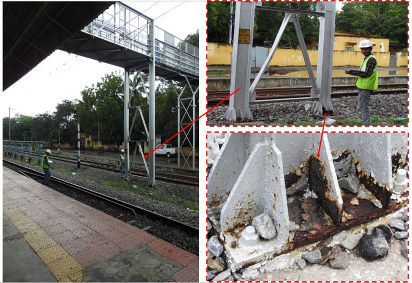
Fig 4: Stanchion column sections details
