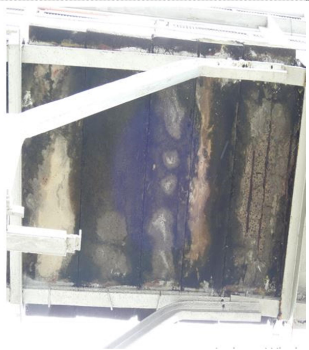
a) Leaching effect and Cracks are observed on Pre-cast slab panels
