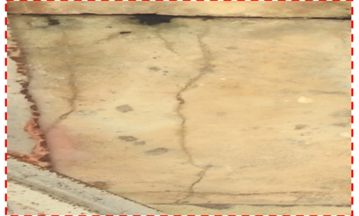
a) Reinforcement exposed at slab panels of 1 st span
