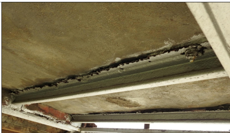
d) Corrosion of floor beam and Patch work observed at landing
