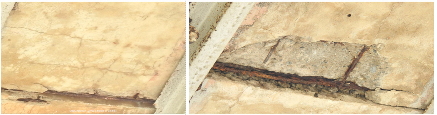
a) Reinforcement exposed at slab panels of 1 st span
