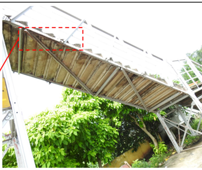
e) Rusting and corrosion observed at Stringer beams
