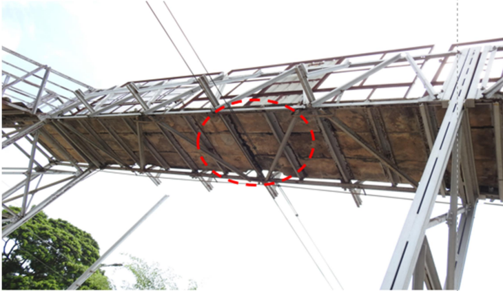
a) Reinforcement exposed at slab panels of 1 st span
