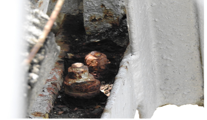
c) Rusting and Corrosion of bottom chord
