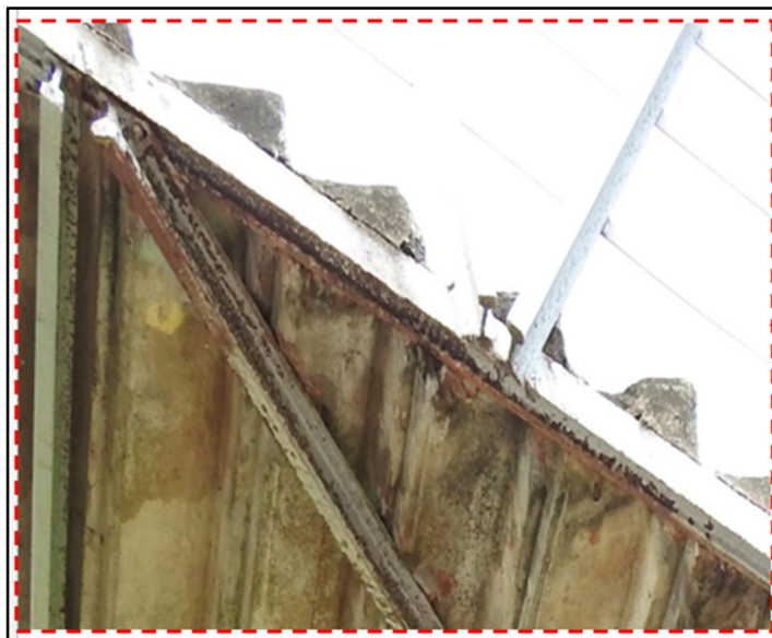
e) Rusting and corrosion observed at Stringer beams
