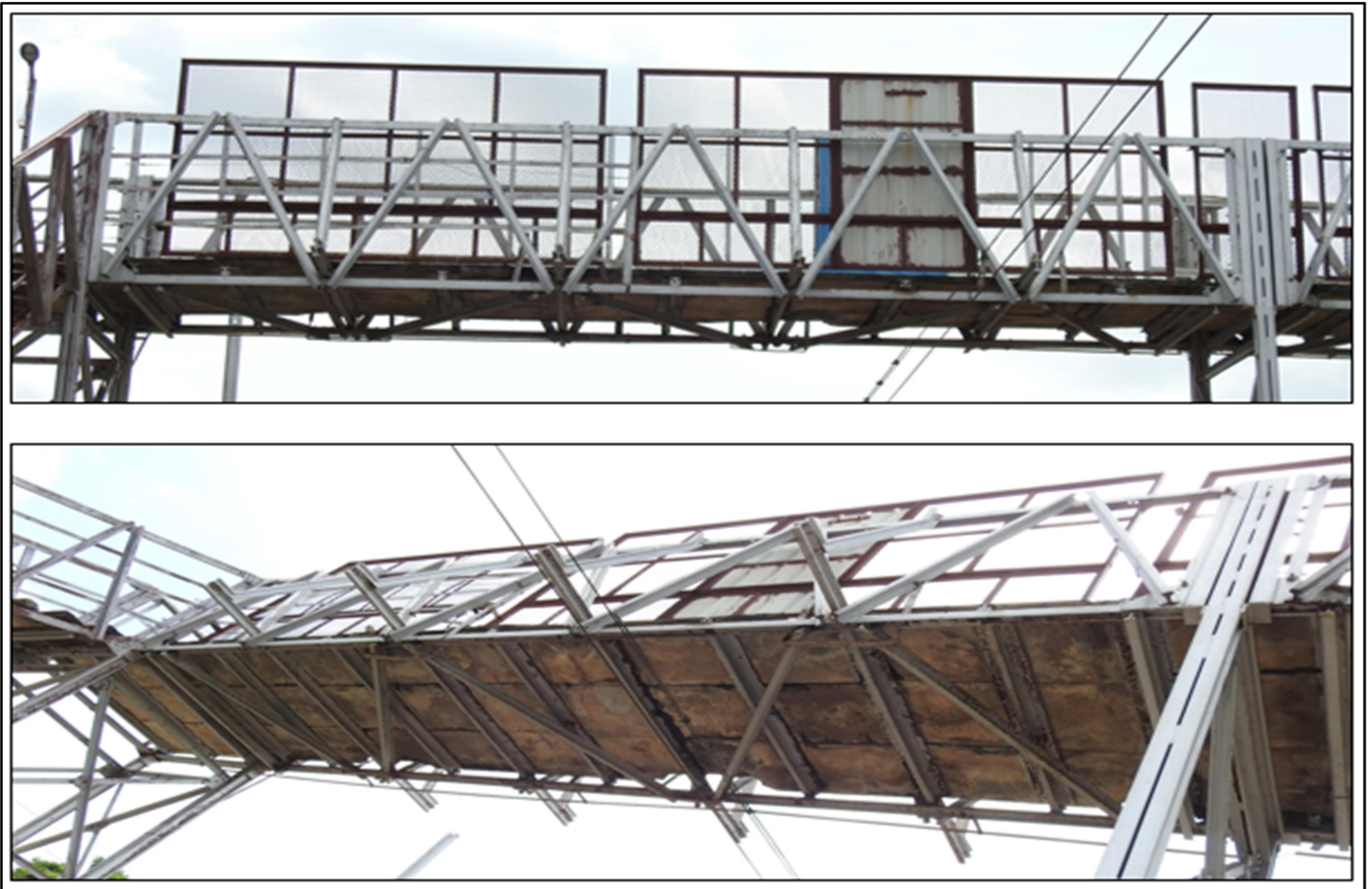
Fig 6: Span 2 Side view and Bottom View
