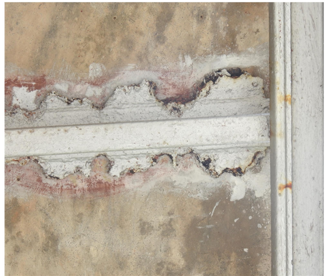
c) Rusting and Corrosion of bottom chord
