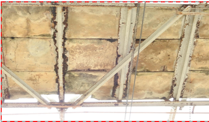
b) Reinforcement exposed at slab panels of 2 nd span
