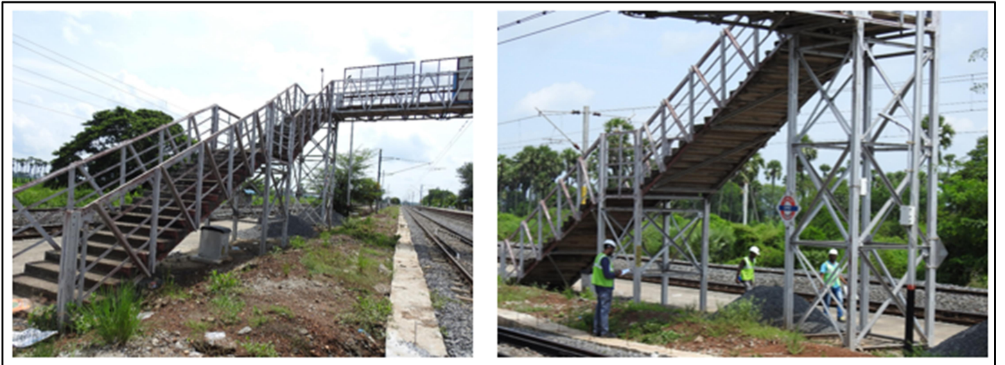
Fig 4: Staircase-2 Trestles details
