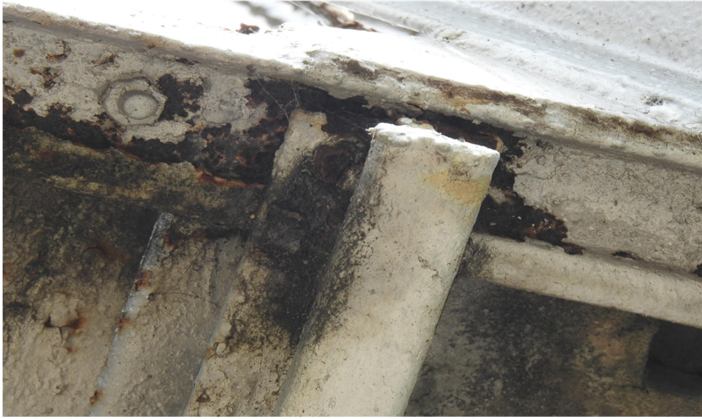
c) Rusting and Corrosion of bottom chord
