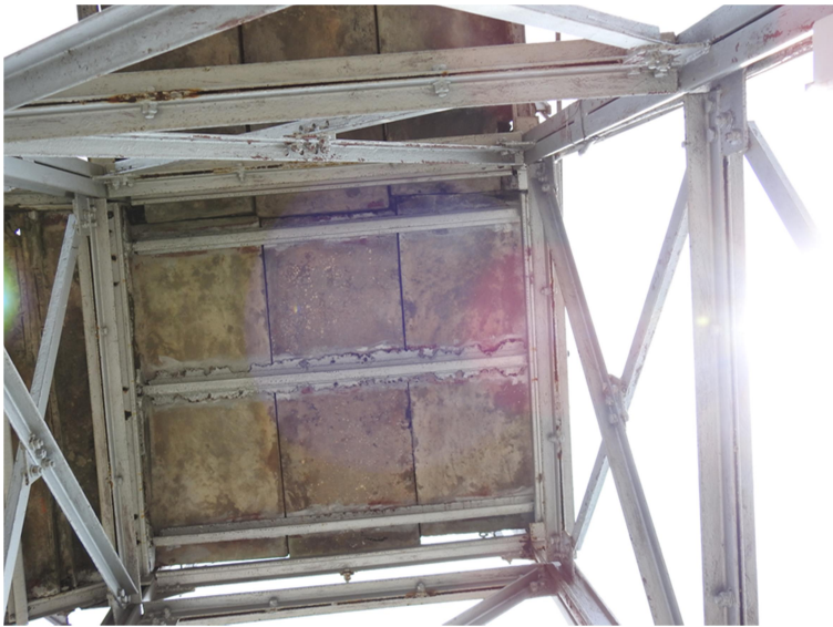
c) Rusting and Corrosion of bottom chord
