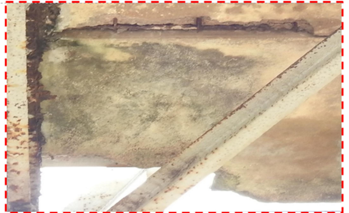
b) Reinforcement exposed at slab panels of 2 nd span
