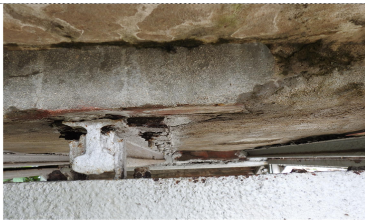
d) Corrosion of floor beam and Patch work observed at landing
