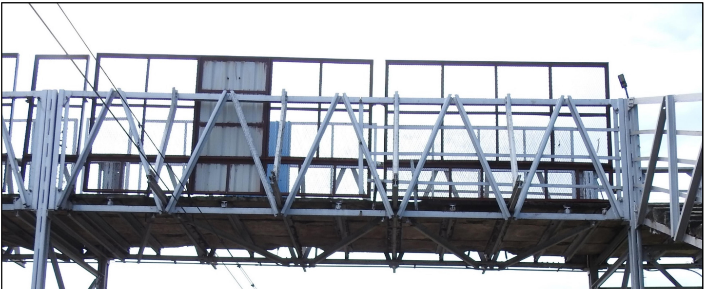
Fig 5: Span 1 Side view and Bottom View
