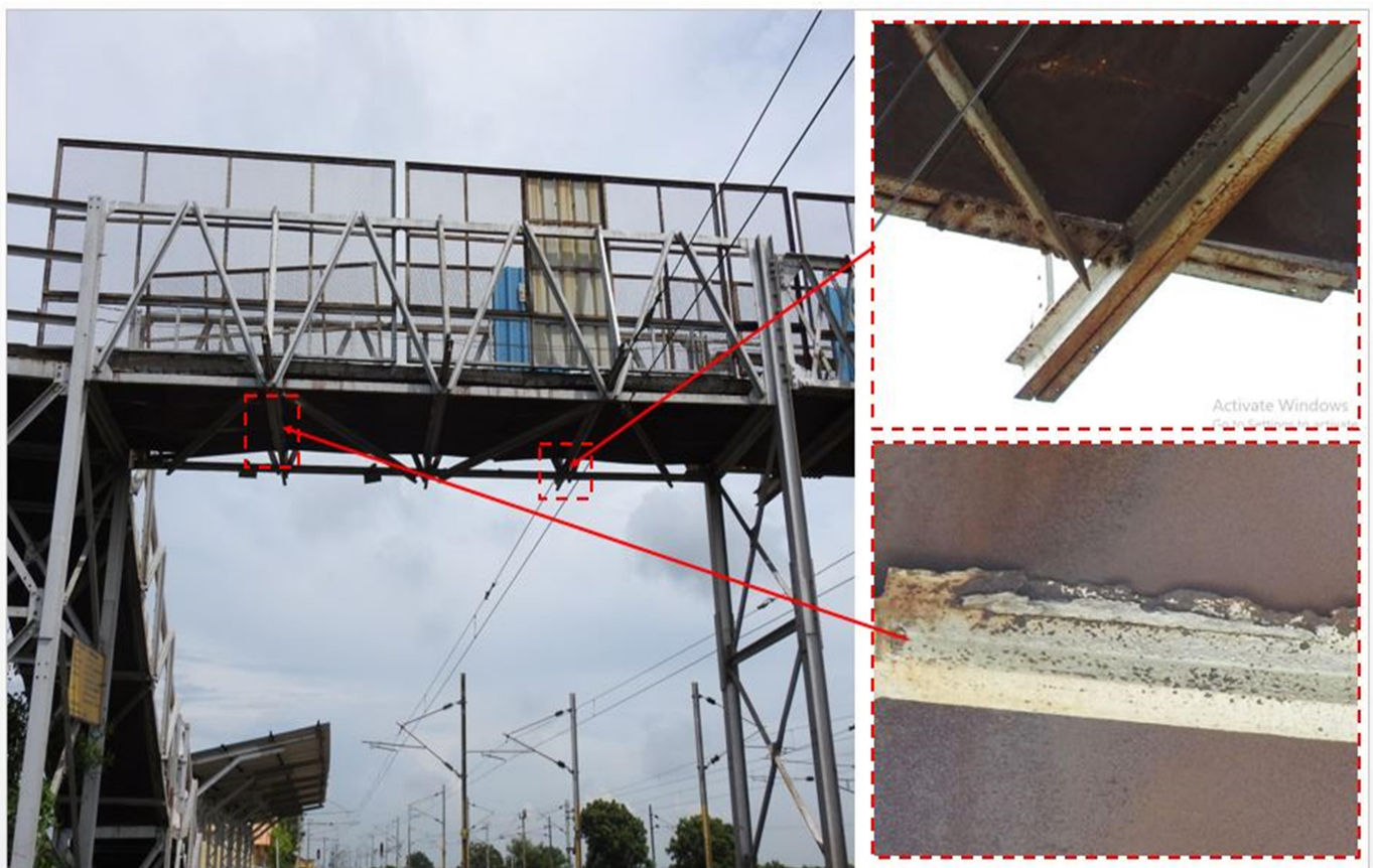
c) Rusting and Corrosion At Span-3
