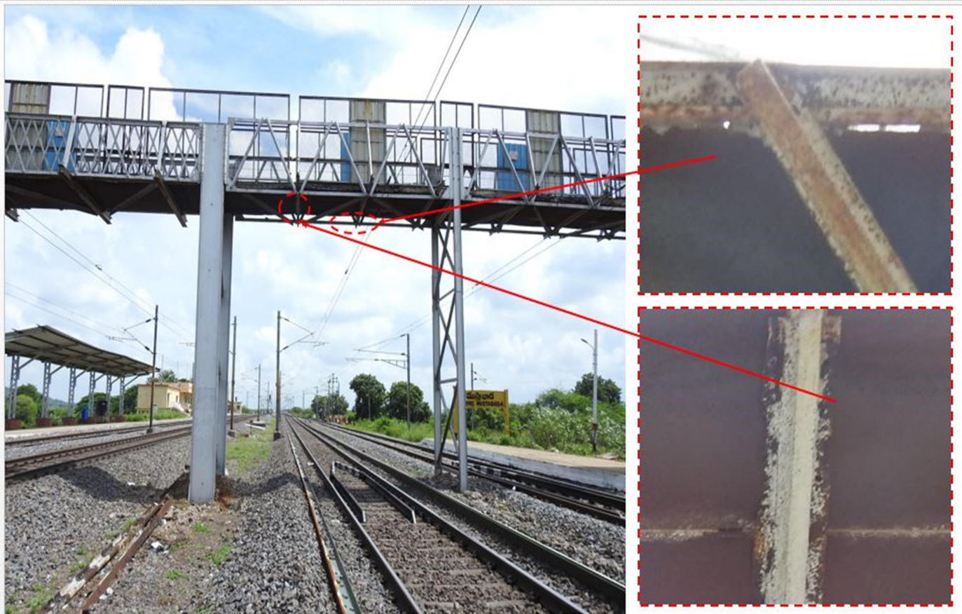
c) Rusting and Corrosion At Span-3
