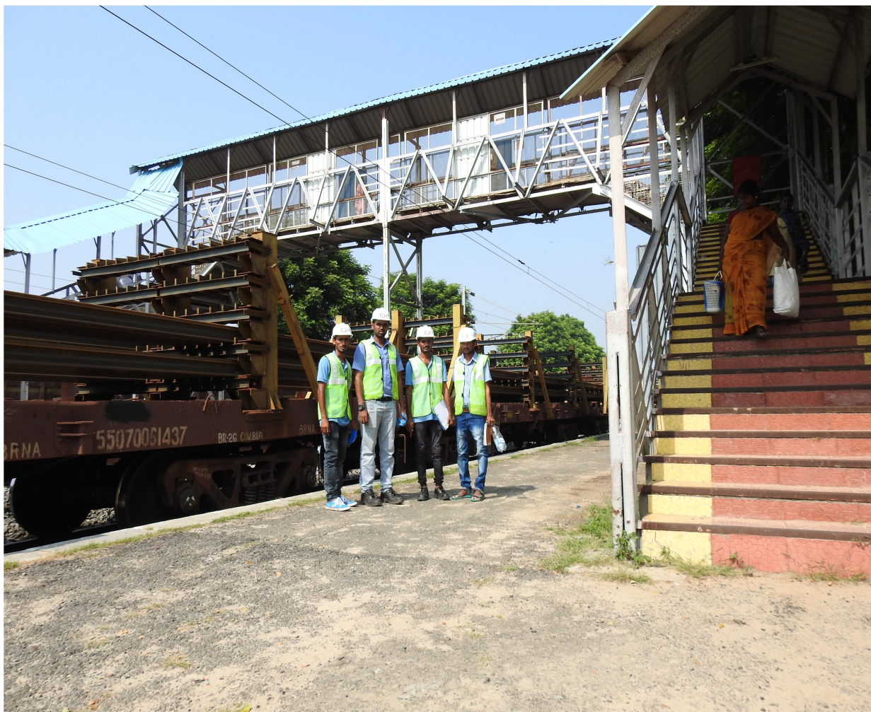
Fig 7: Inspection Team at Chinnaganjam FOB
