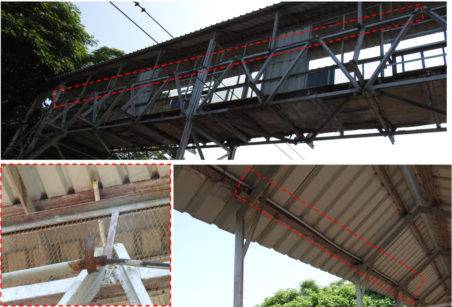
Fig 3: Additional loads of HDPE, PVC pipes
