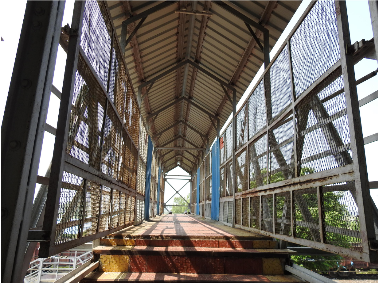
Fig 2: FOB span 1 & 2 pathway, additional wearing coat, protective screen
