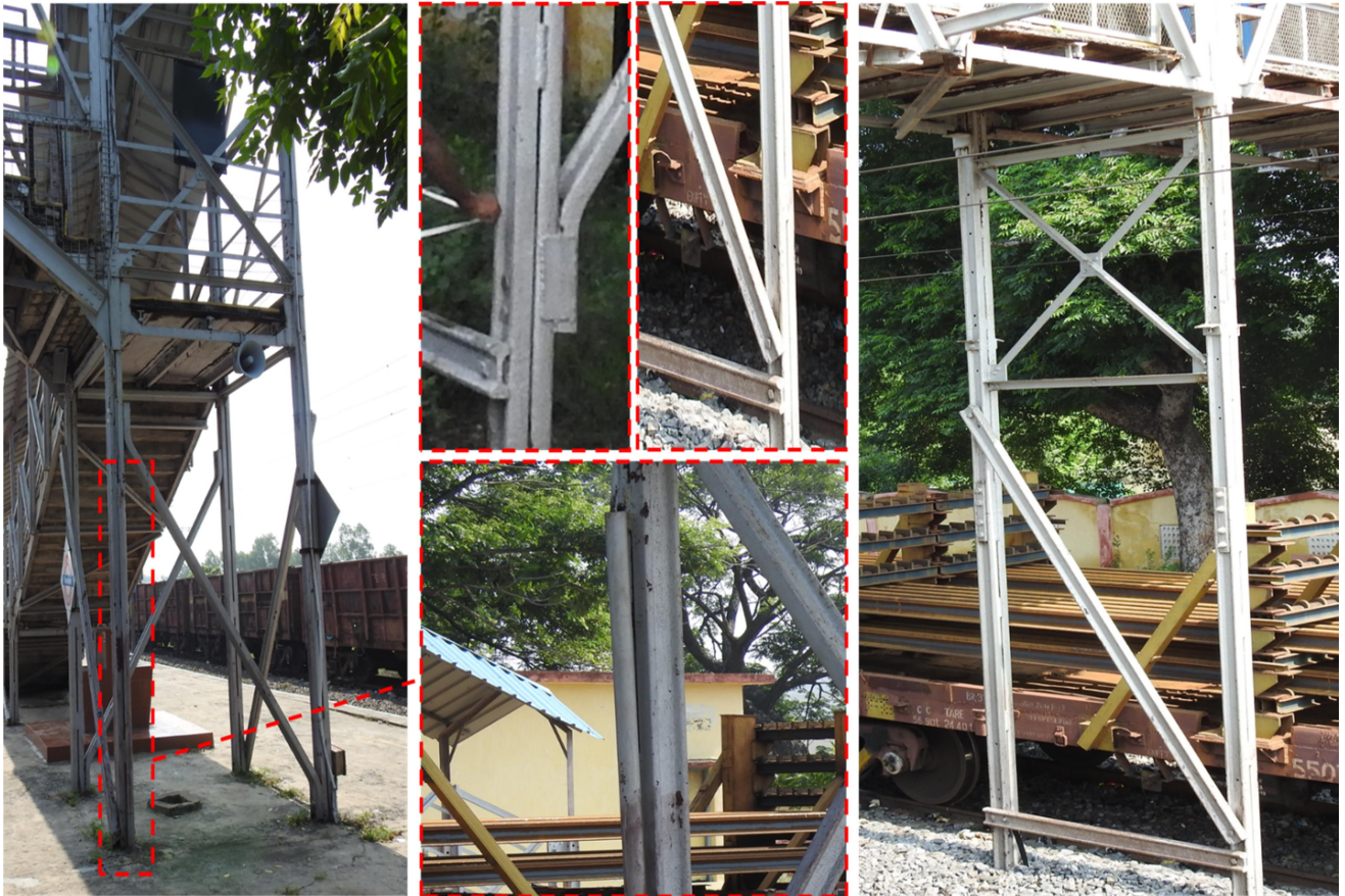
Fig 4: Trestles, Stanchion column Rail sections details.
