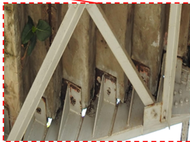
c) Exposed Reinforcement, vegetation and corrosion at cleat angles observed at staircase Span 2
