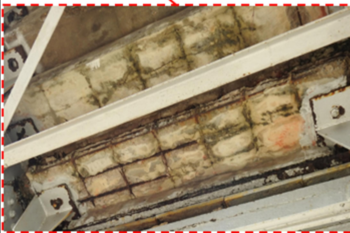
c) Exposed Reinforcement, vegetation and corrosion at cleat angles observed at staircase Span 2
