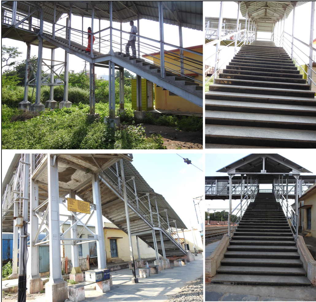
Fig 5(a): View of Staircase-1 and staircase-2
