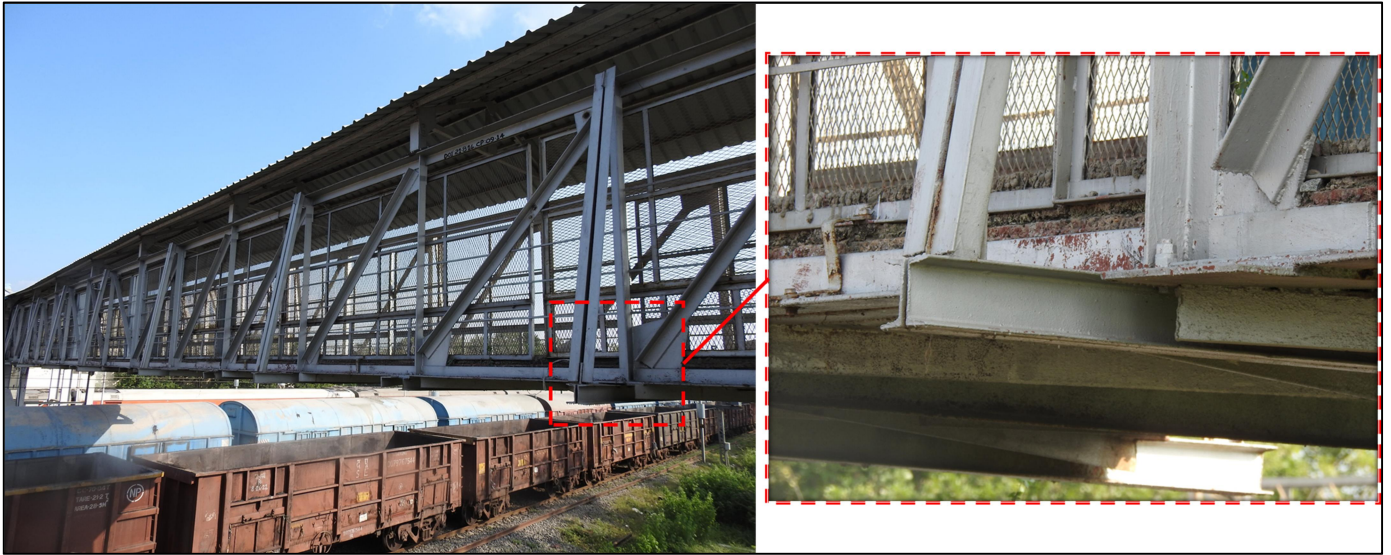
Fig 7: View of Top, bottom and floor beam in span 1 st 2 nd & 3 rd of FOB
