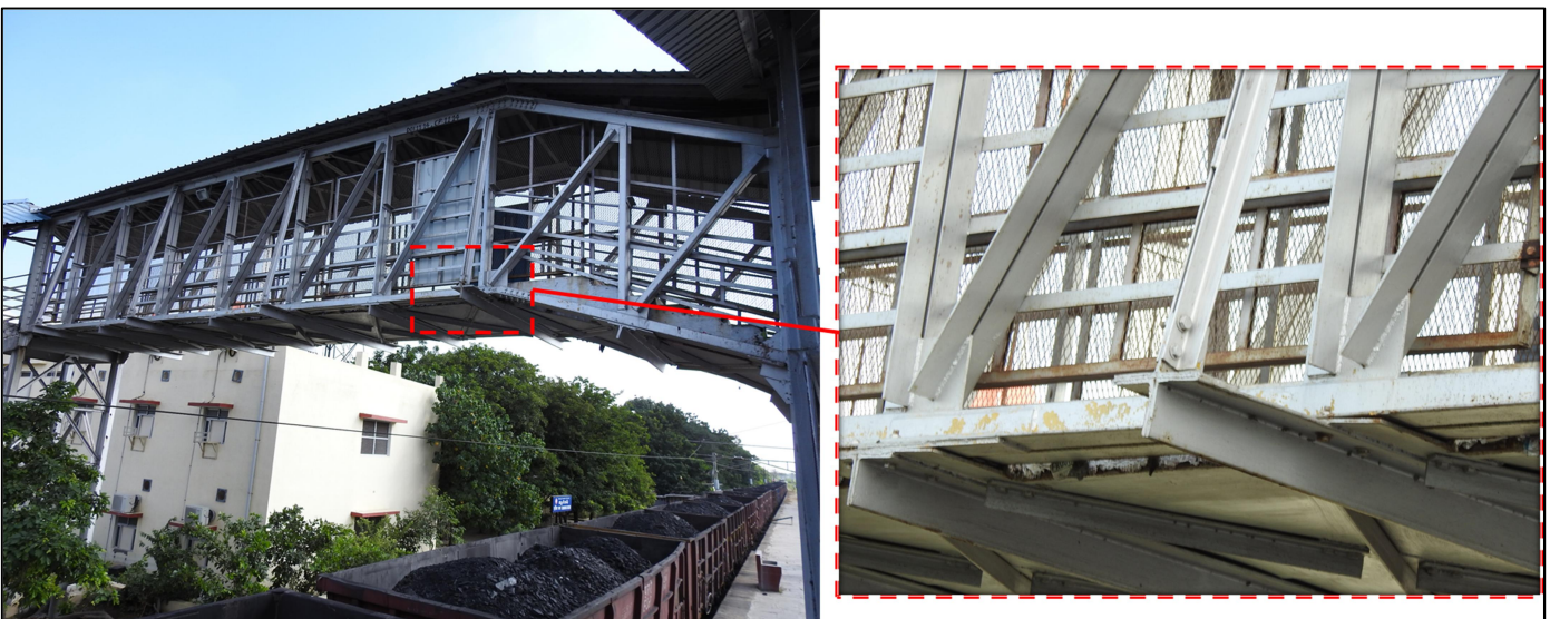
Fig 8: View of Top, bottom and floor beam in 4th span of FOB
