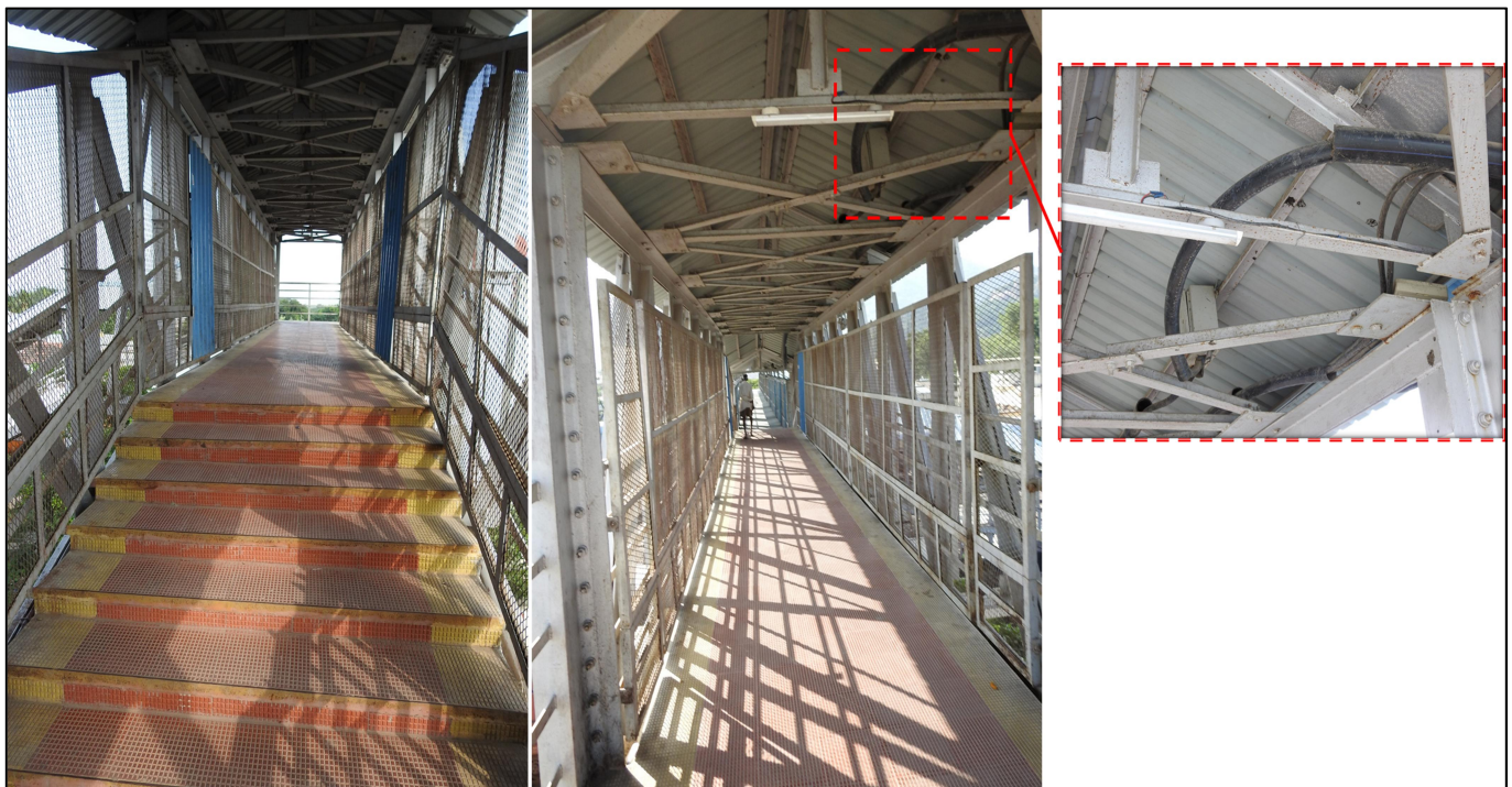
Fig 2(c): FOB pathway, protective screen, Roof truss and cables on 4 th span
