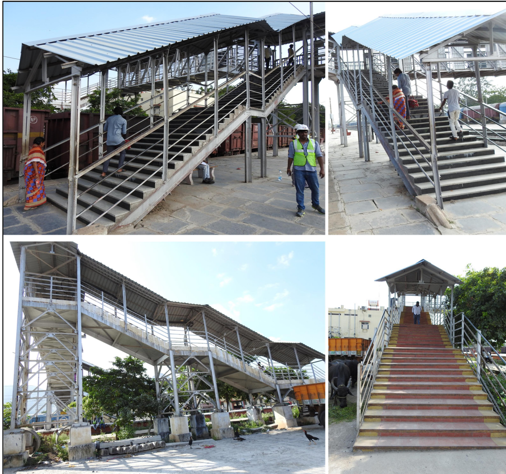
Fig 5(b): View of Staircase-3 and staircase-4
