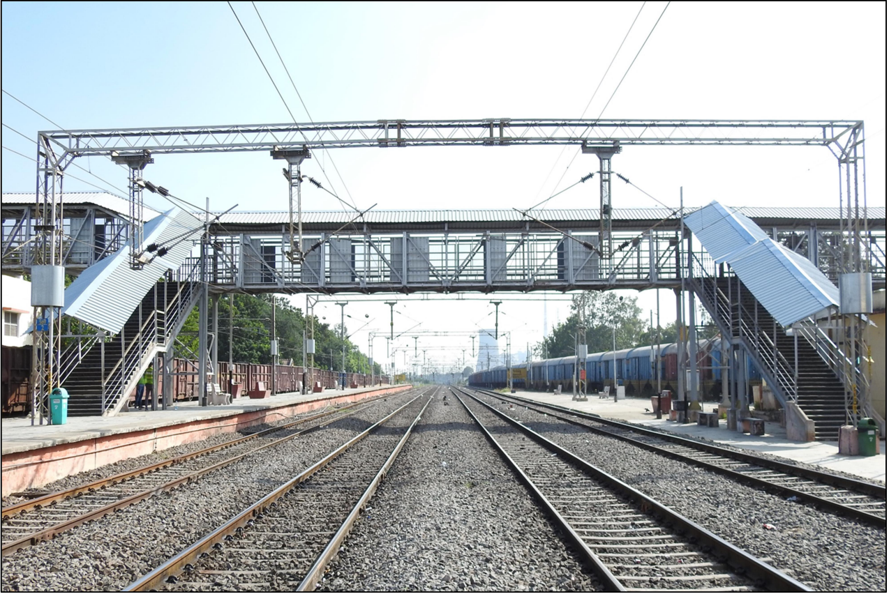
Fig 1(c): View of 3 rd span of FOB
