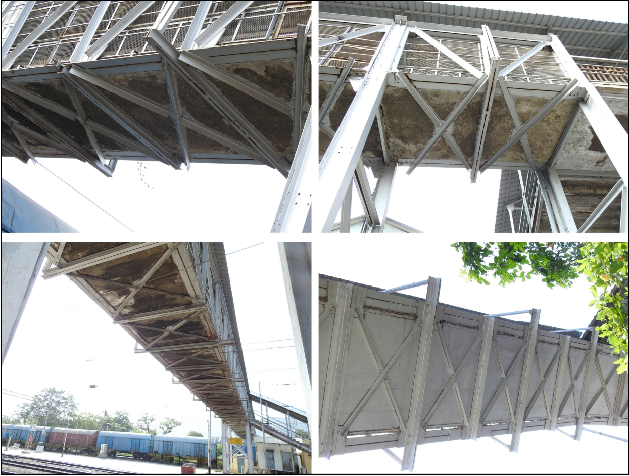
Fig 4: Bottom view of 1 st , 2 nd , 3 rd span and sacrificial plate for 4 th span of FOB
