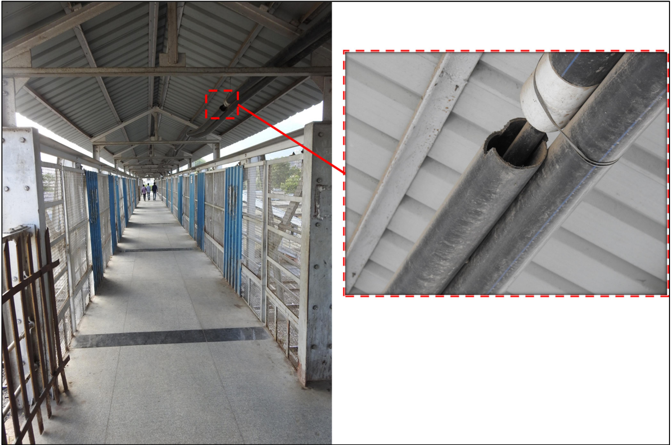
Fig 2(b): FOB pathway, protective screen, Roof truss and cables on 2 nd and 3 rd span
