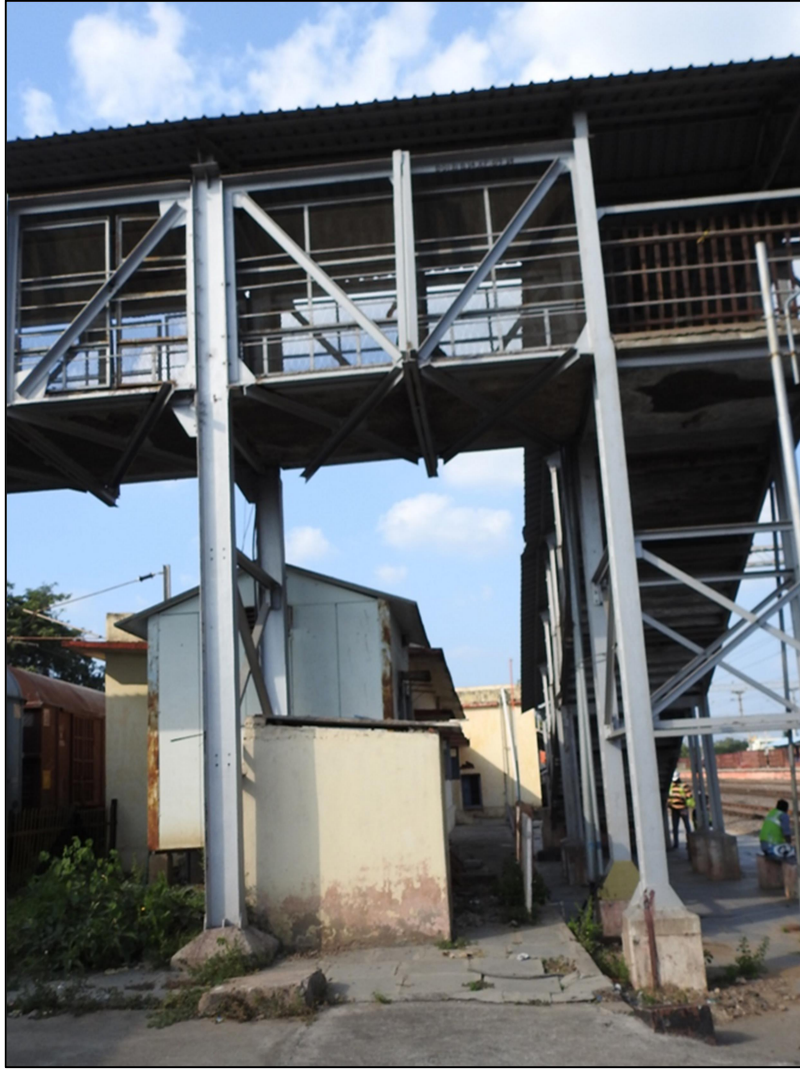
Fig 1(b): View of 2 nd span of FOB
