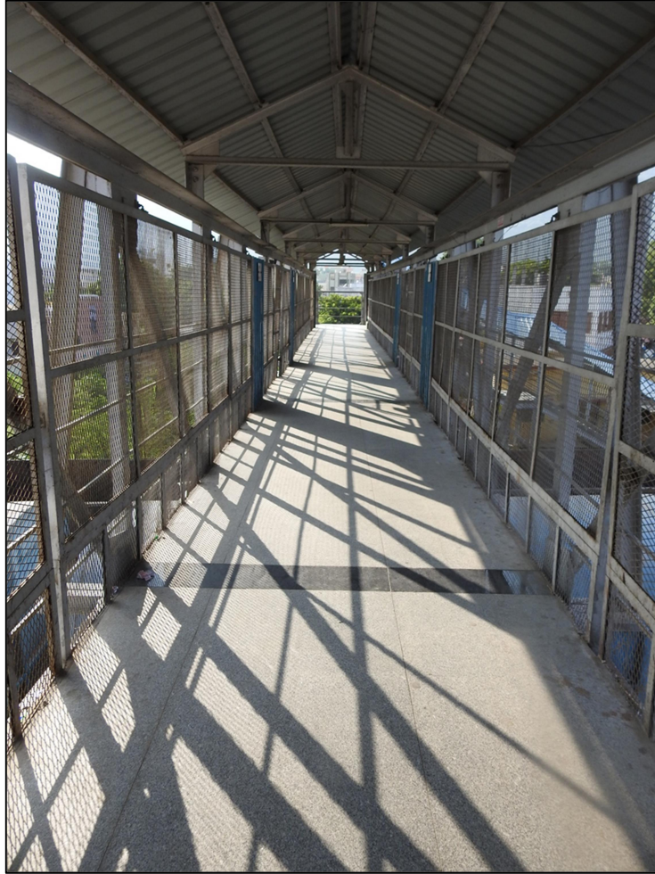
Fig 2(a): FOB pathway, protective screen and roof truss on 1 st span
