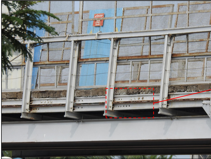
e) Corrosion observed in bottom rail
