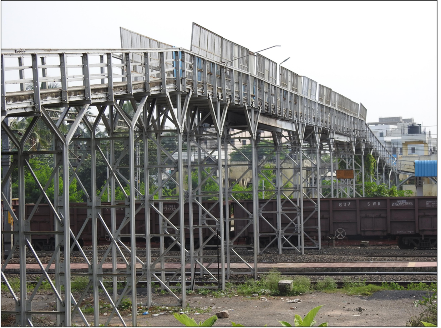
Fig 1: View of FOB and Ramps on both sides
