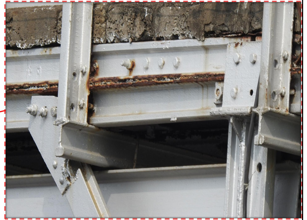
e) Corrosion observed in bottom rail
