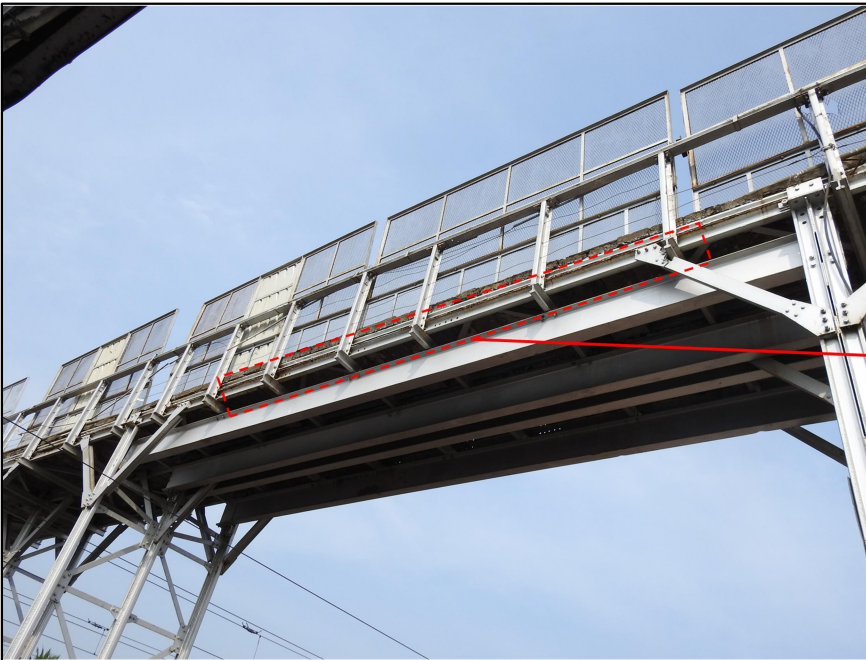
f) Corrosion observed in bottom rail
