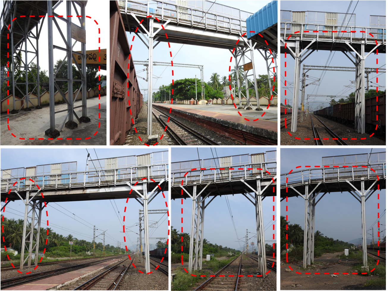
Fig 3: Stanchion column details
