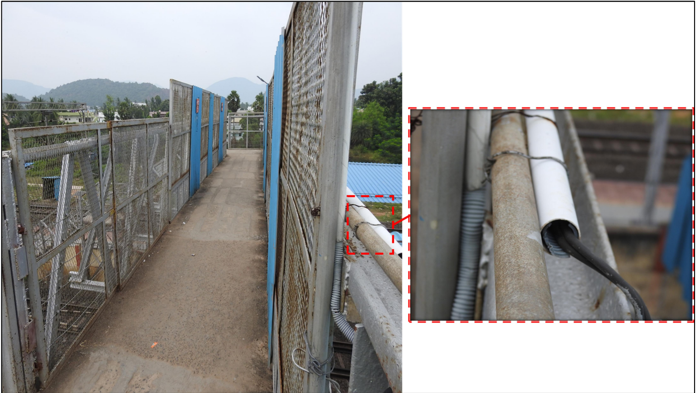
Fig 2: FOB pathway, protective screen and Additional loads of PVC pipes
