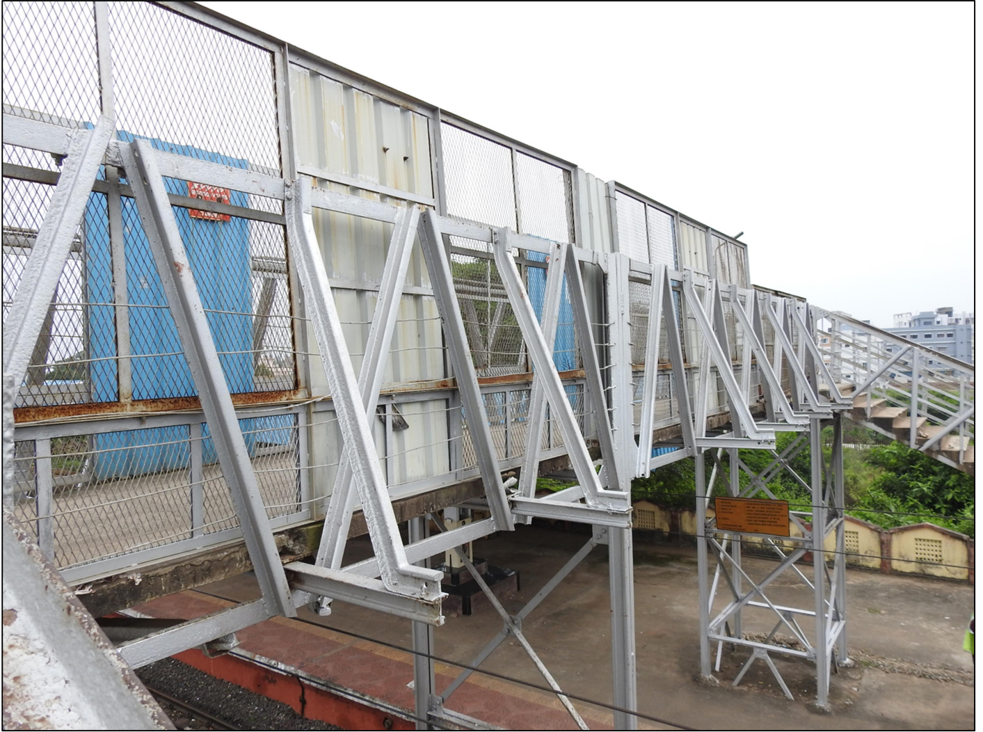
Fig 4: Arrangement of truss
