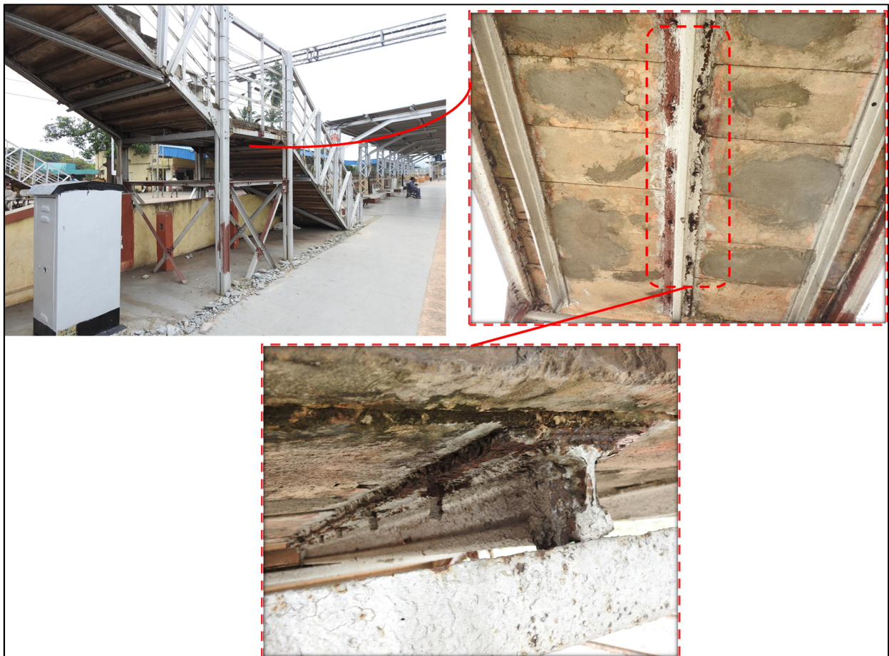
(a) Corrosion of floor beam and stringer beam in staircase-1
