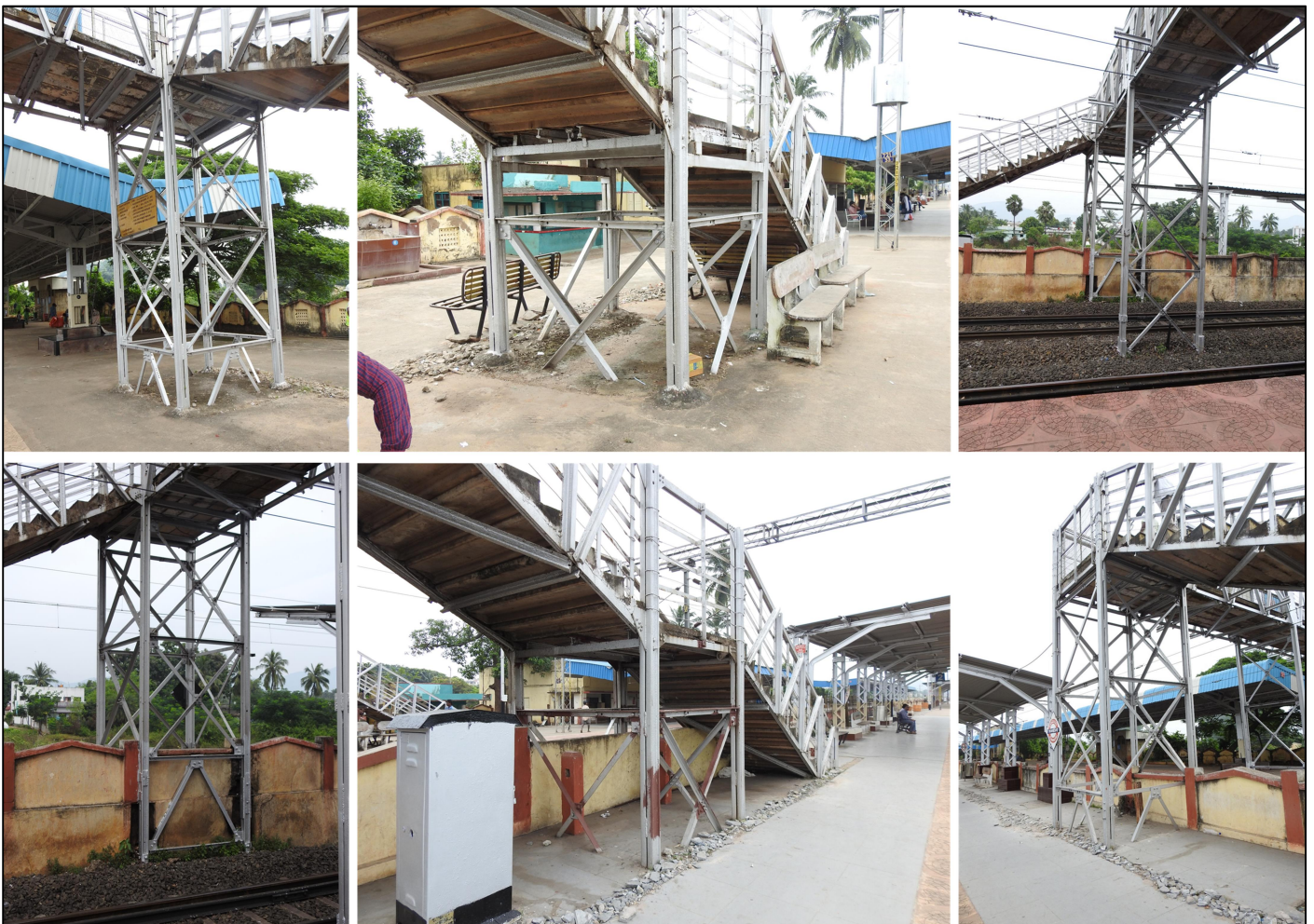
Fig 3: Trestles and Stanchion column details
