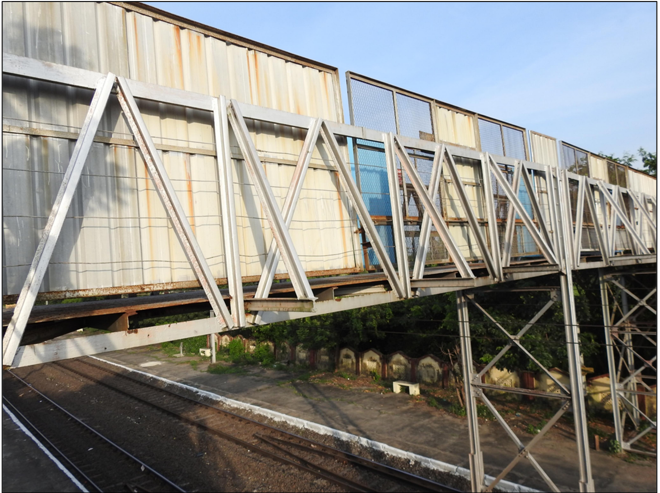
Fig 6: Arrangement of Truss
