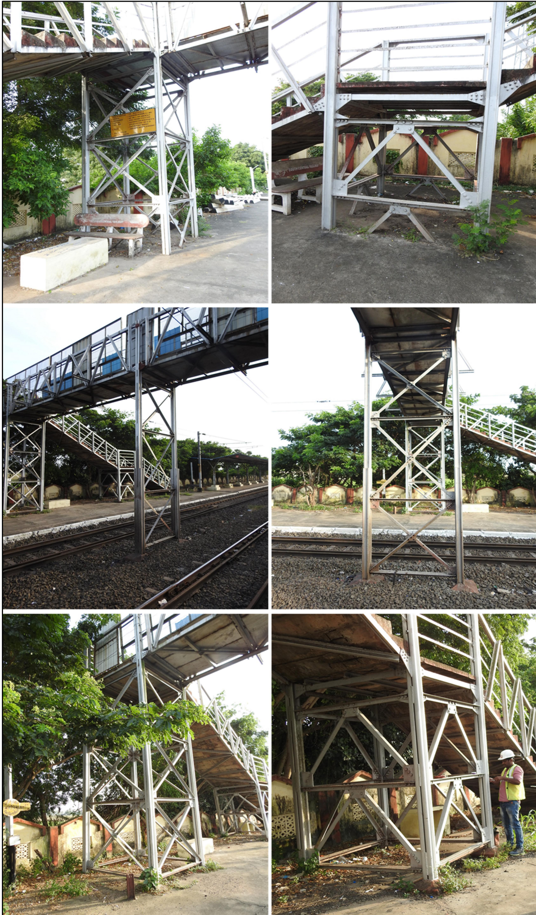
Fig 3: Stanchion column details
