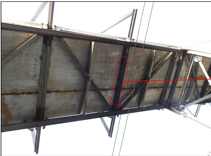
Corrosion of Floor beams
