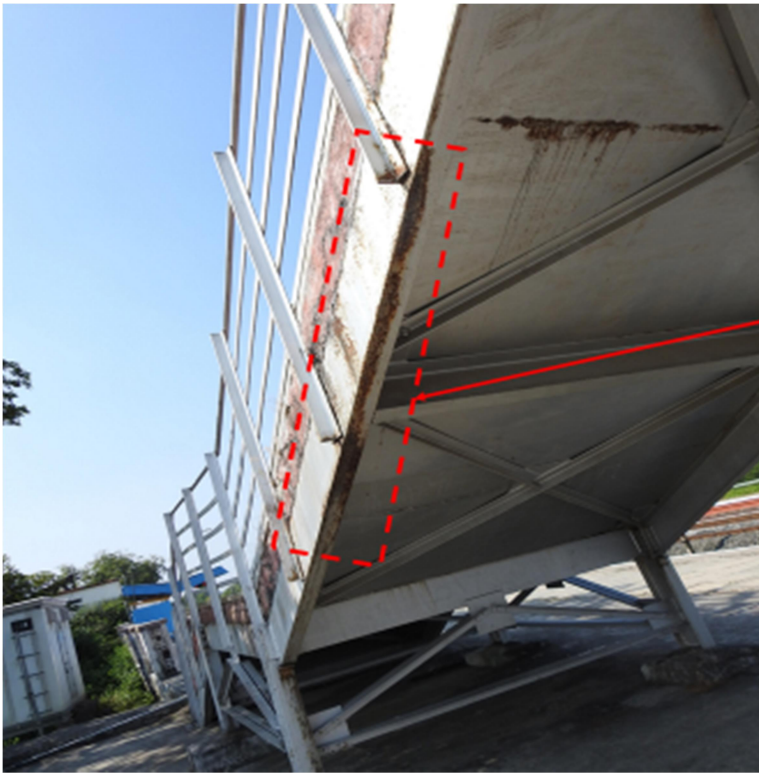
a) Rusting observed at Stringer beam of Staircase-1
