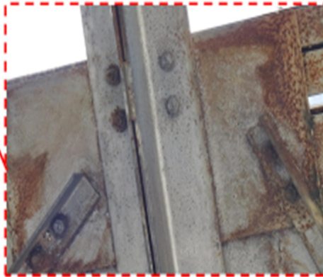
e) Rusting observed at stanchion column tie members
