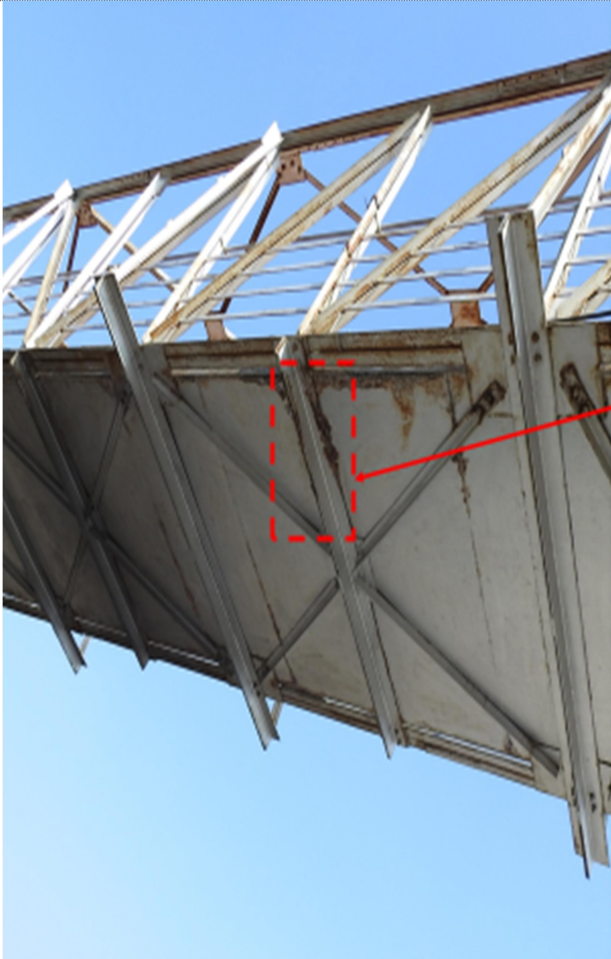
c) Corrosion observed at floor beam of Span-1
