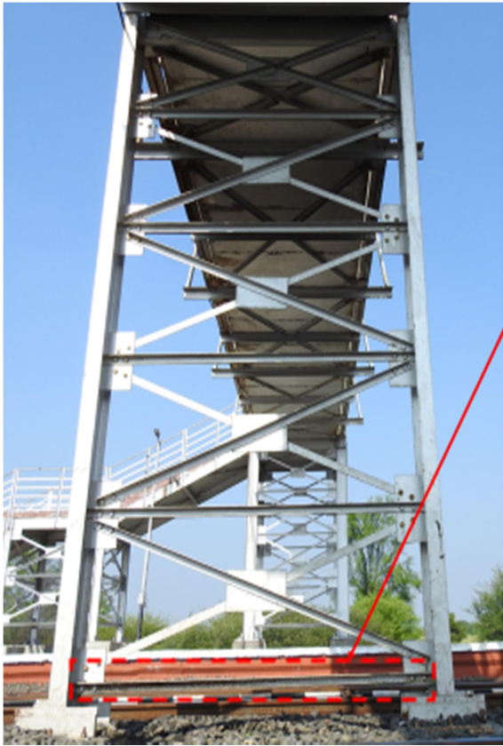
e) Rusting observed at stanchion column tie members
