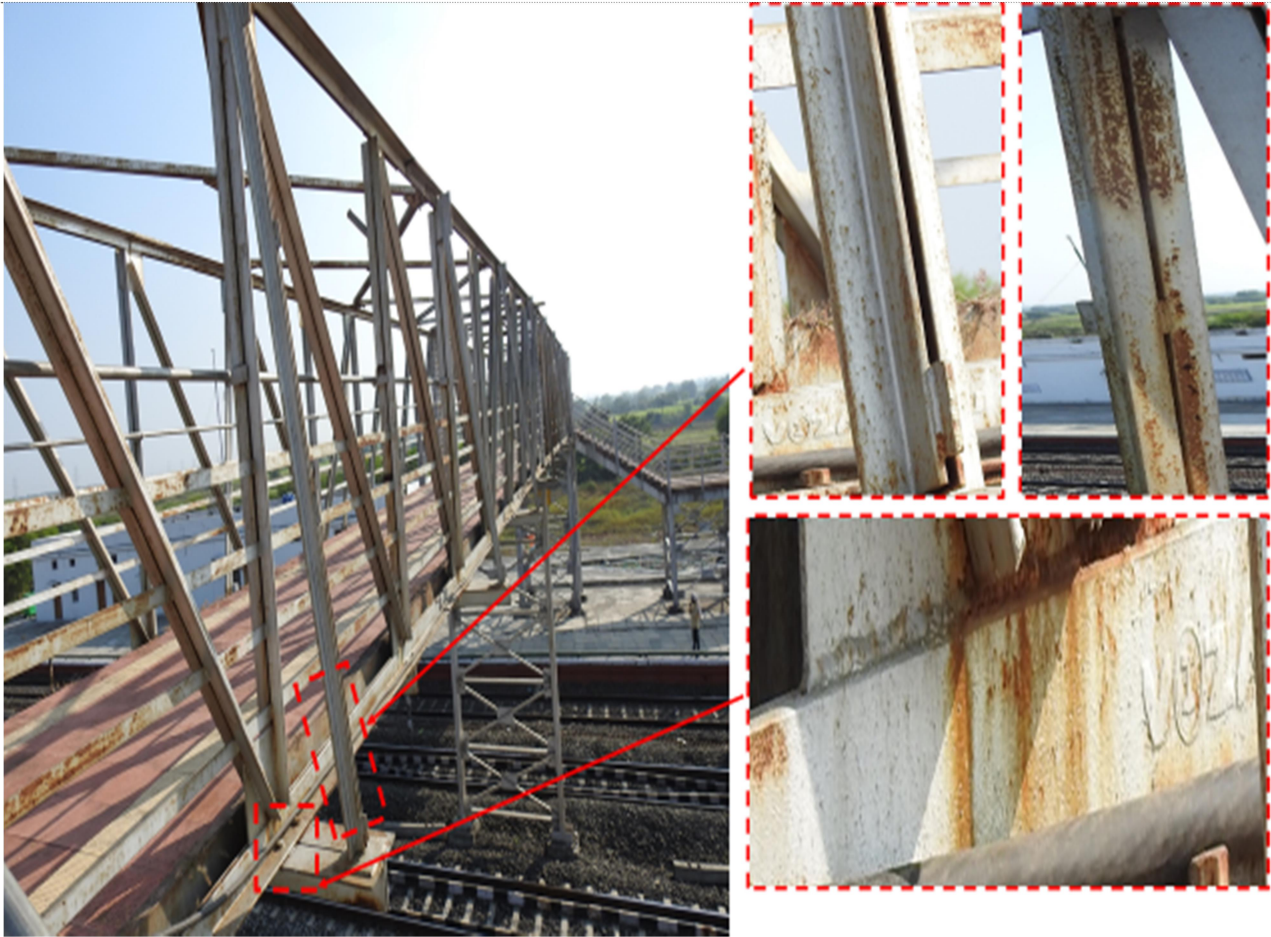
i) Rusting observed at knee bracing, bottom chord of Span-2
