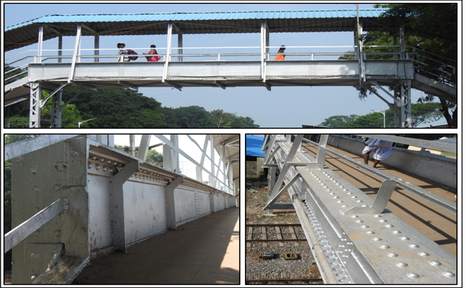
Fig 5: Plate Girder
