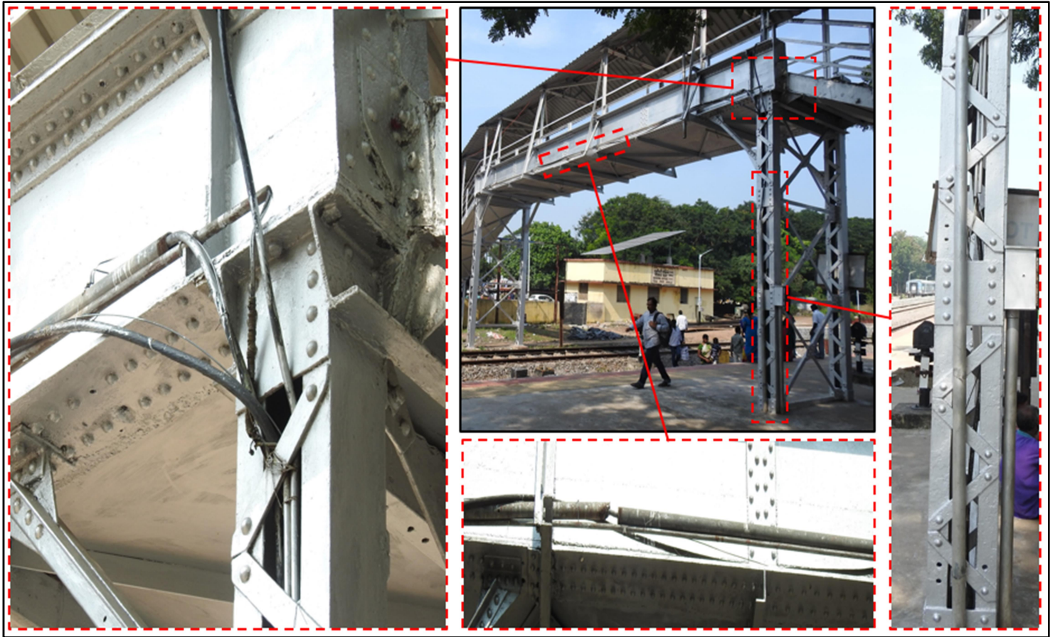
Fig 3: Additional loads of HDPE, GI pipes
