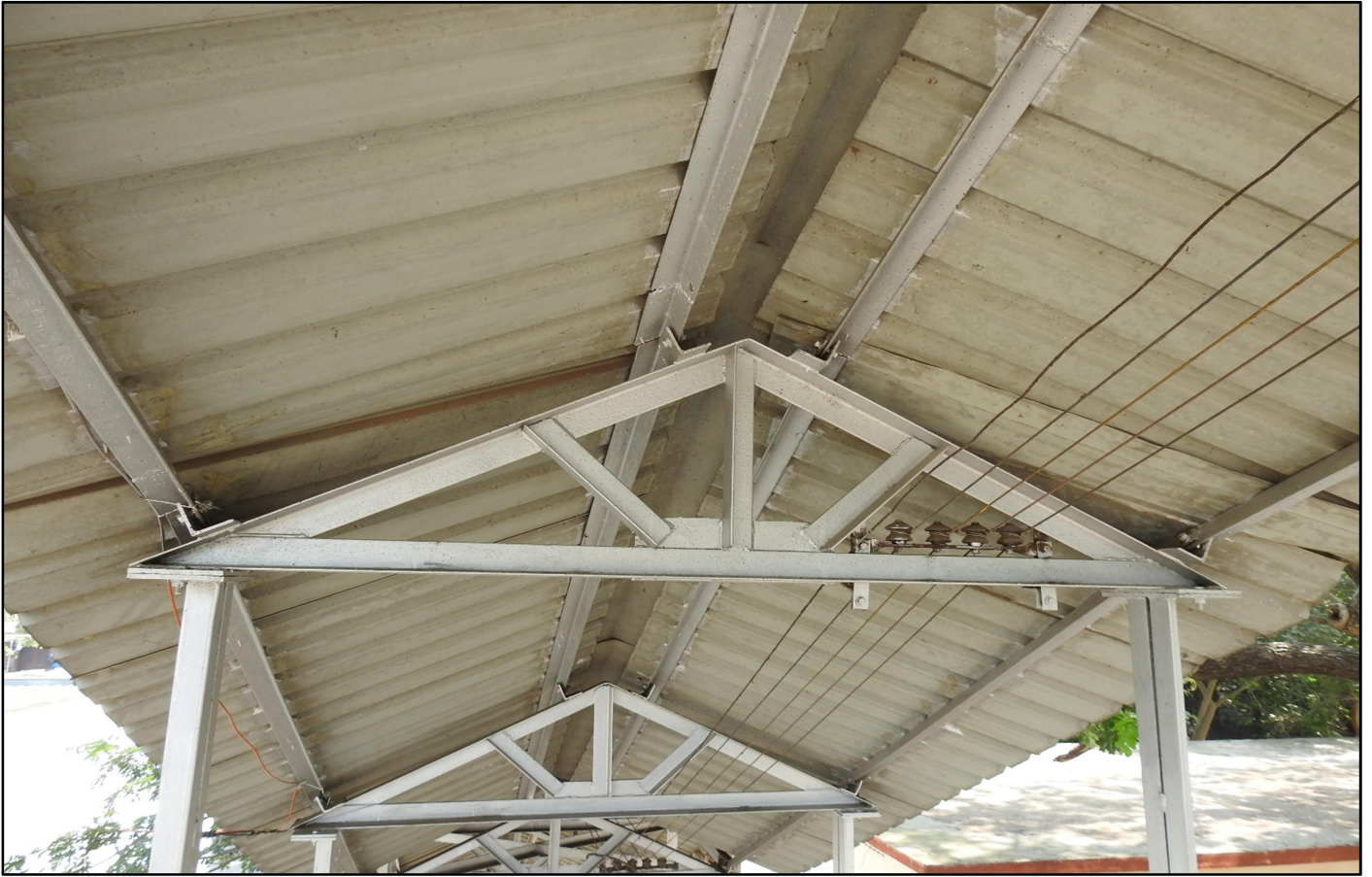
Fig 9: Insulated Electrical lines on Roof truss
