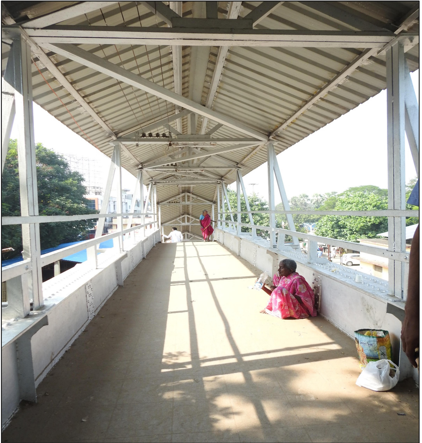
Fig 2: Pathway, Steel Railing of FOB
