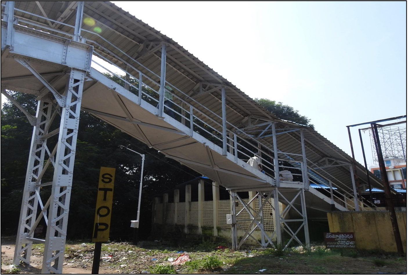
Fig 8: Staircase Bottom view
