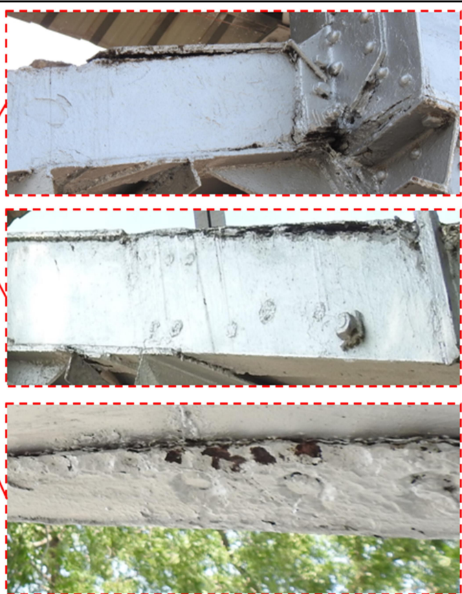
a) Corrosion observed at Staircase 1 Stringer beam
