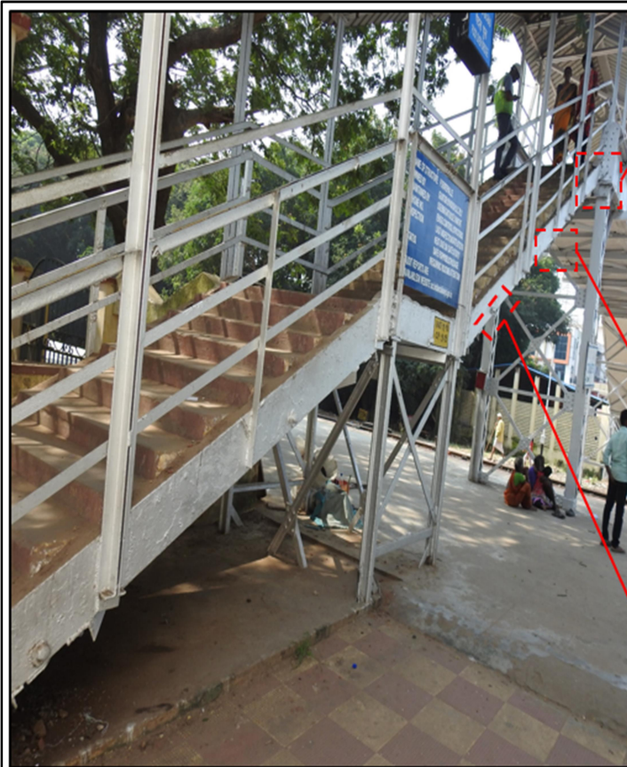
a) Corrosion observed at Staircase 1 Stringer beam
