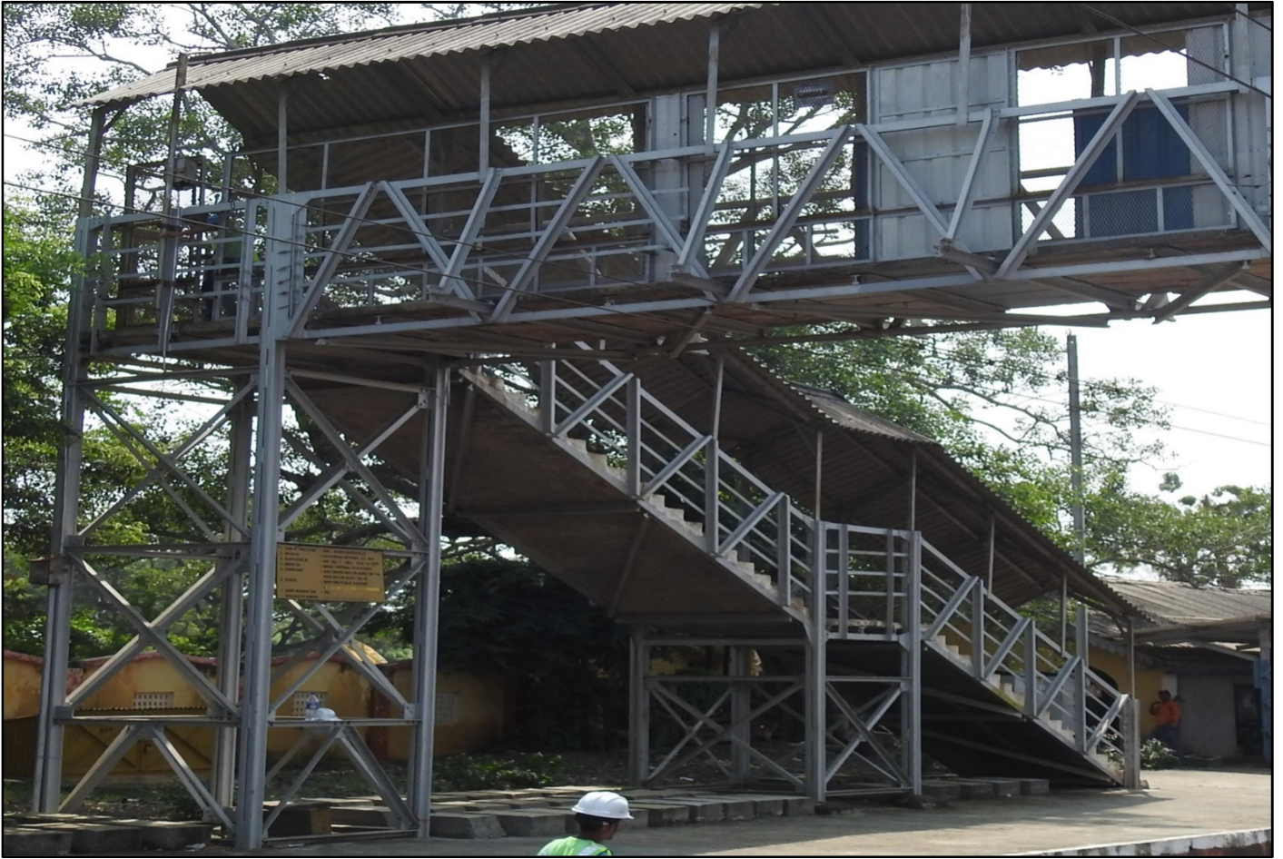
Fig 5: Staircase bottom view
