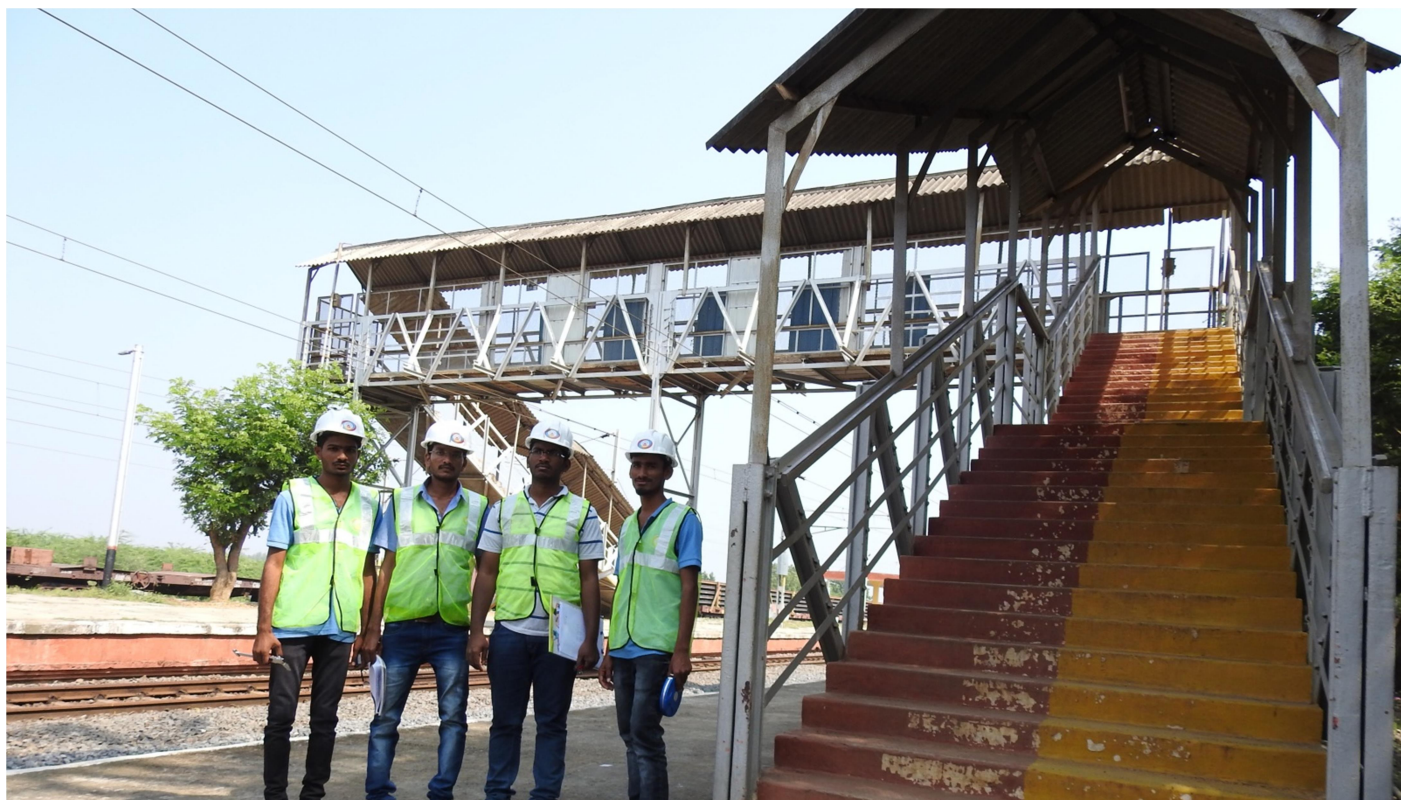
Fig 11: Inspection Team at Ammanabrolu FOB
