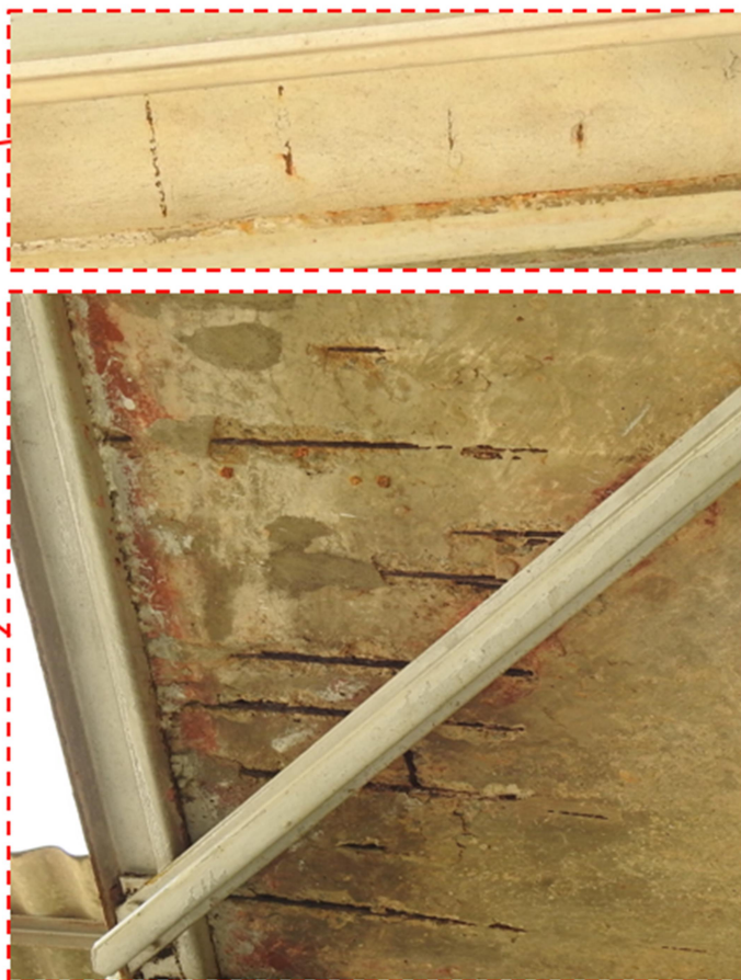
a) Reinforcement exposed observed at Staircase 1 Slab
