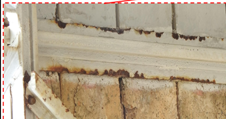
c) Corrosion observed at floor beams on Span 1
