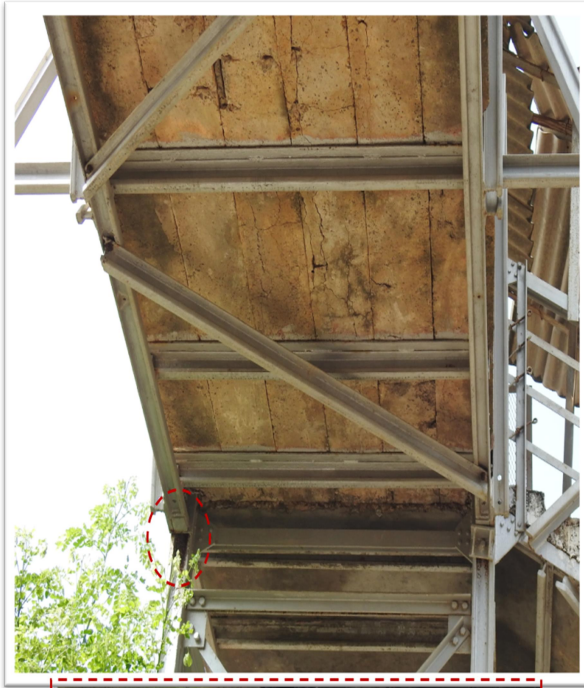
d) Rusting & Corrosion observed at Top & Bottom chord members of FOB
