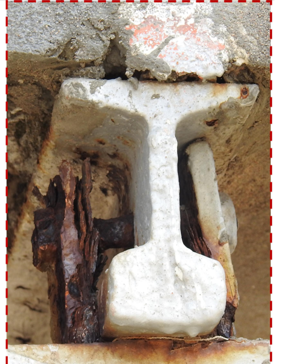
Fig 10: Corrosion of Floor beams joints at Midlandings of Staircase 1 and 2
