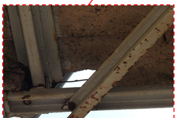
c) Corrosion observed at floor beams on Span 1
