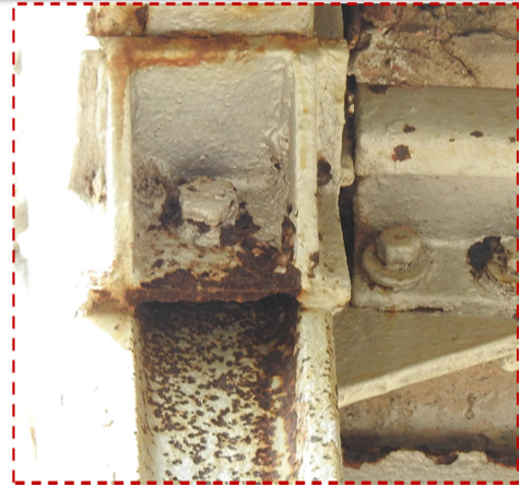
e) Corrosion of Cleat angles at Beam column joint of Trestle-2 and Stanchion
