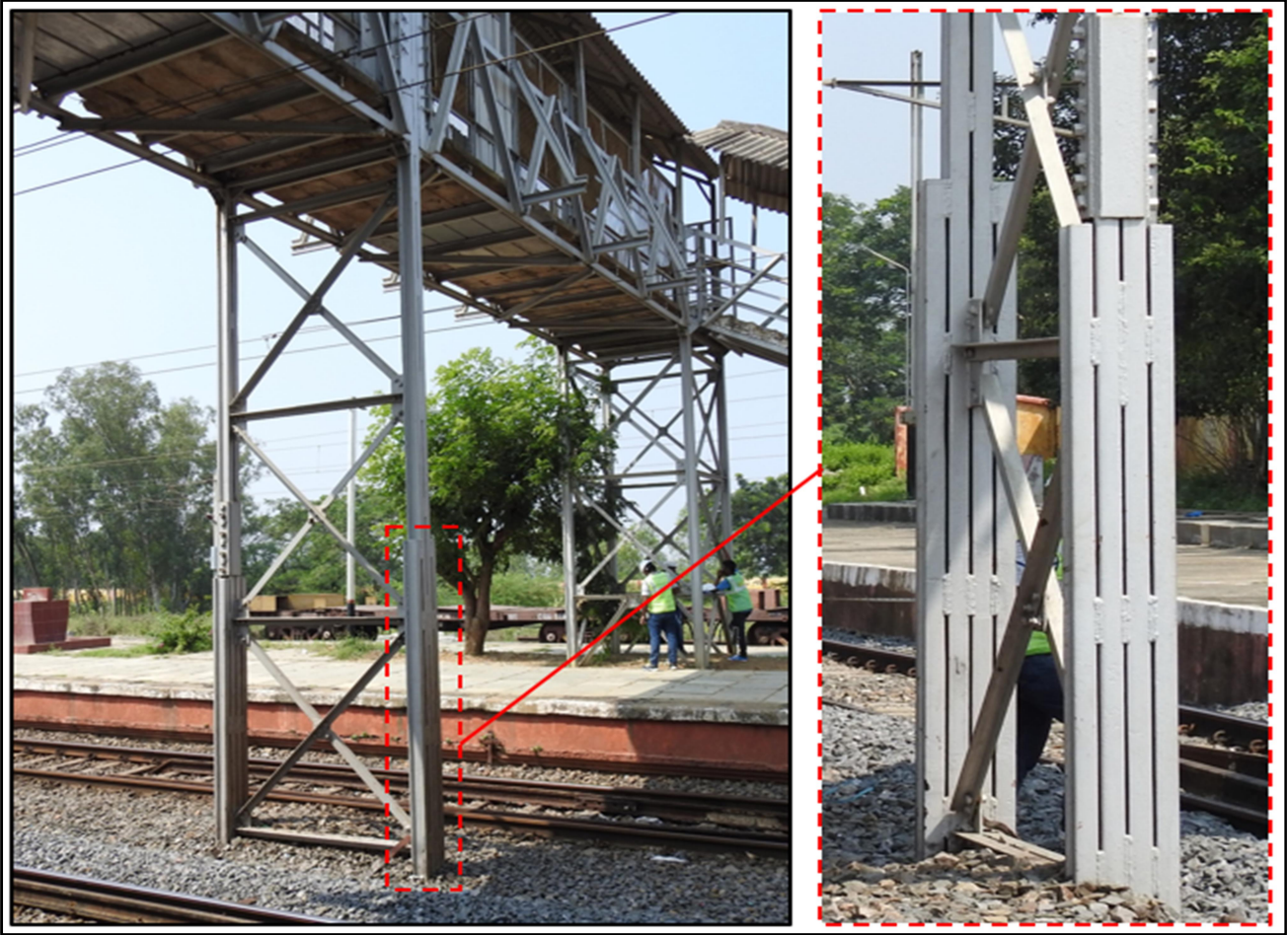
Fig 4: Stanchion column Rail sections details
