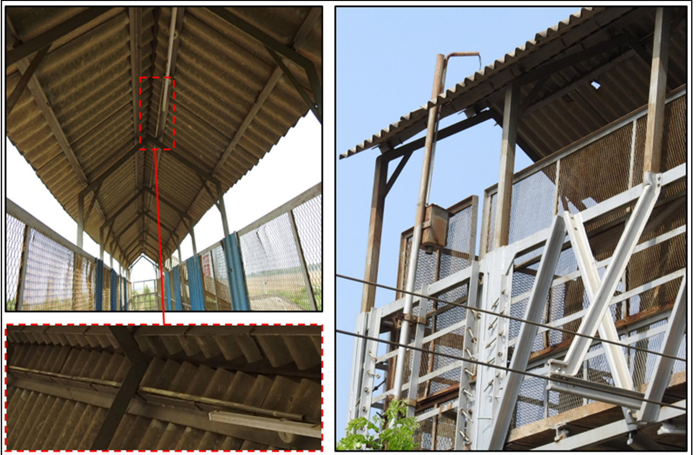
Fig 3: Additional loads of GI, HDPE, PVC pipes
