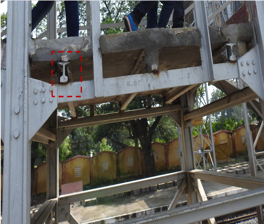
Fig 10: Corrosion of Floor beams joints at Midlandings of Staircase 1 and 2
