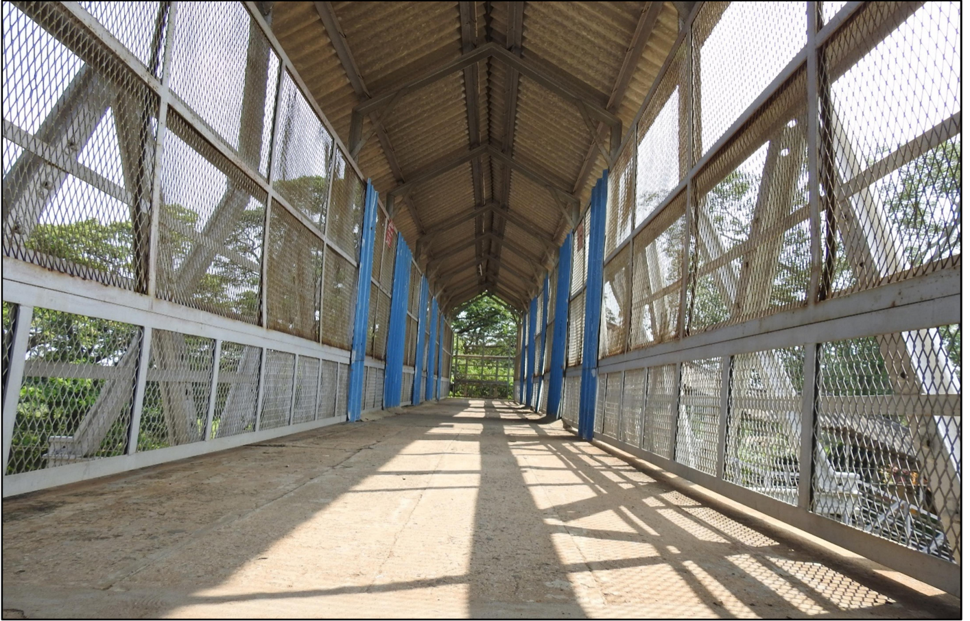
Fig 2: Pathway, protective screen of FOB
