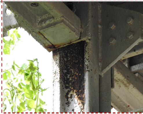
e) Corrosion of Cleat angles at Beam column joint of Trestle-2 and Stanchion
