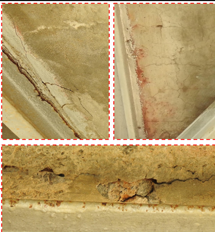
b) Cracks and reinforcement exposed observed at Staircase 2 Slab
