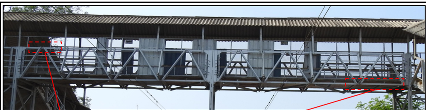
c) Corrosion observed at floor beams on Span 1
