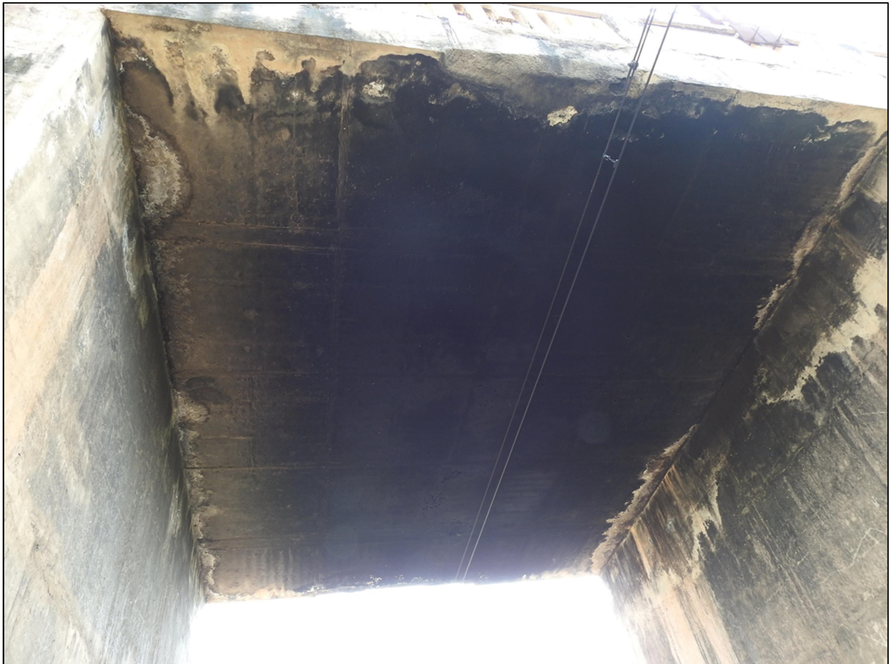
Fig 3: Bottom view of Slab
