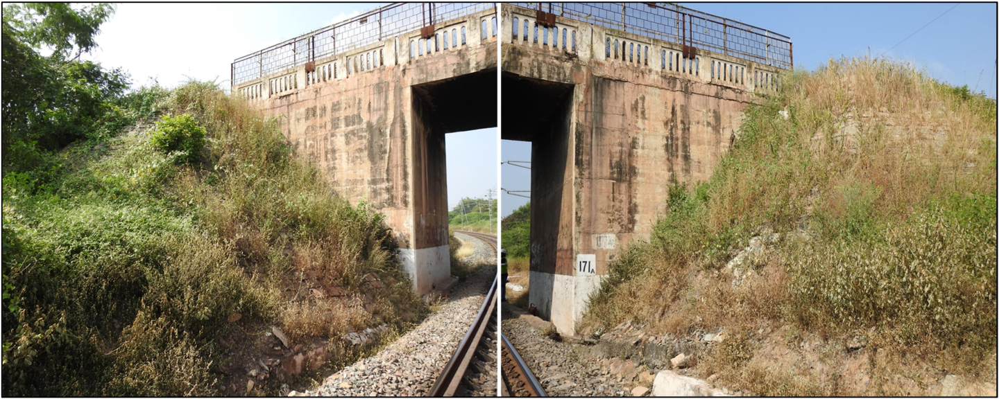
Fig 2: Abutment on both sides (A1 and A2)
