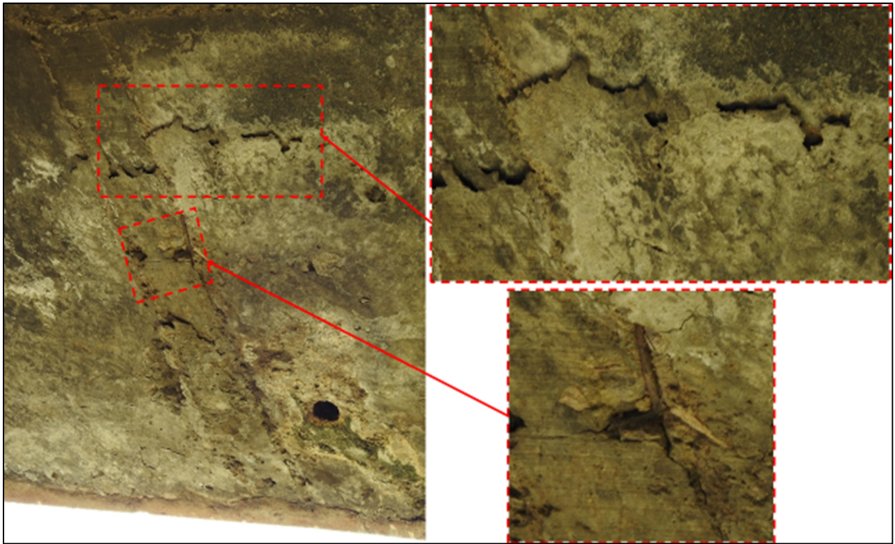
Fig: 16 Spalling & Reinforcement exposure observed at slab of Span-5
