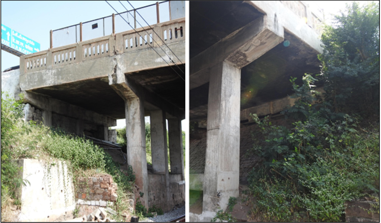
Fig: 2 View of Abutment (A1 and A2)
