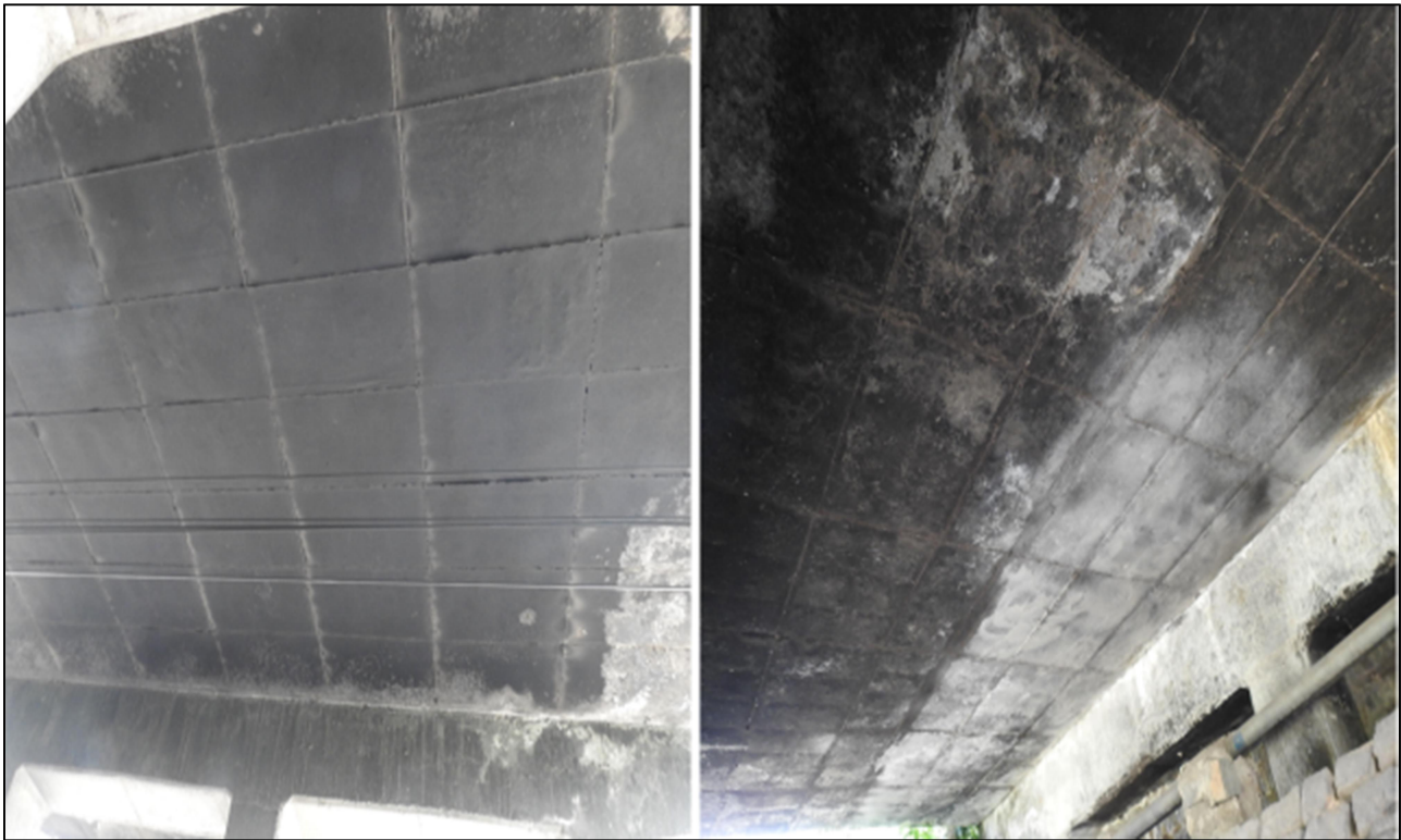
Fig: 3 Bottom view of Slab
