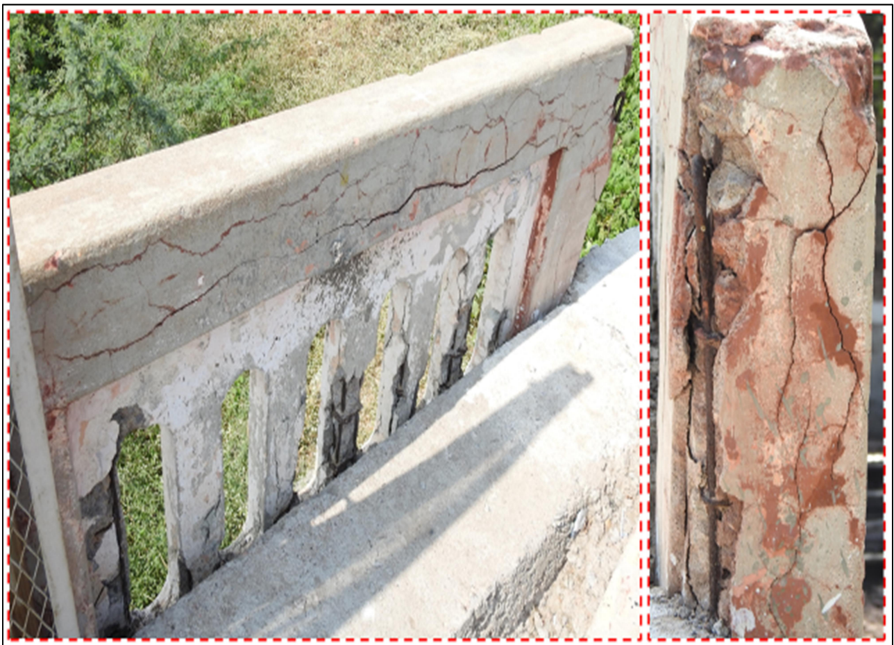
Fig: 16 Spalling & Reinforcement exposure observed at slab of Span-5
