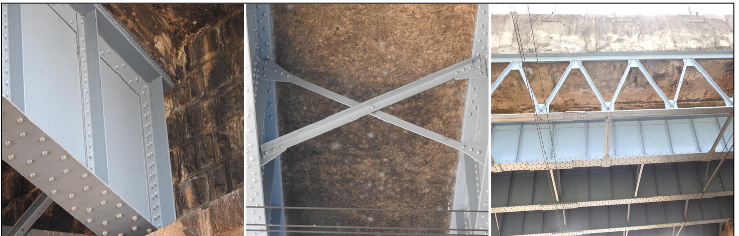
Fig: 4 View of Longitudinal & Cross Girders
