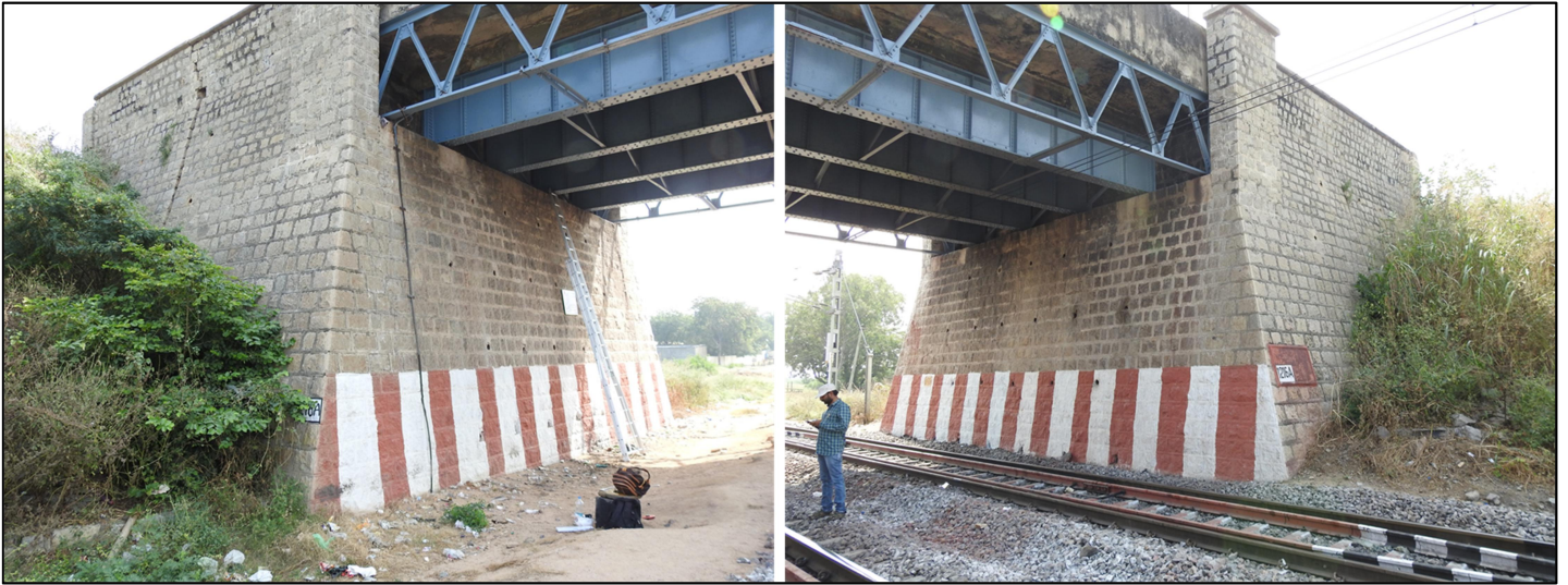
Fig: 2 Abutment (A1 and A2) Stone Masonry
