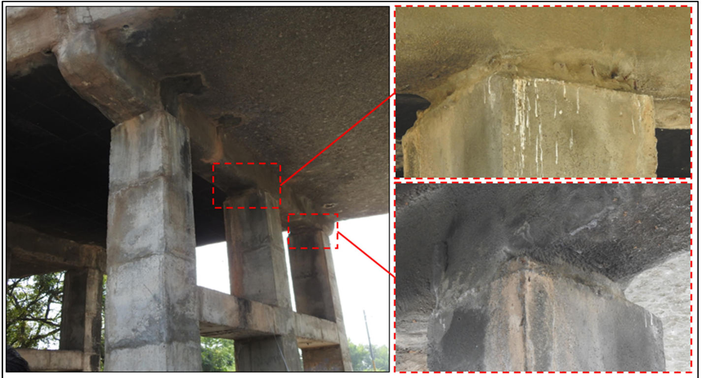
Fig.3: Patch works observed at Columns
