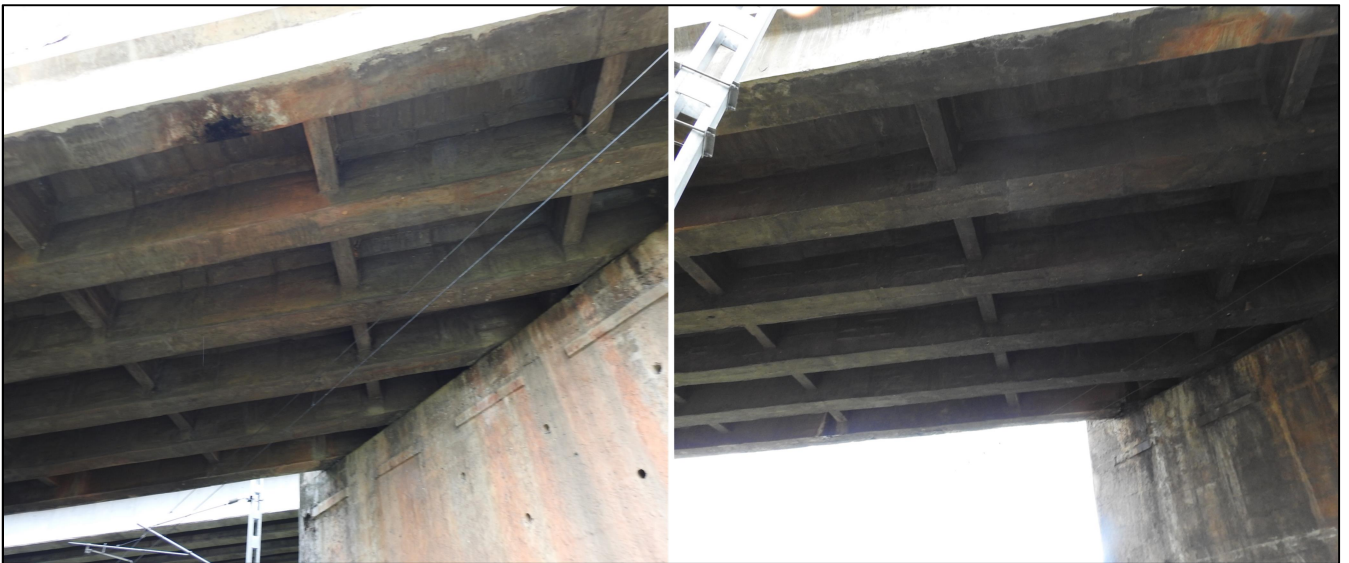
Fig: 3 Bottom view of Bridge
