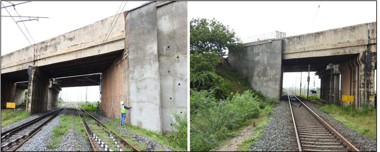
Fig: 2 View of Abutments (A1 and A2)
