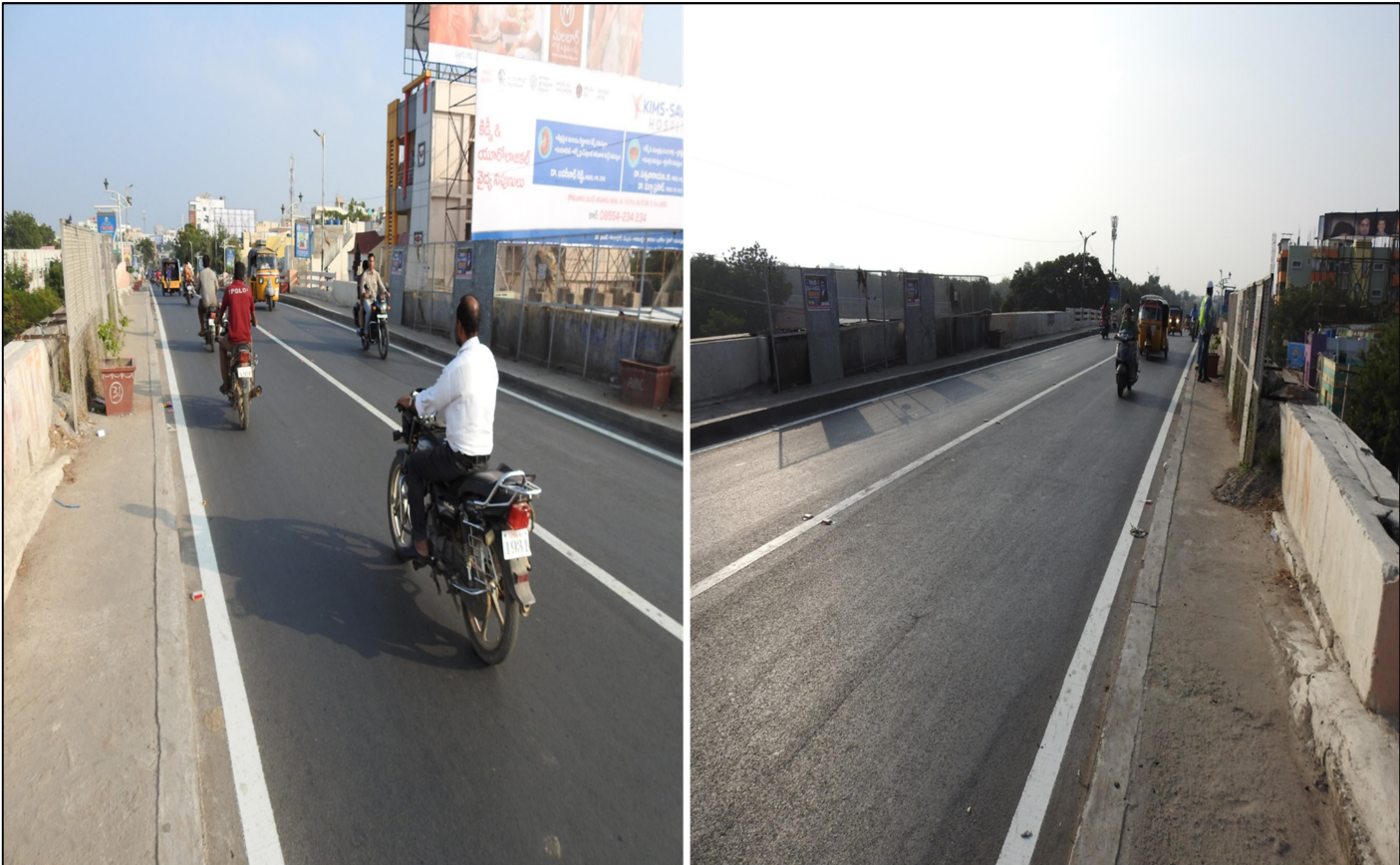
Fig 7: Top View / Wearing coat of the Bridge
