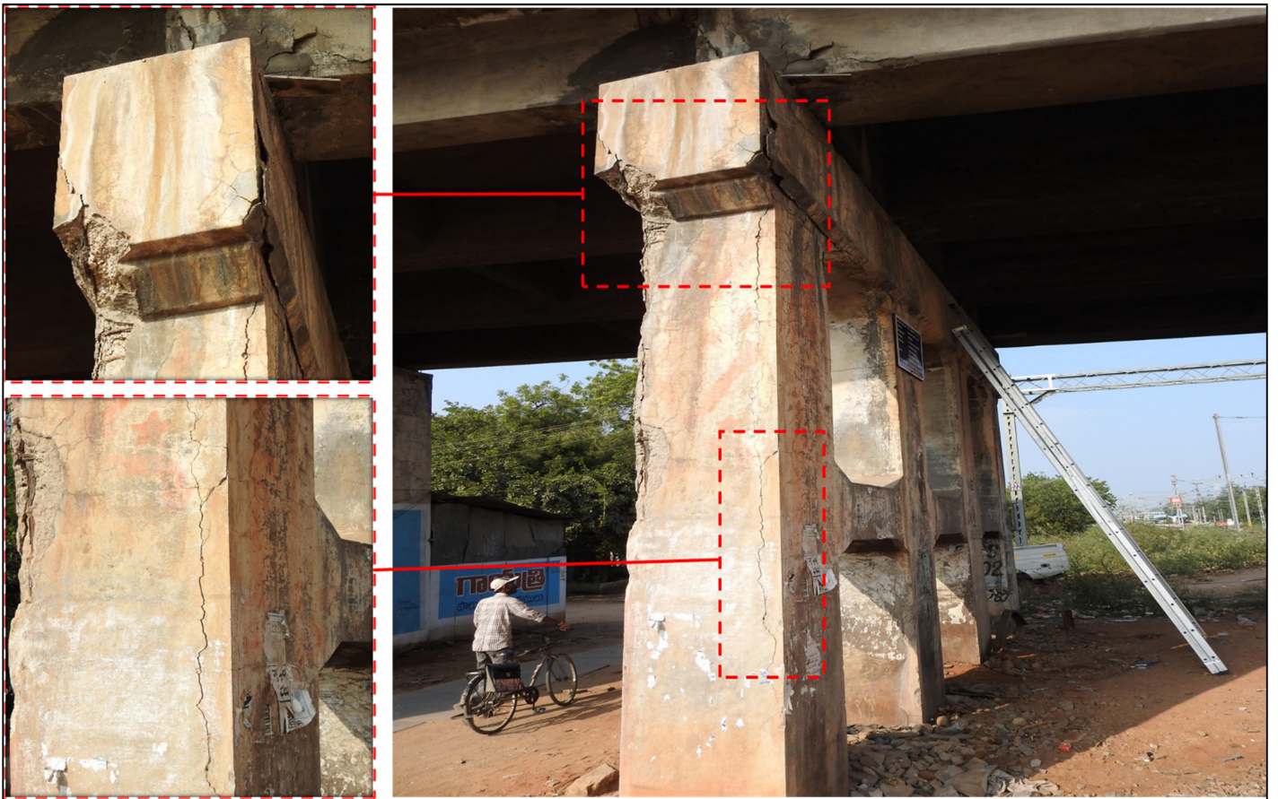
Fig 5(b): Cracks, Spalling & Patching works in column and cap of Pier
