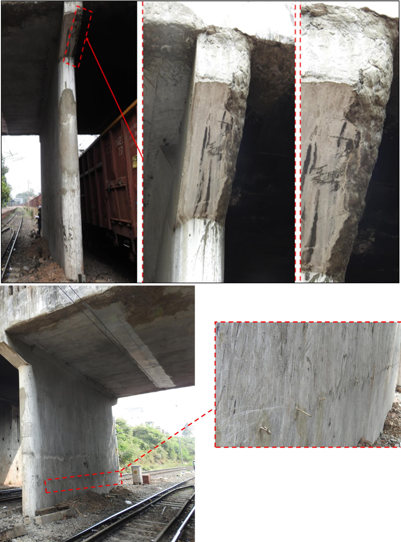
Fig: 6 Grouting observed at Pier
