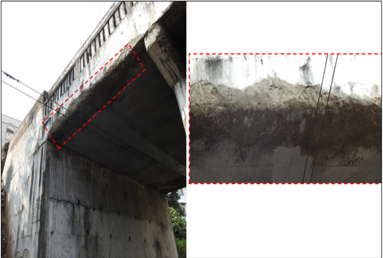
Fig: 9 Patch repair work observed at Span-2
