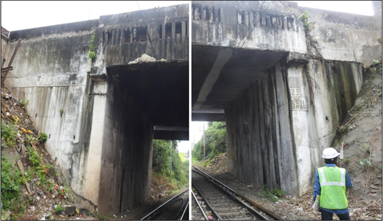
Fig: 2 Abutments (A1 and A2)
