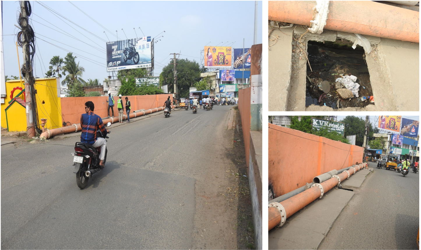
Fig 15: Road surface and drain on ROB
