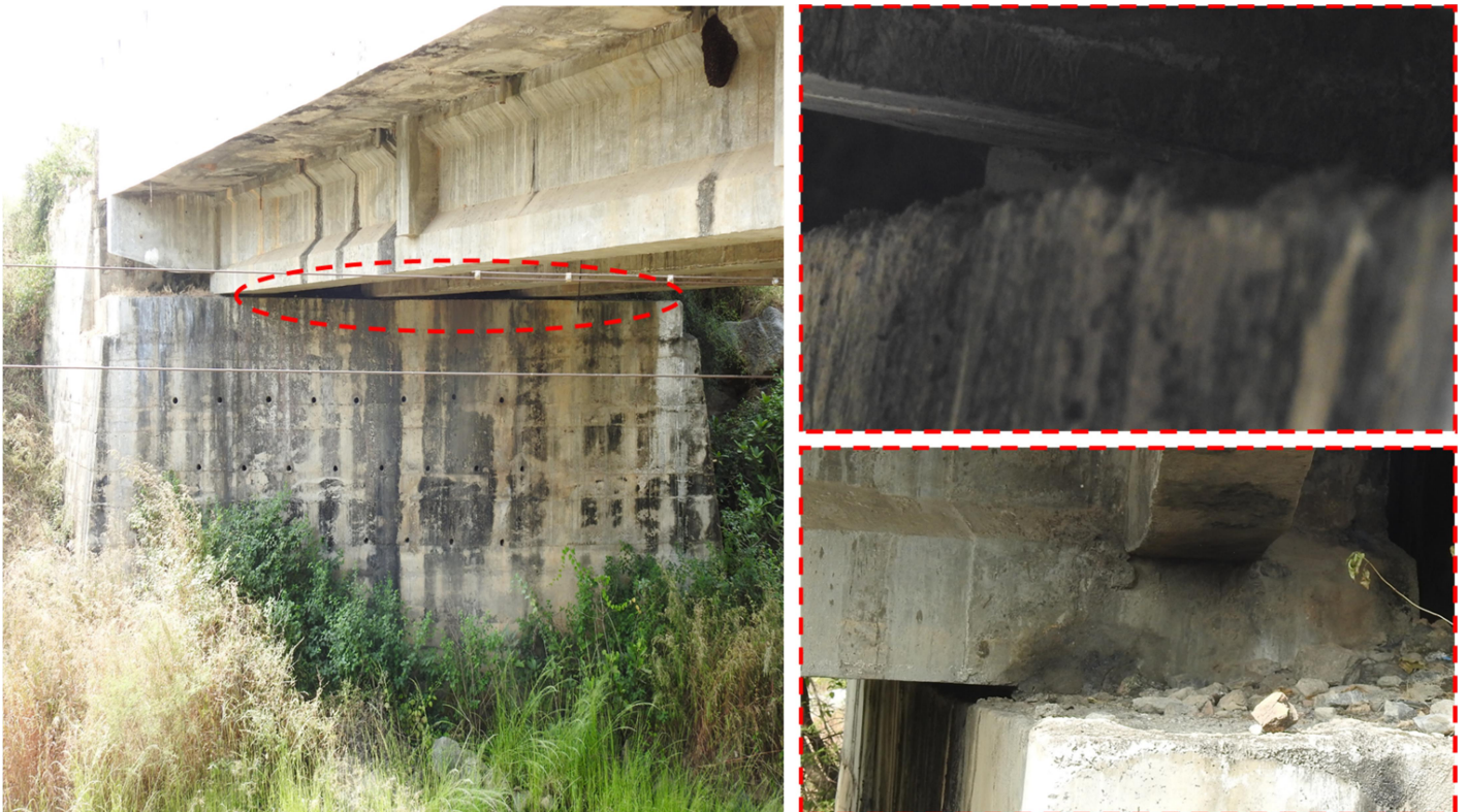
Fig 8: Bearing details
