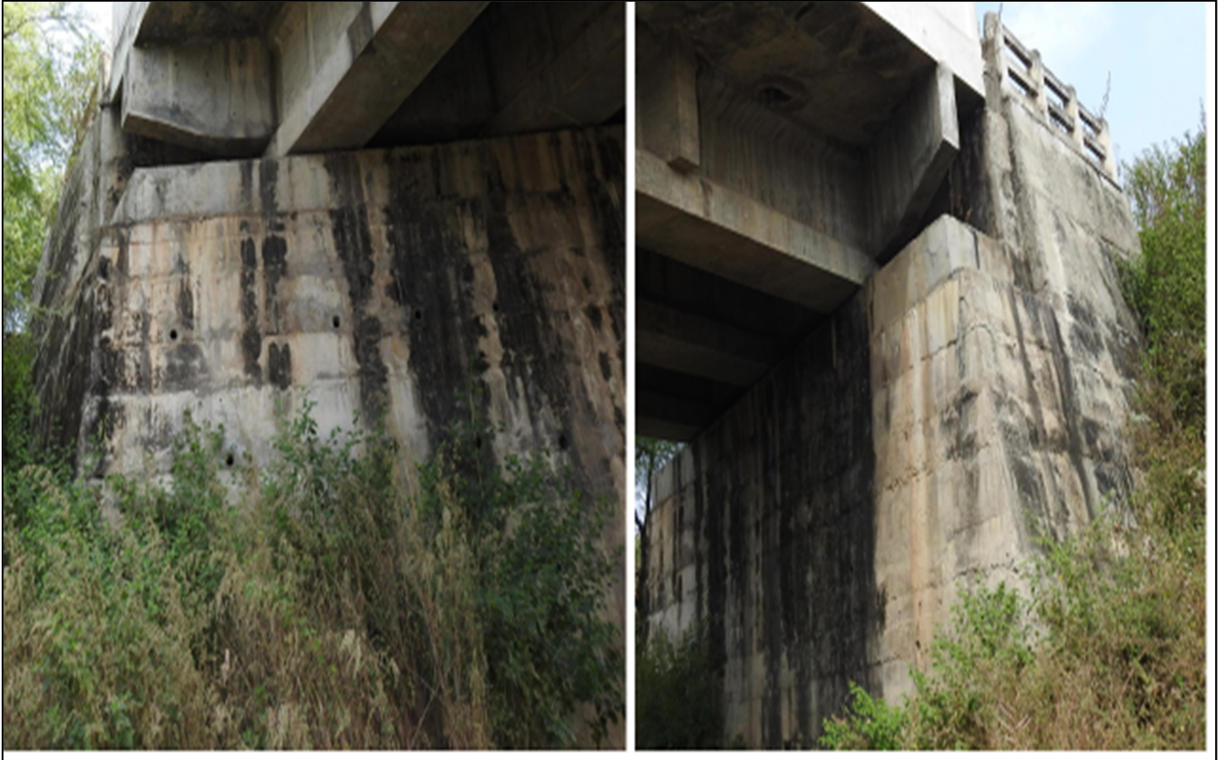
Fig: 2 View of Abutments (A1 and A2)
