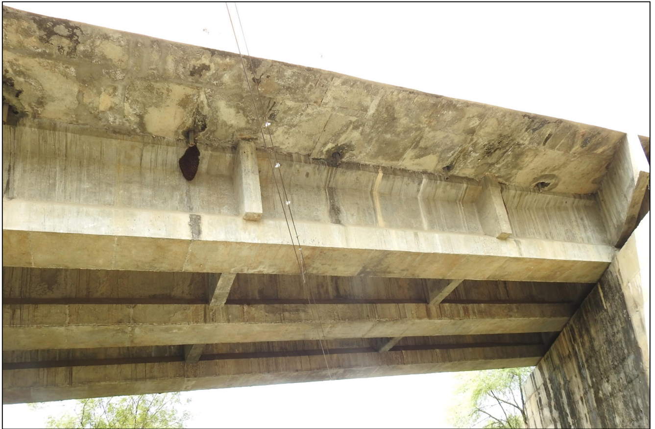
Fig: 3 Bottom view of Bridge
