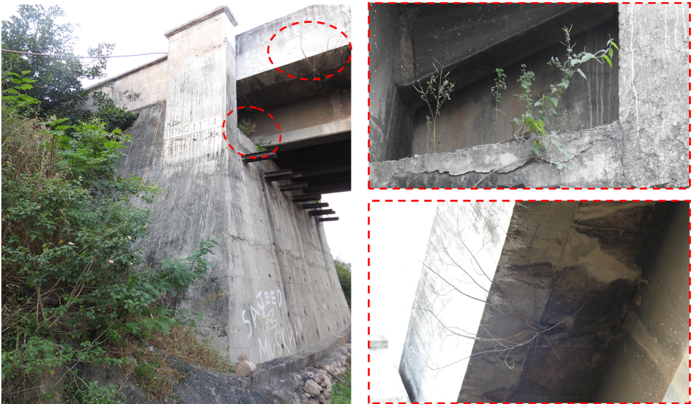
Fig 12: Vegetation observed at abutment and Drainage spouts
