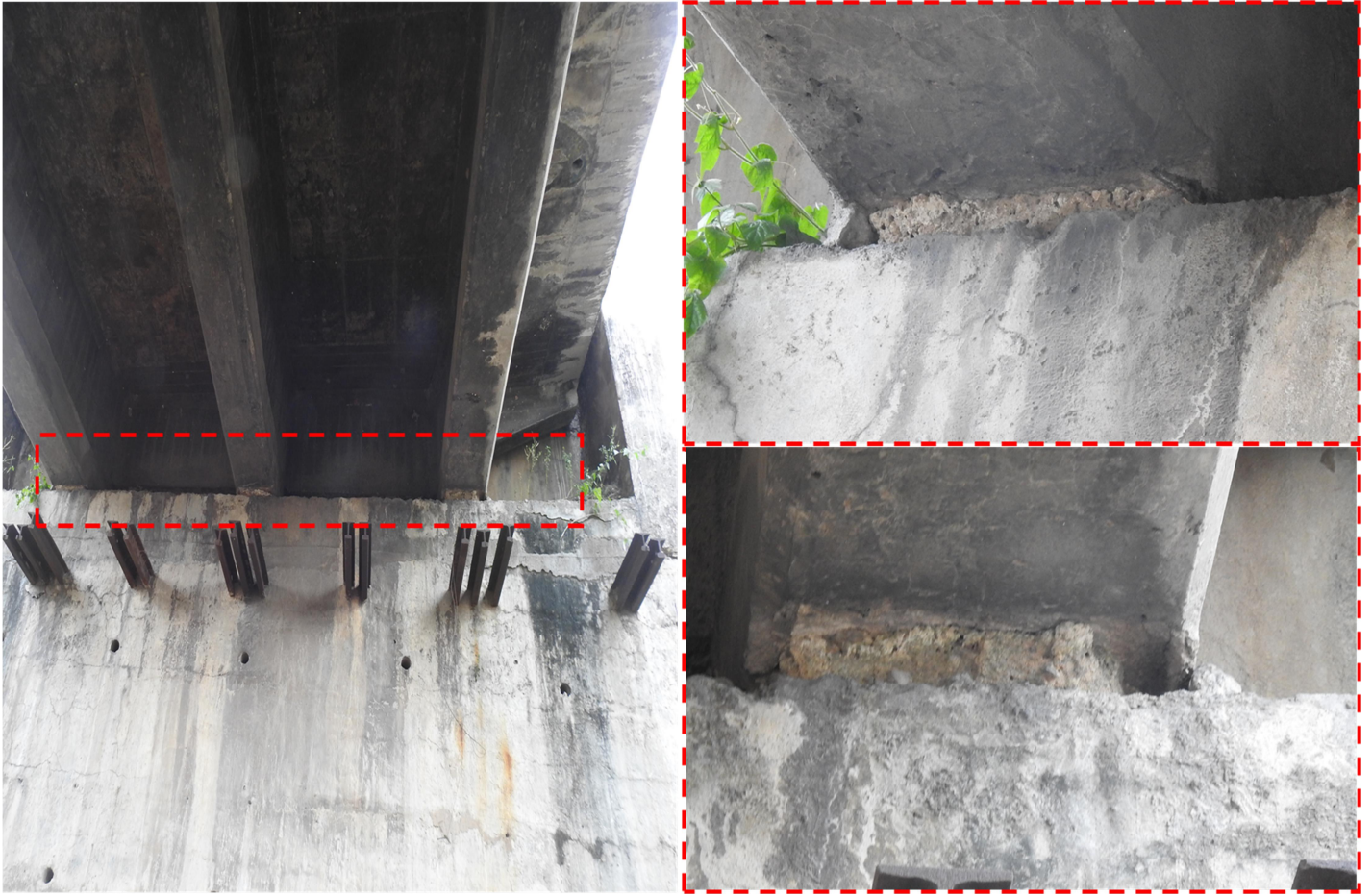
Fig 4: Bearings at Abutment 1
