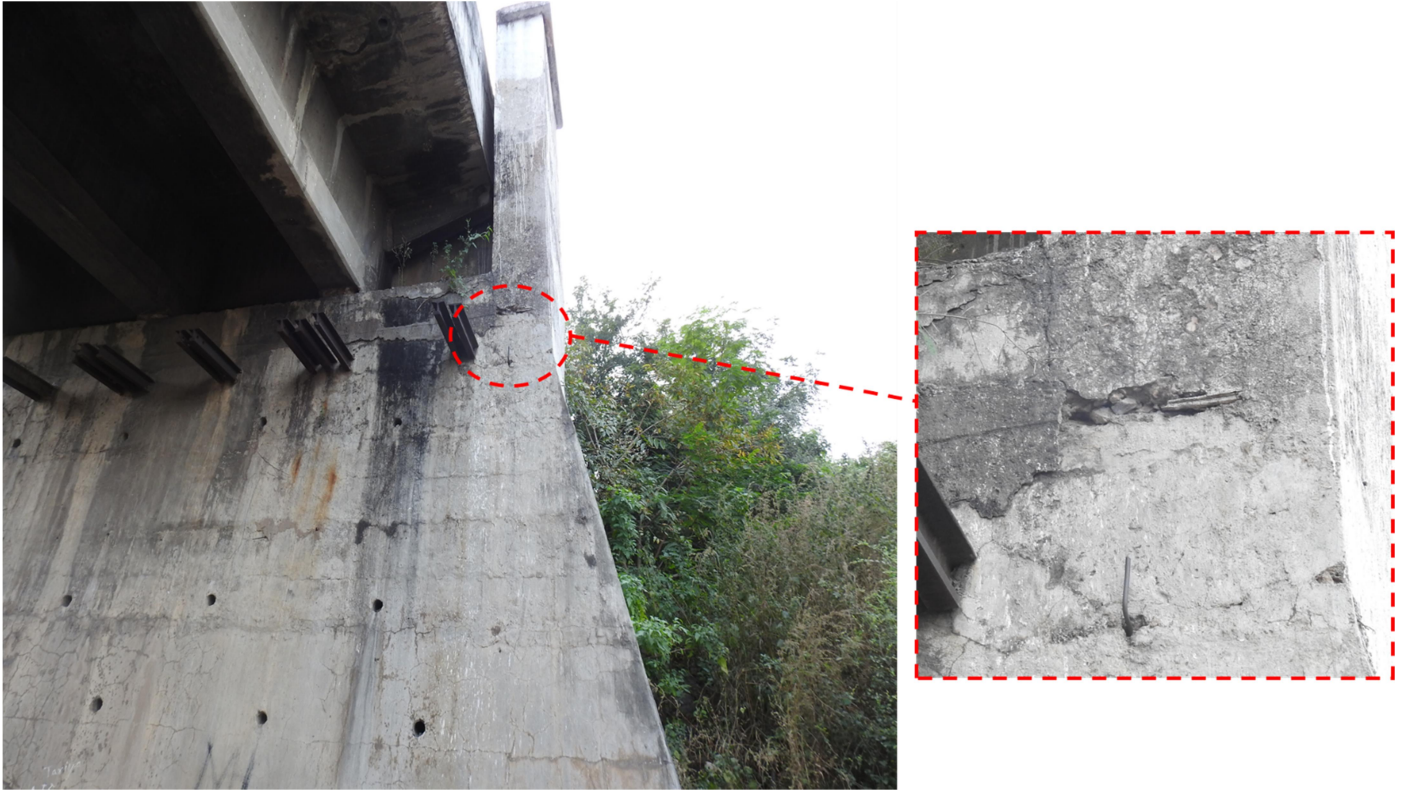
Fig 7: Minor Spalling, leaching at Abutment
