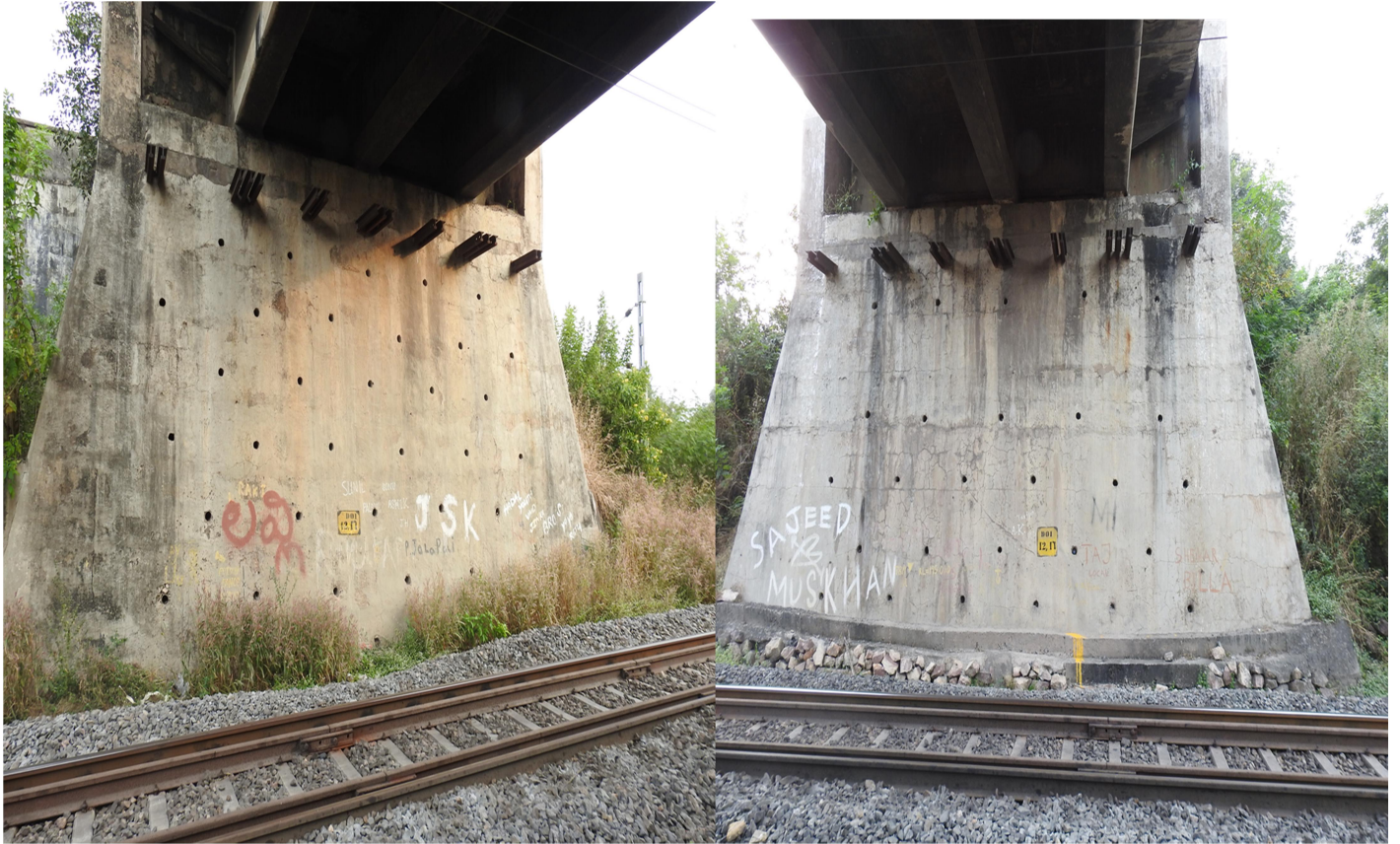
Fig: 2 Abutments (A1 and A2)
