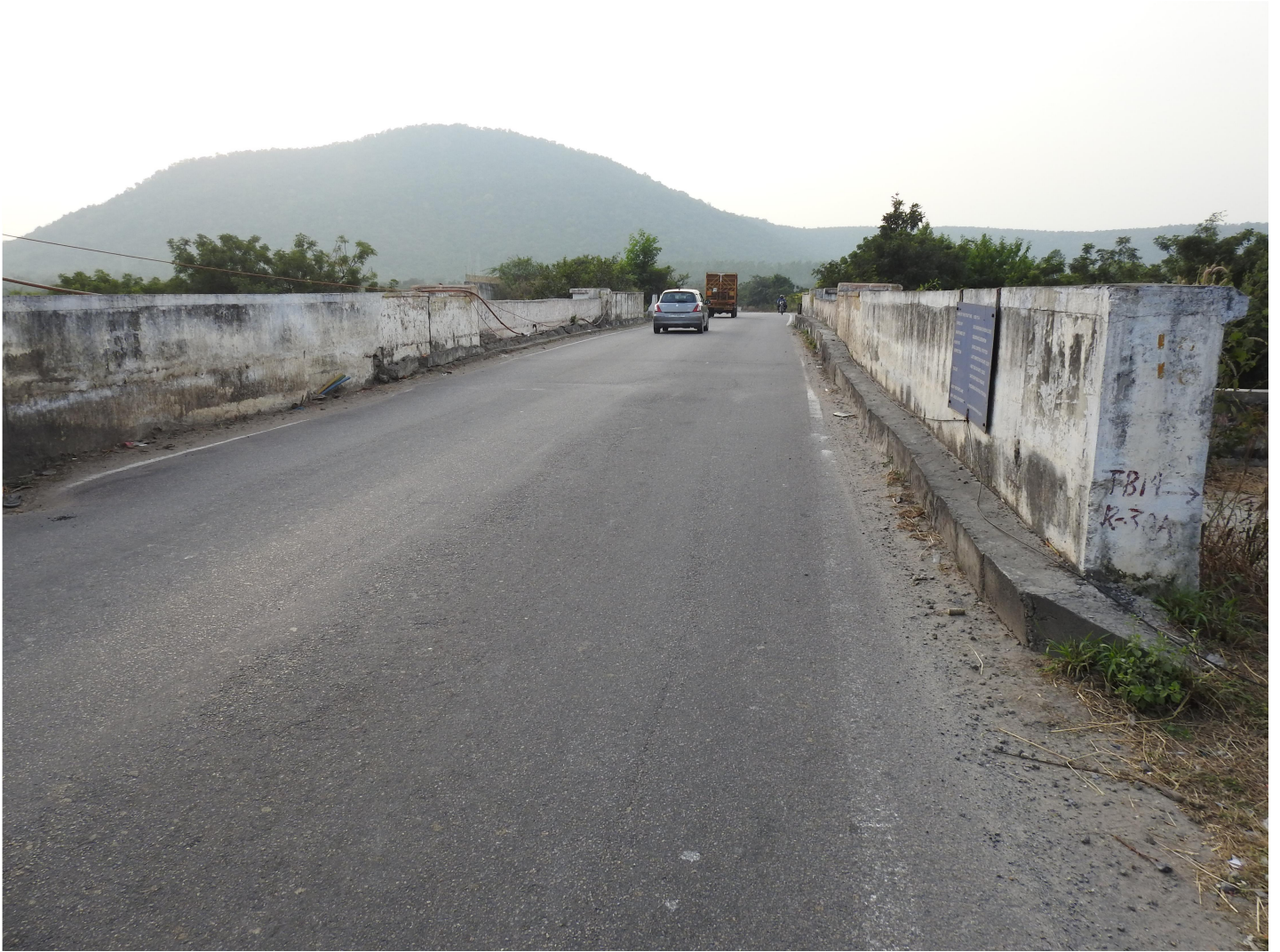
Fig 13: Road surface & Parapet wall
