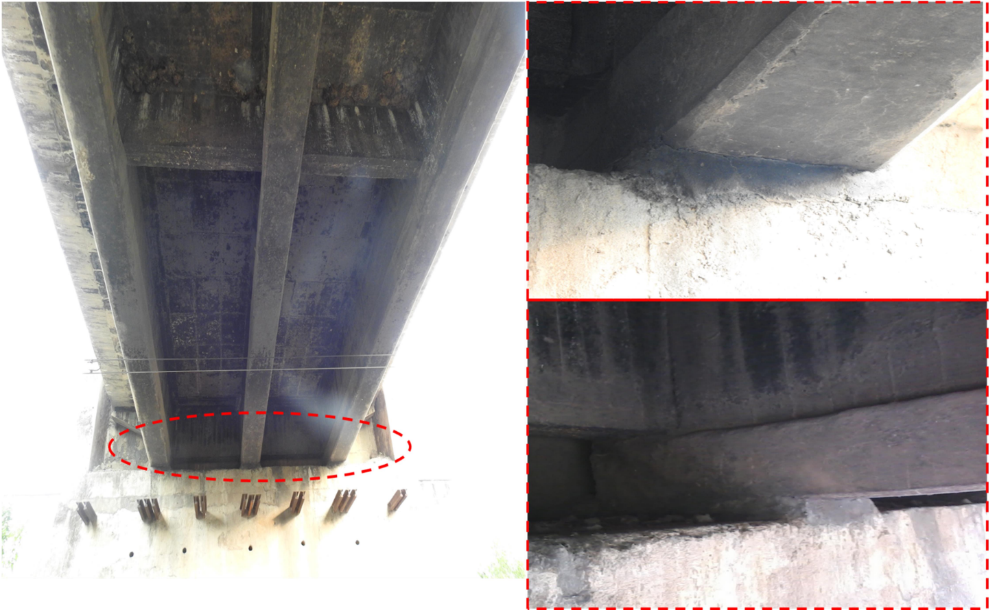
Fig 5: Bearings at Abutment 2
