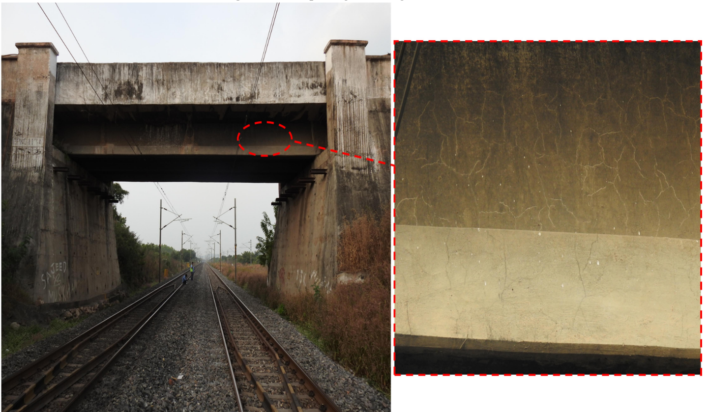
Fig 7: Minor Spalling, leaching at Abutment
