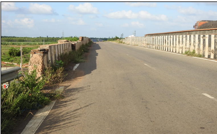
Fig 18: Vegetation at Pier cap & Abutment Retaining Walls
