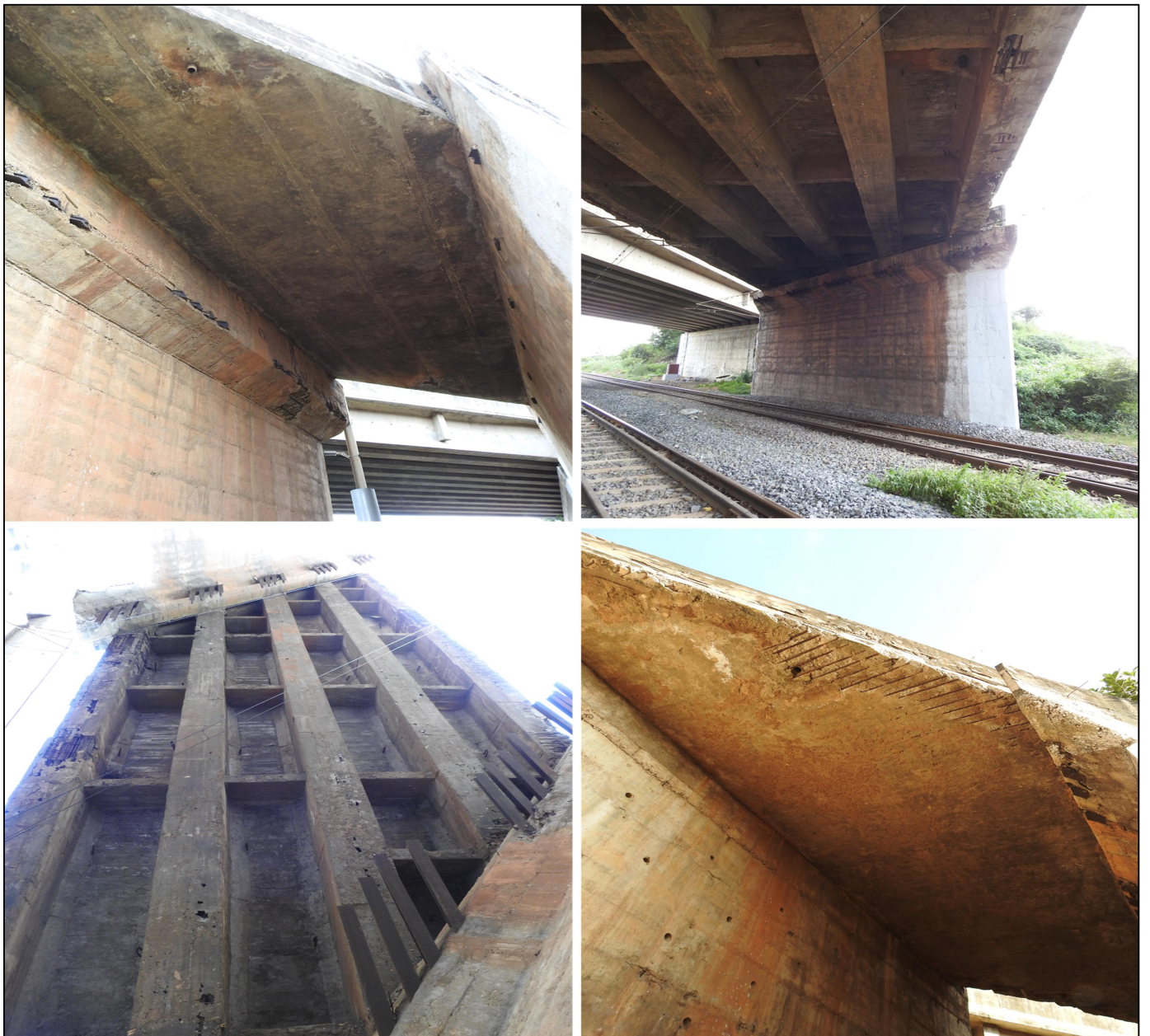
Fig: 3 Bottom view of the Bridge
