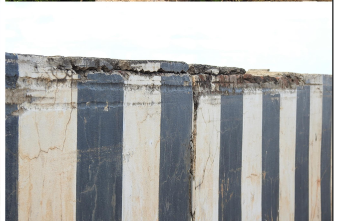
Fig 19: Top View/ Condition of Road surface and Crash Barrier
