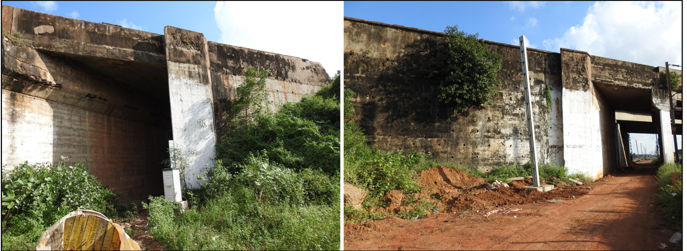
Fig: 2 Abutments (A1 and A2)
