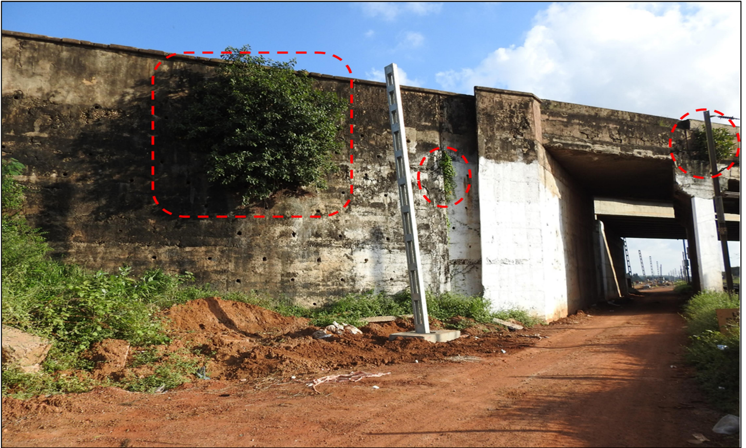
Fig 18: Vegetation at Pier cap & Abutment Retaining Walls
