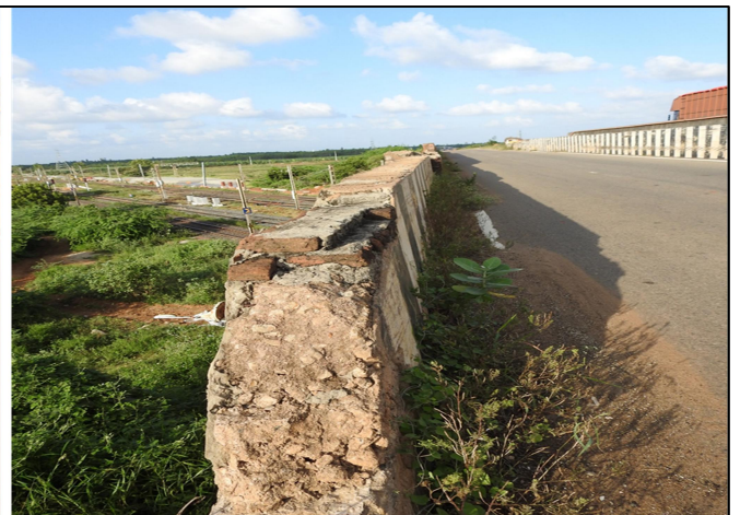
Fig 18: Vegetation at Pier cap & Abutment Retaining Walls
