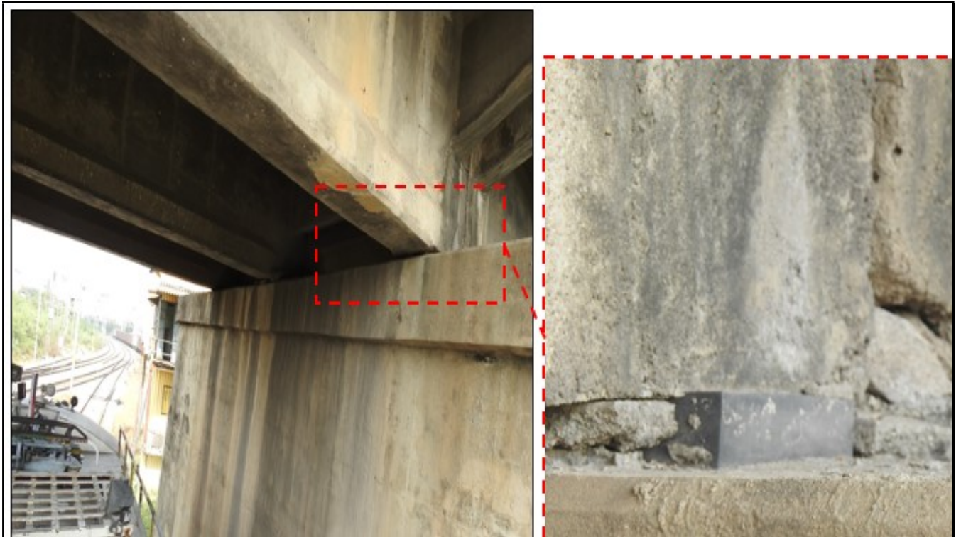
Fig.4 : Elastomeric Bearings observed at span 2 & 3
