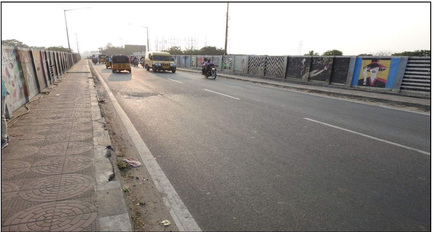
Fig.16 : Road surface, Parapet wall
