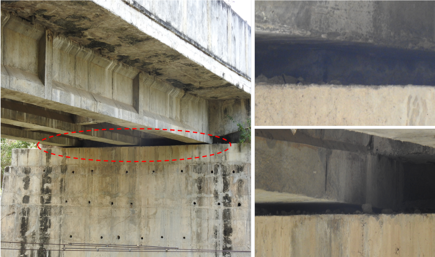
Fig 8: Bearing details
