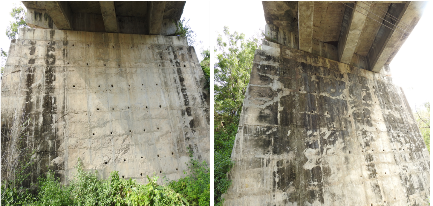
Fig: 2 Abutments (A1 and A2)
