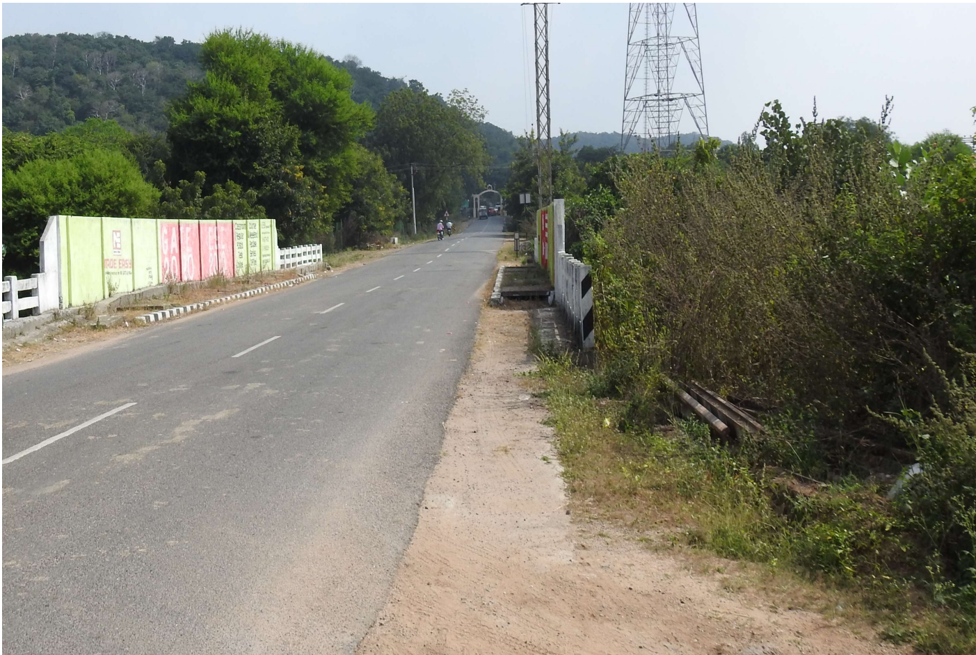
Fig 10: Road surface & Parapet wall
