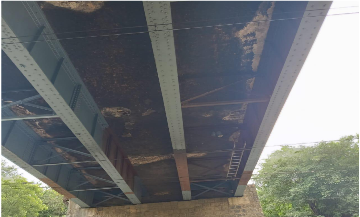
Fig:2 Bottom view of Slab
