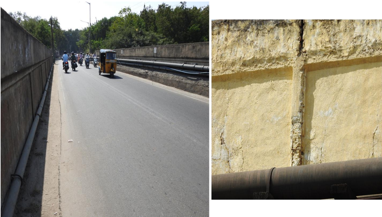
Fig: 13 Wearing coat and parapet wall
