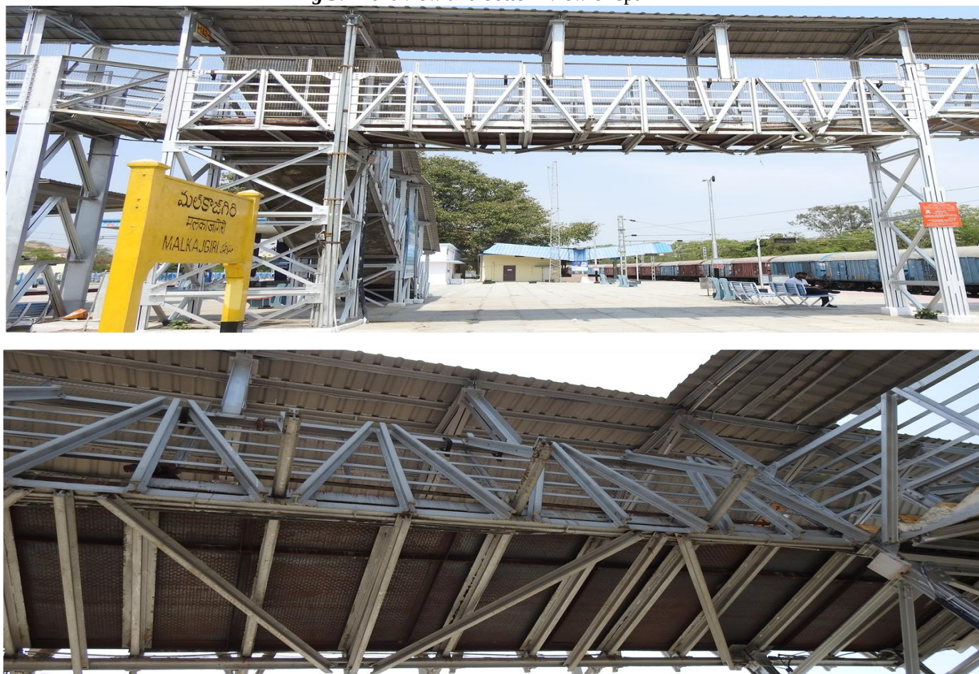
Fig 4: Front view and bottom view of span 2
