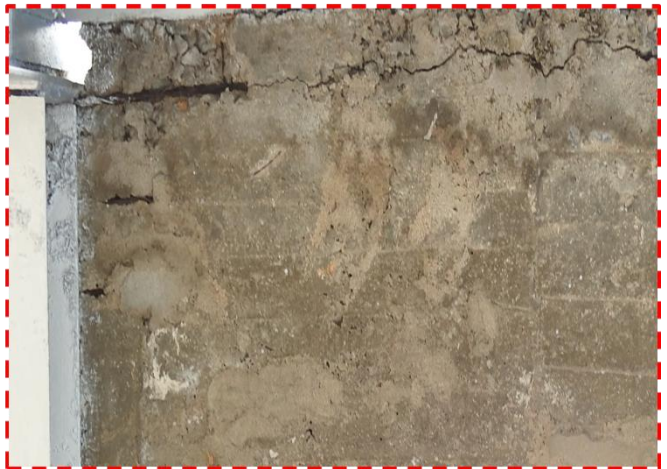
Spalling and reinforcement exposure in span 1
