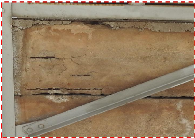
Spalling and reinforcement exposure in span 1
