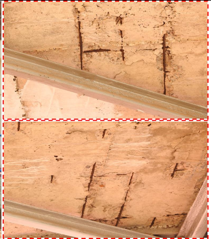
Spalling at stair case 3
