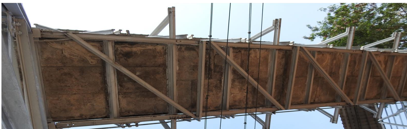
Fig 6: Front view and bottom view of span 4
