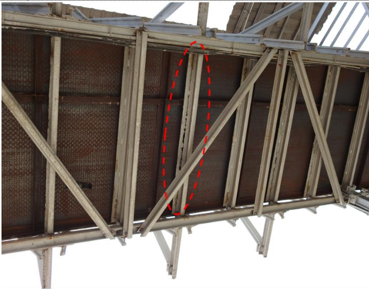
Slight Corrosion of Floor beams
