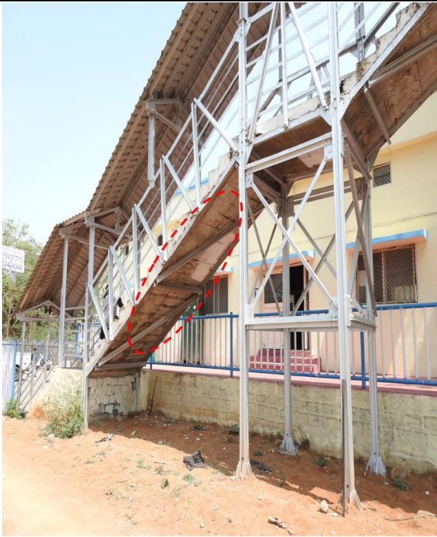
Spalling at stair case 3
