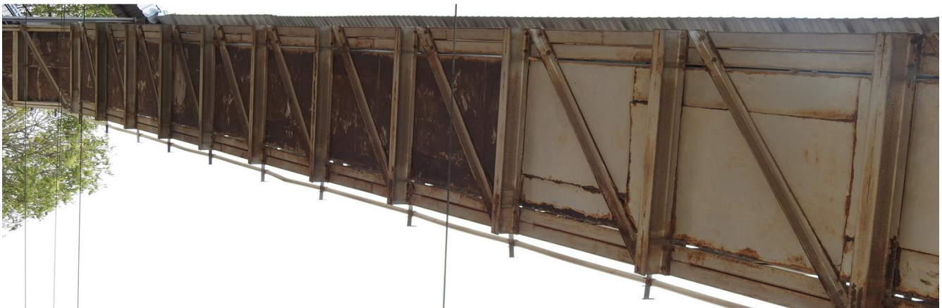
Fig 4: Front view and bottom view of span 2
