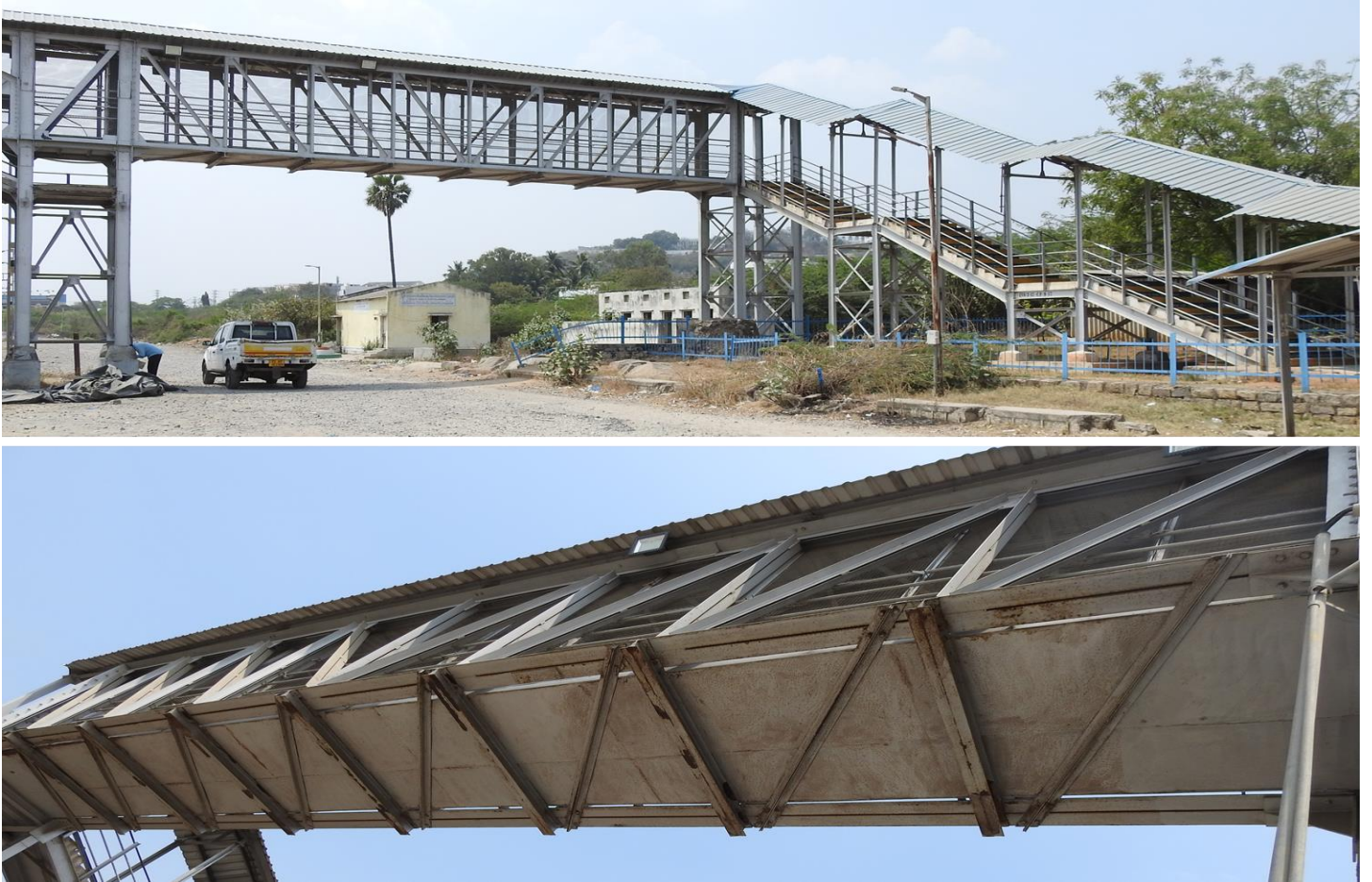
Fig 5: Front view and bottom view of span 3
