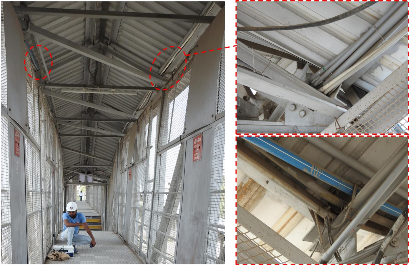
Fig 1: Cables, Roof truss, Flooring and Protective screen
